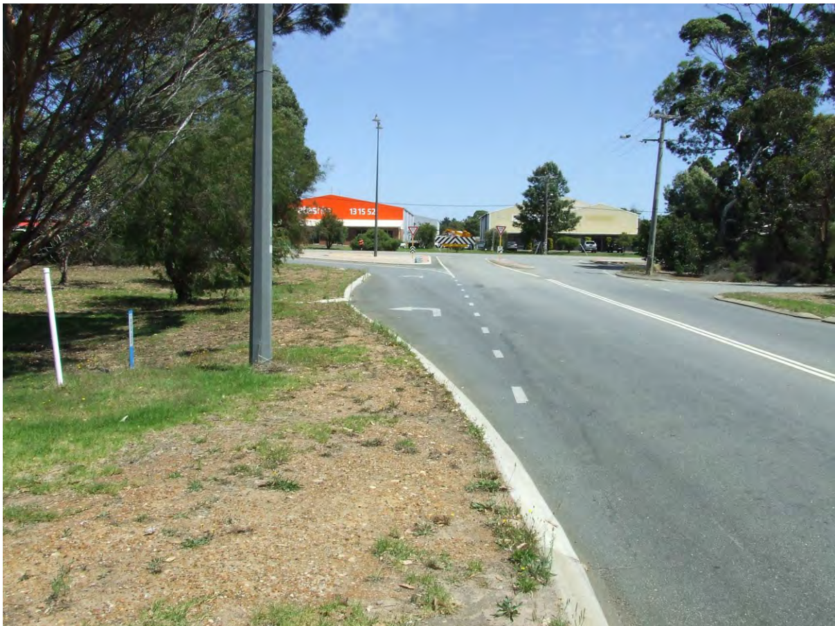
FIGURE 2 – LEFT TURN AUXILIARY LANE ON MERCER ROAD CONSTRUCTED 2012/13
