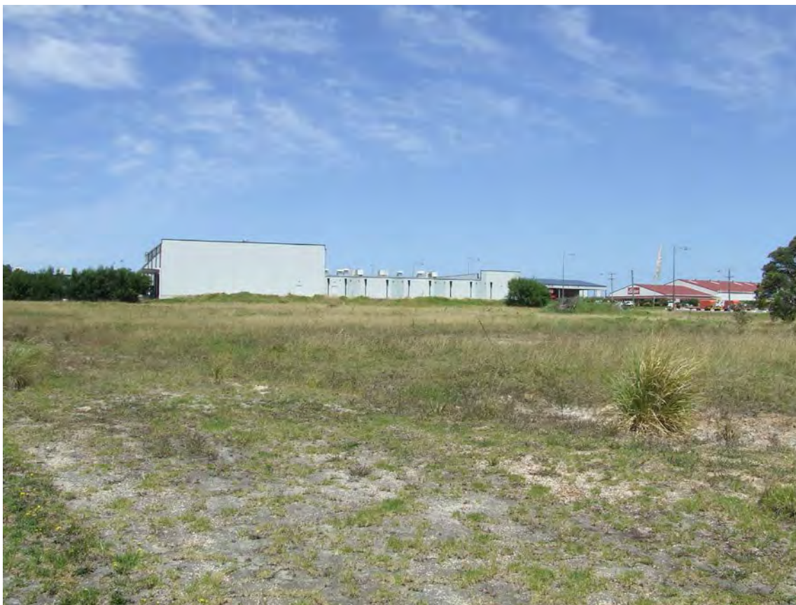
FIGURE 7 – LOT 1004 VIASTRA DRIVE, VIEW FROM VIASTRA DRIVE
