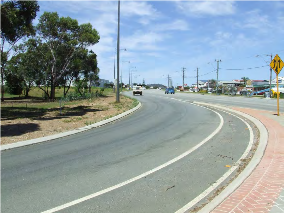
FIGURE 3 – MERGE LANE FROM MERCER ROAD ONTO CHESTER PASS ROAD, CONSTRUCTED 2012/13
