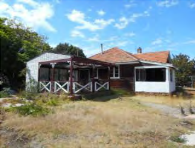
Photograph 1 – View of existing dwelling central to the property.
