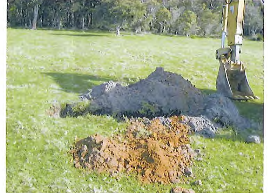
Typical soils of much of the site, with grey and white sand over laterite over yellow silt
