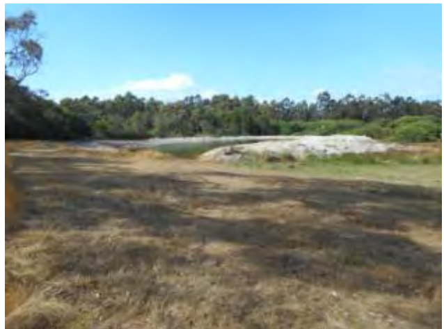
Photograph 6 – View of dam located in the southern portion of the property.
