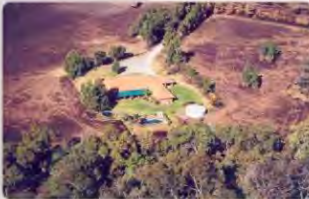
Above: Reduced fuel in the Building Protection Zone contributed to the survival of this home in a bushfire.
