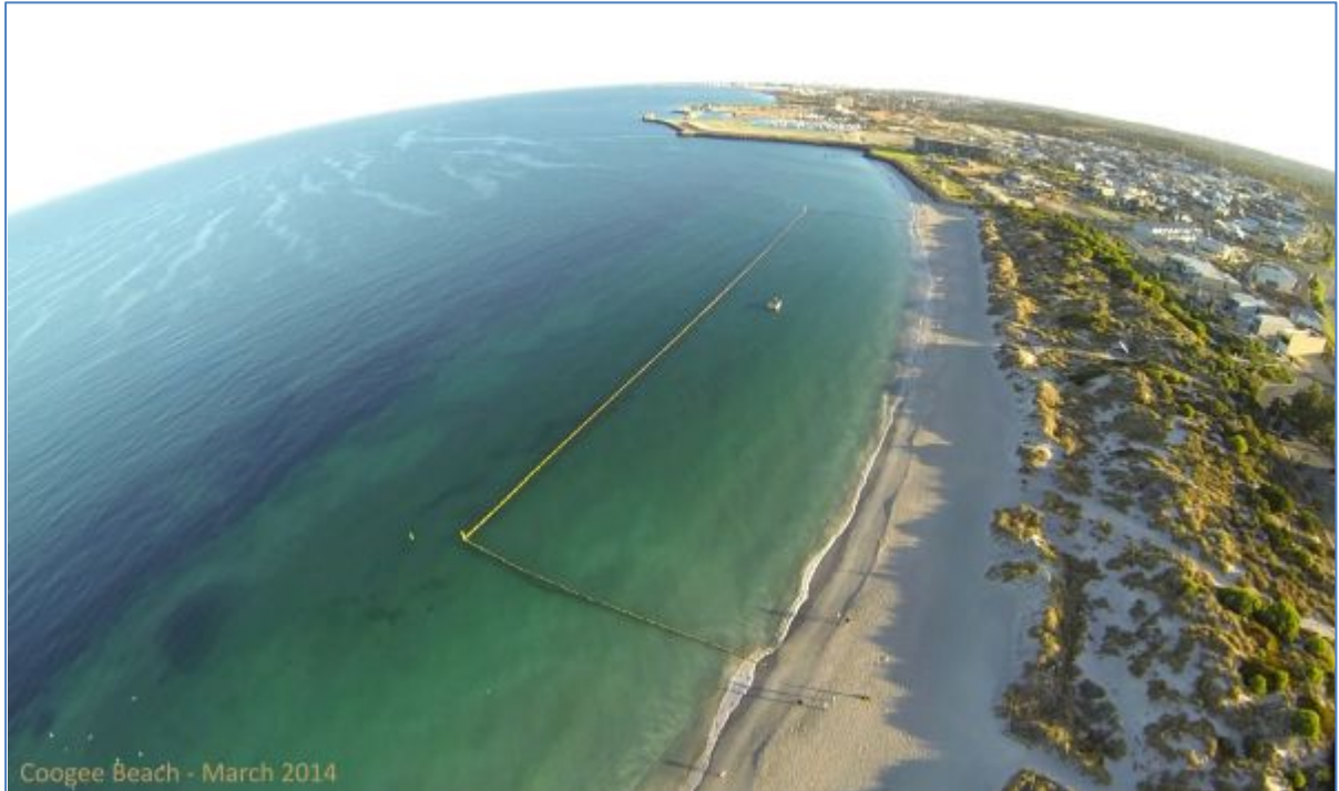
Image 1 – Eco Shark Barrier installed at Coogee Beach March 2014
