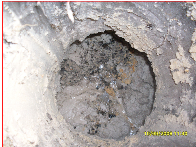
Plate 6: Ground water observed pooling into Test Pit 5
