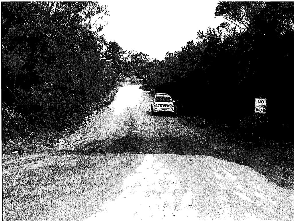
6. Attwell Road constructed with compacted limestone.
