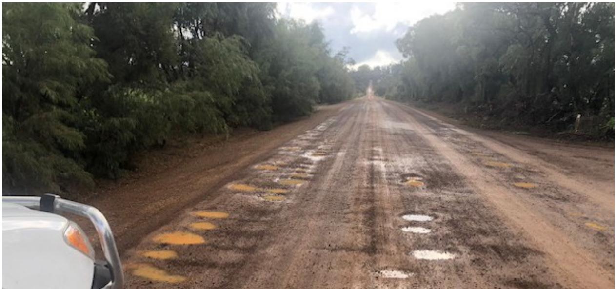
Deep potholes on long sections of the road.
