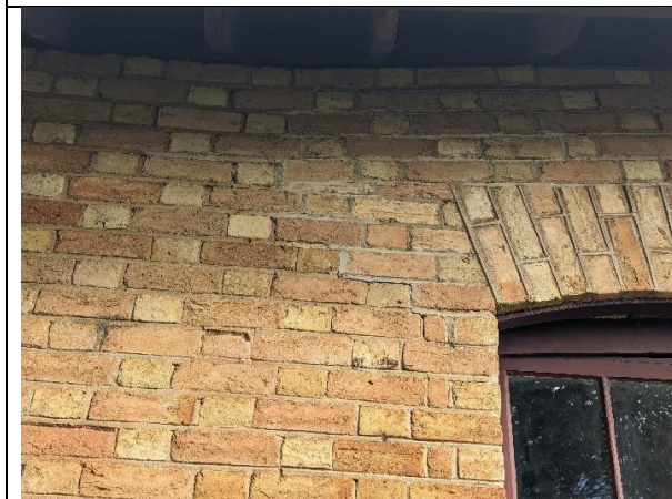
Photograph 5: Crack to mortar joints in external wall face and evidence of previous repairs
