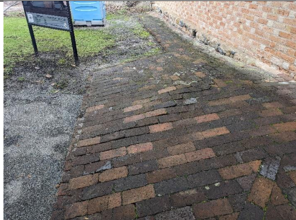
Photograph 2: Lifting pavers near building entrance
