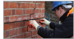
4. Using the HeliBar Insertion Tool, push one HeliBar into the grout to obtain good coverage
