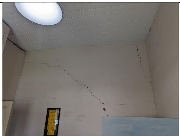
Photograph 8: Crack to plastered wall finish inside building
