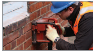
1. Rake out or cut slots into the horizontal mortar beds, a minimum of 500mm either side of the crack
