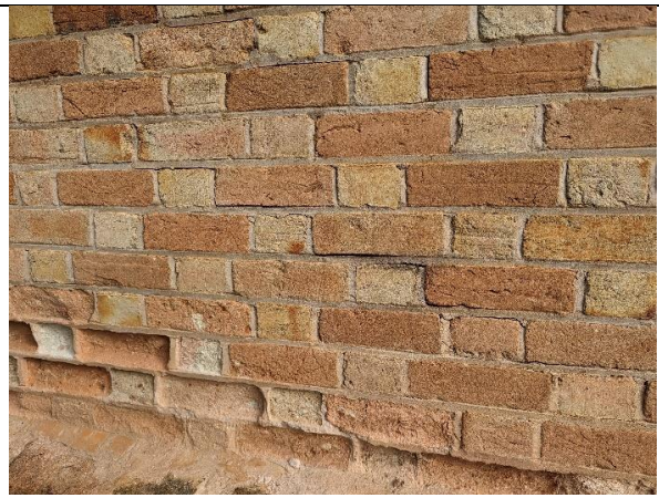
Photograph 4: Crack to mortar joints in external wall face
