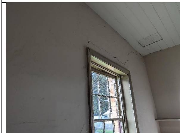
Photograph 7: Crack to plastered wall finish inside building
