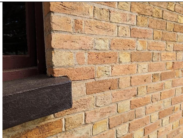
Photograph 6: Crack to mortar joints in external wall face
