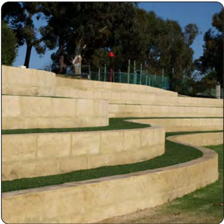
LIMESTONE RETAINING WALLS
