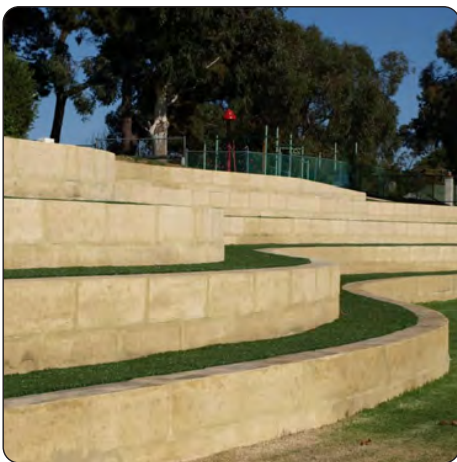
LIMESTONE RETAINING WALLS
