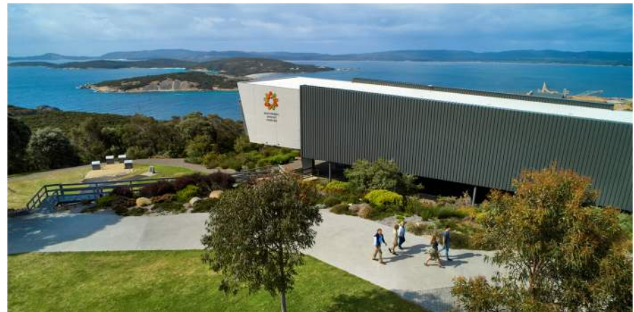
Wastewater treatment system at the National Anzac Centre Image: frances andrijich photography
