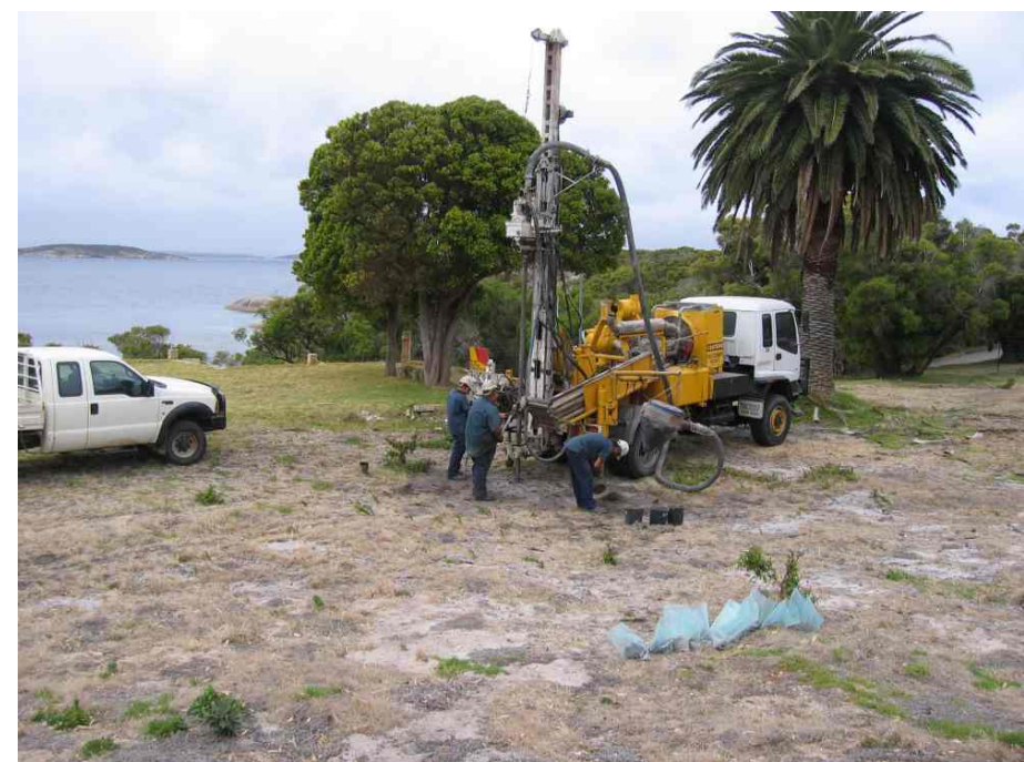
Figure 4D Drilling proposed development site
