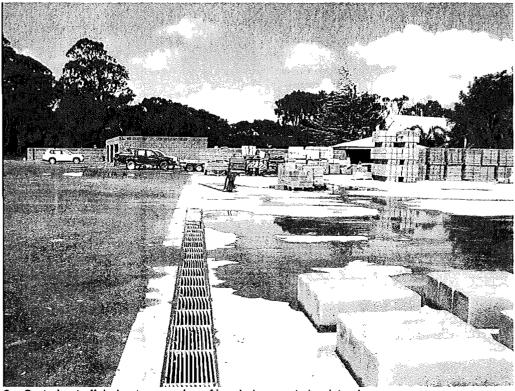
2. Grated cut off drain at open edge of bunded concrete hardstand
