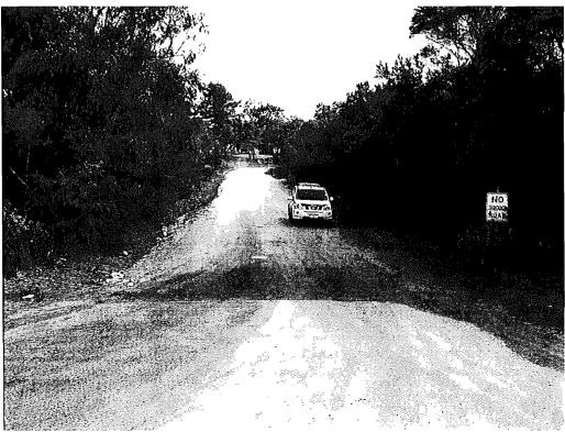
6. Attwell Road constructed with compacted limestone.
