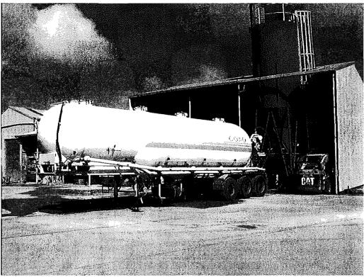
1. Tanker delivery of cement directly to Hopper
