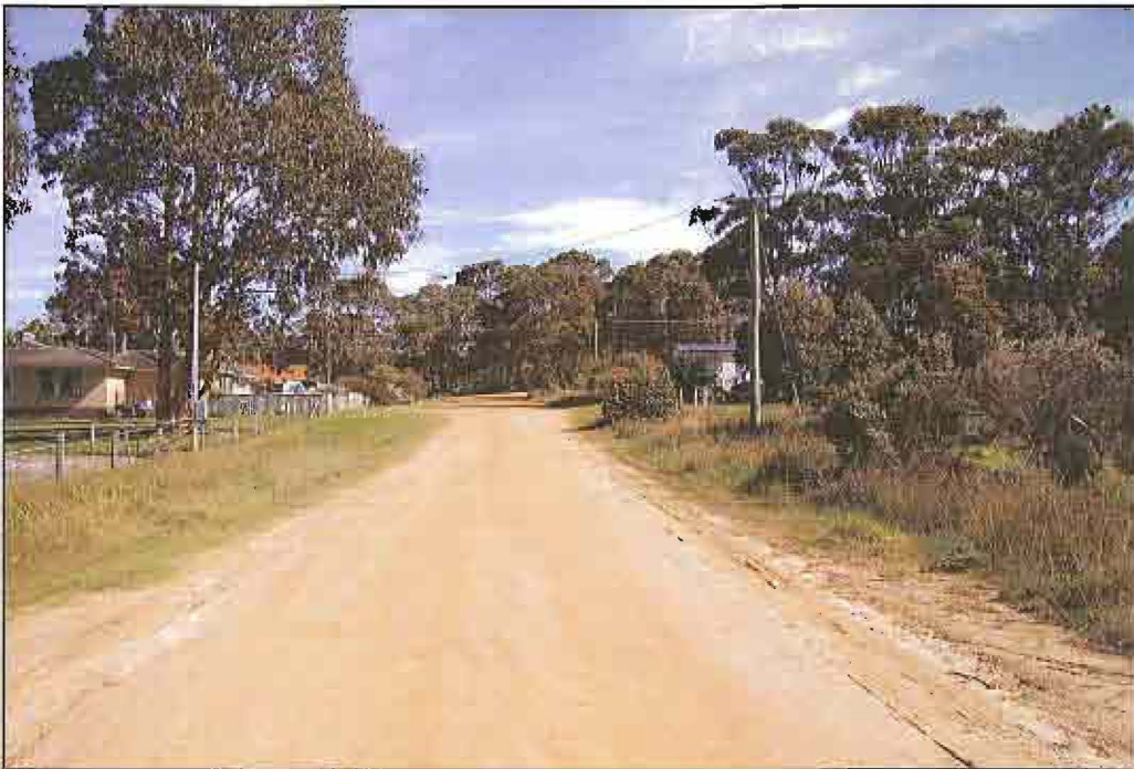
Figure 5 – View of Hadley Street looking east towards Baker Street.
