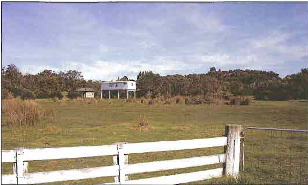
Figure 3 – View of house and outbuilding on Lot 107, west from Francis Street.
