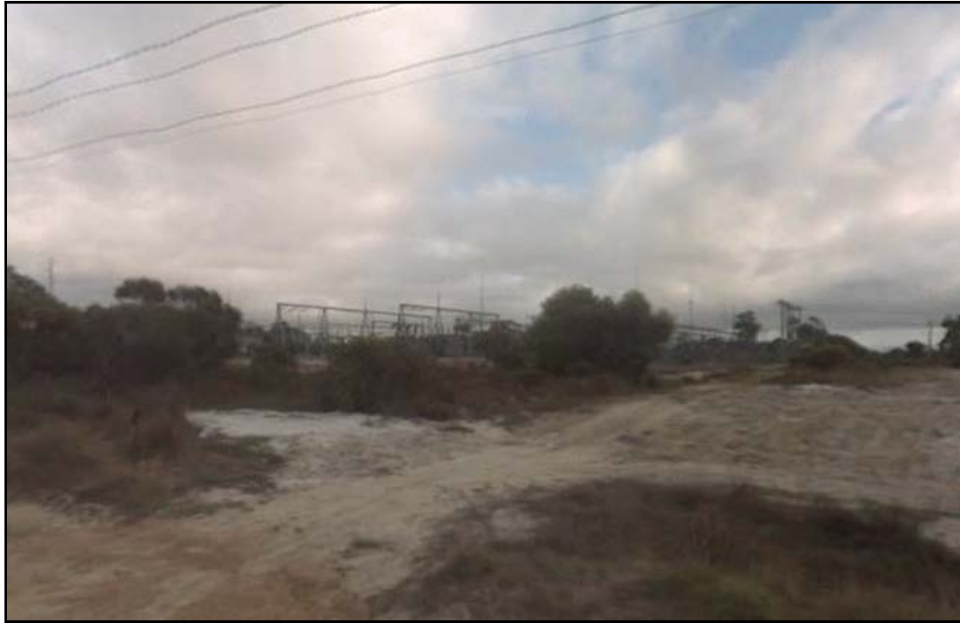
Figure 5.5: View of Western Power Sub-Station site from Federal Street. Vegetation is either cleared or kept in a fuel reduced state across the entire site.
