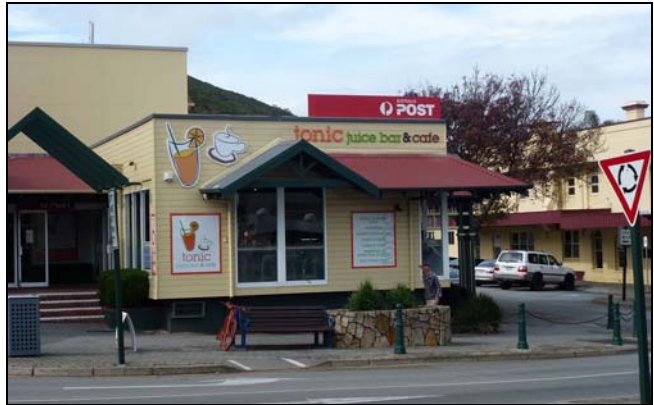
Roof sign unrelated to use below and not integrated with building design.
