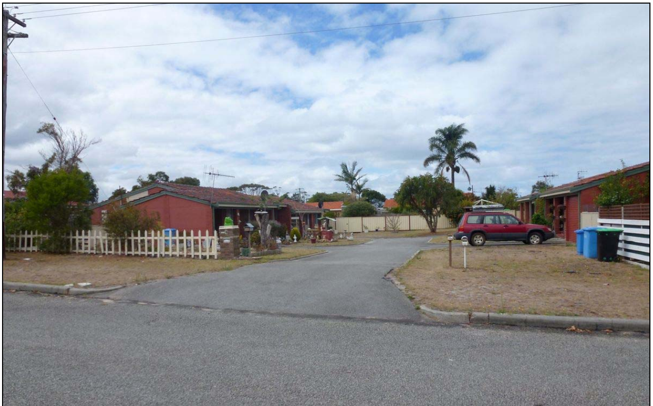
Photo 17: Grouped Housing on Bellingham Street.
