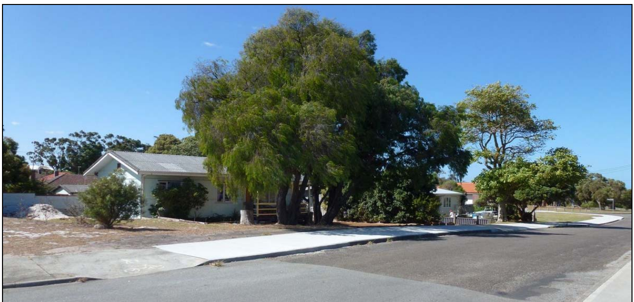
Photo 7: Lots on the northern side on Mokare Road.
