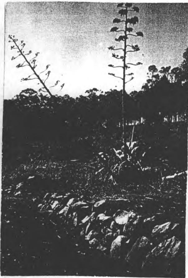
The old "Candyup" foundations.
