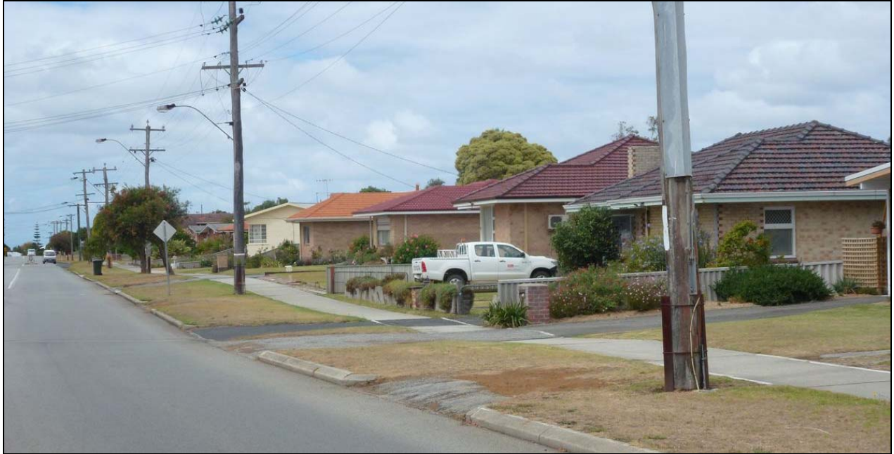
Photo 8: Housing on southern side of Angove Road.
