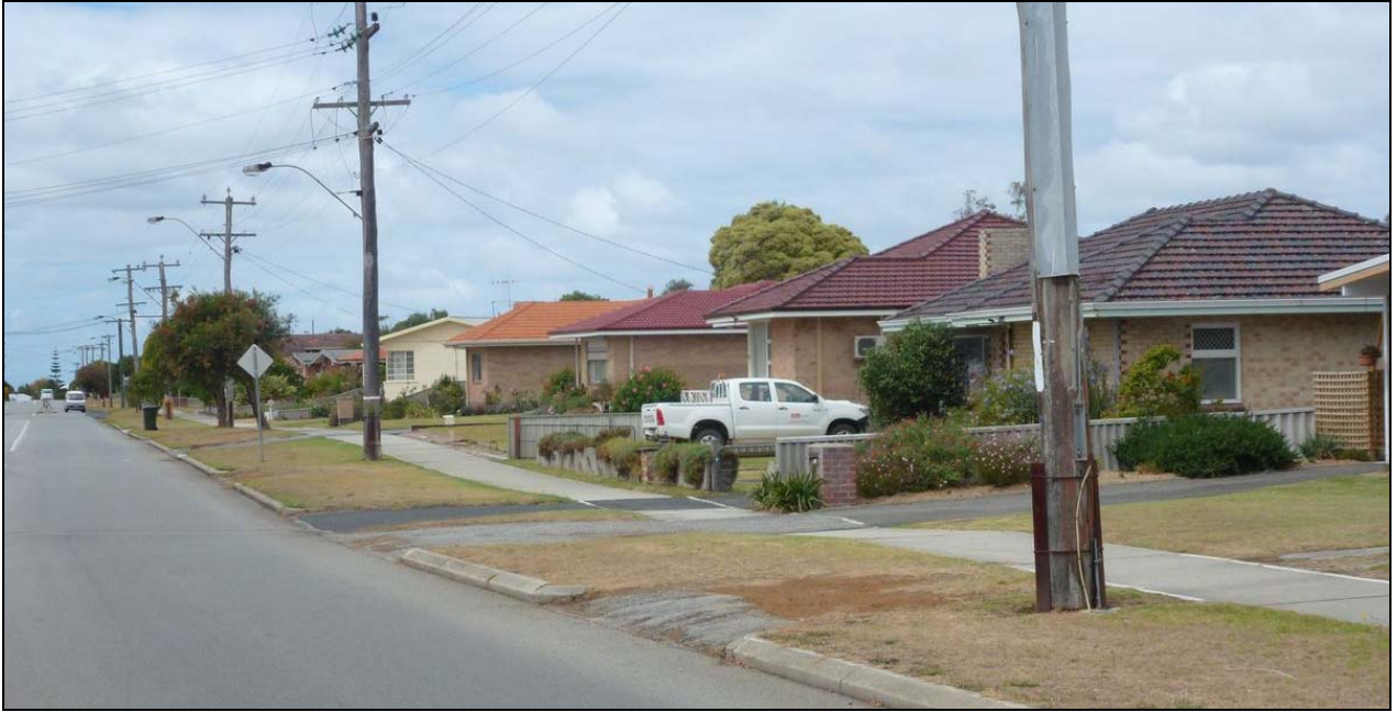
Photo 8: Housing on southern side of Angove Road.
