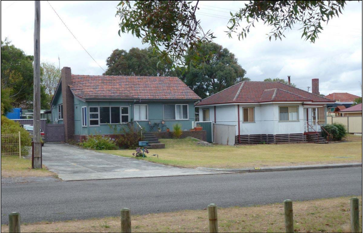
Photo 16: Fibro cottages in Burville Street.
