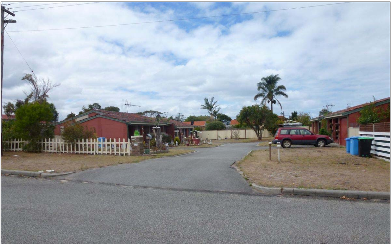
Photo 17: Grouped Housing on Bellingham Street.
