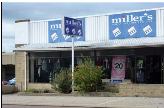
Freestanding sign inappropriate to town centre.
