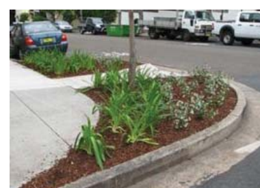
Typical crossing point where planting is used to direct traffic
