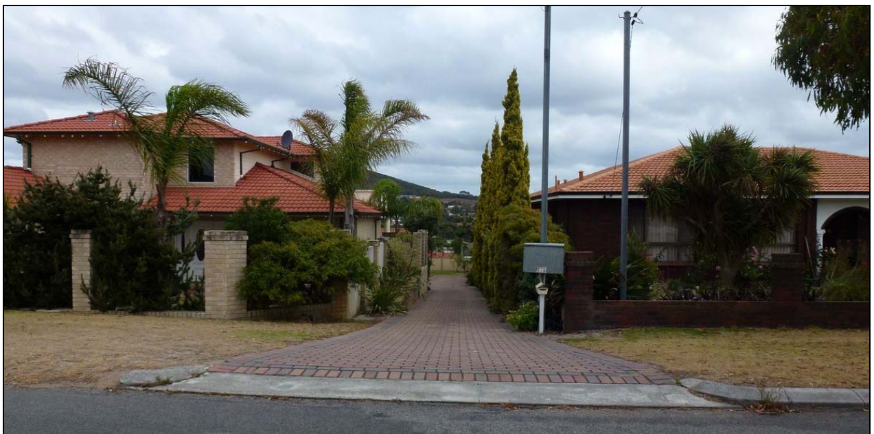
Photo 13: Redeveloped brick & tile housing on Hillman Street.
