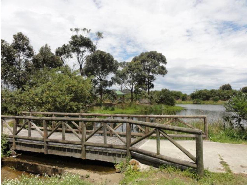
Image 4.: Wetland outfall to degraded stream. This wetland has an integrated drainage function attenuating storm water runoff from urban areas and providing passive and active recreation whilst providing a biological function of improving water quality whilst providing habitat to aquatic fauna including the (Aboriginal significant) long neck tortoise and native waterbirds.
