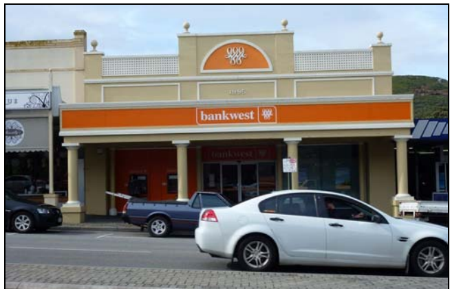
Signage fully integrated with design of building.
