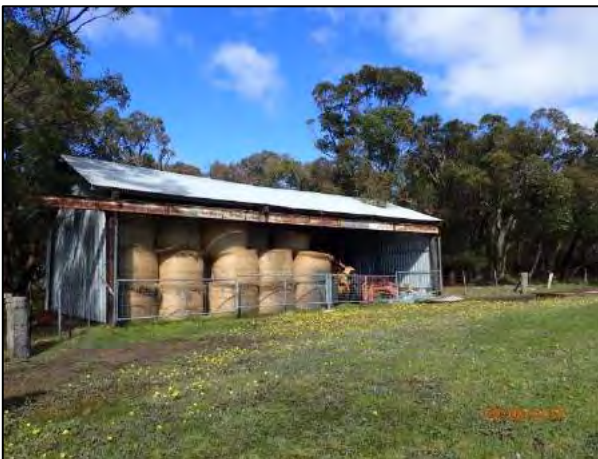
Photograph 3 – View of hay and machinery shed located in the north of Lot 521 Mercer Road.
