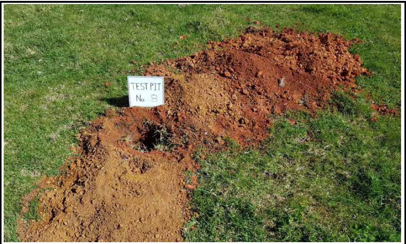
Test Pit No. 8 Spoil
