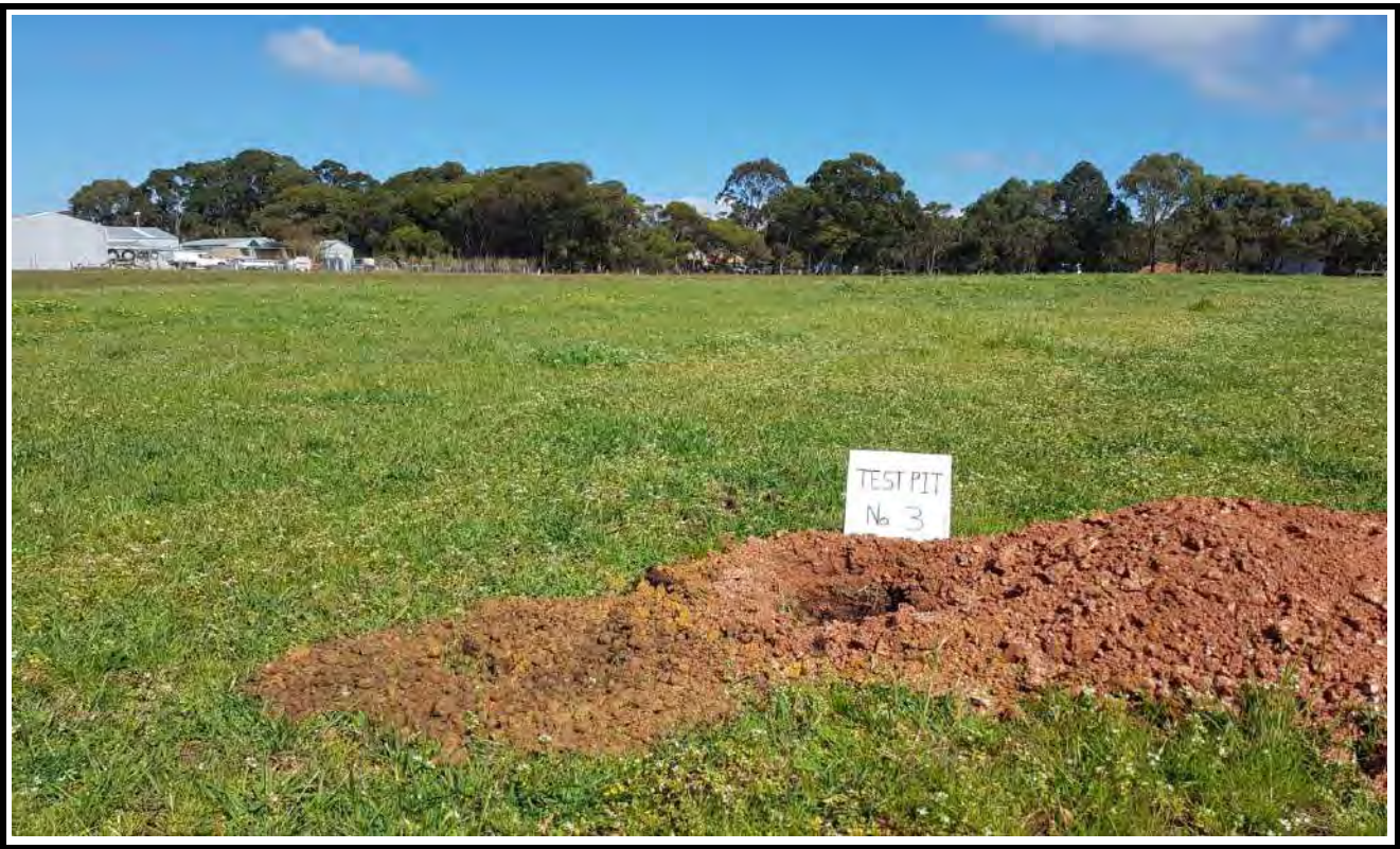
Test Pit No. 3 Excavation
