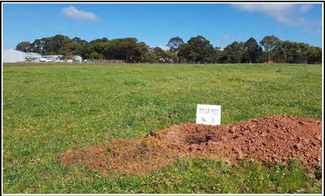
Test Pit No. 3 Excavation
