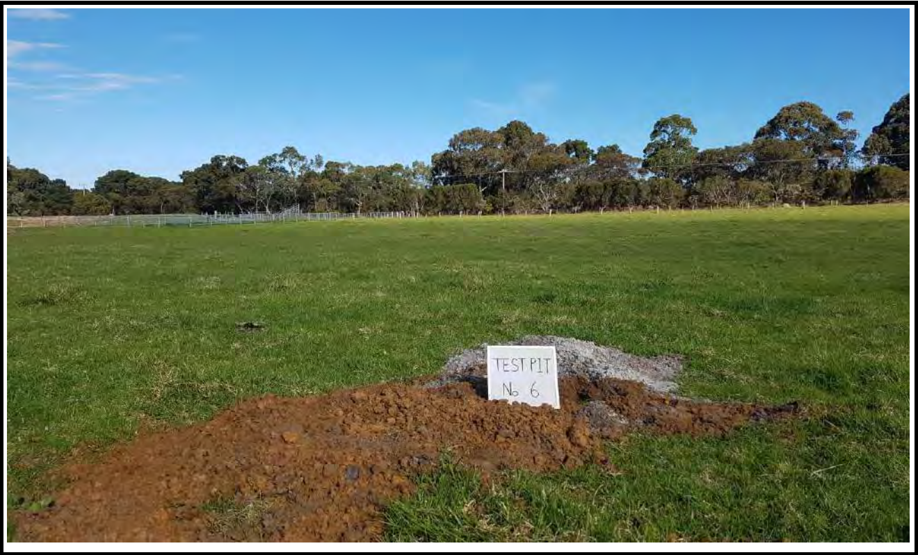
Test Pit No. 6 Excavation
