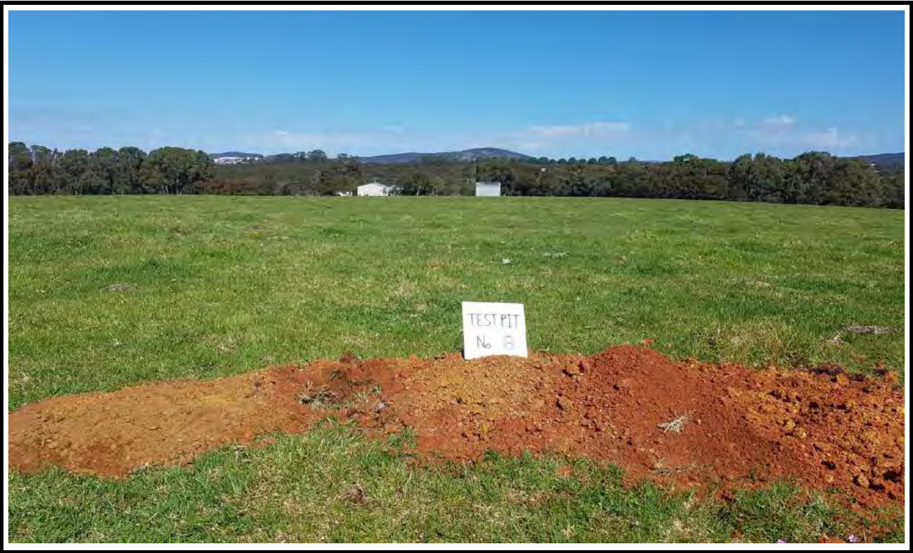
Test Pit No. 8 Excavation
