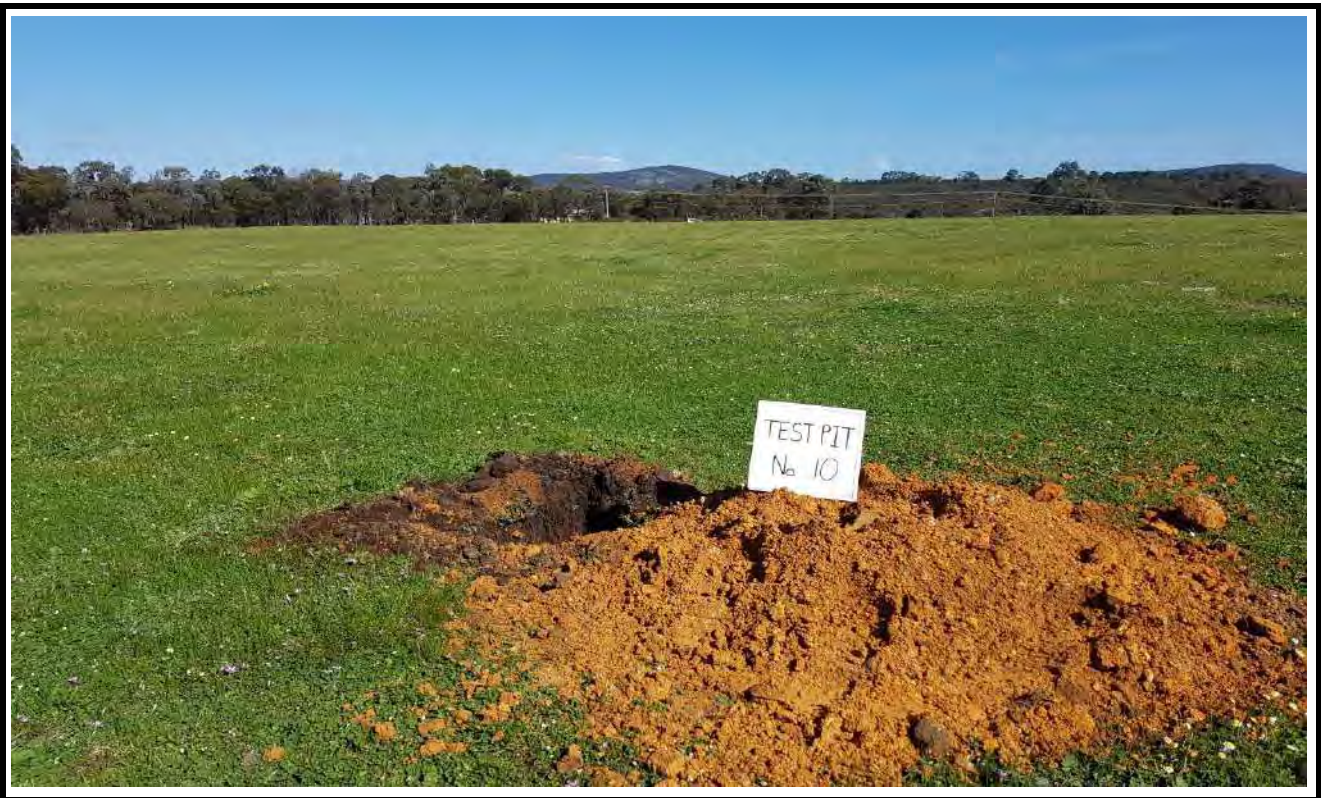
Test Pit No. 10 Excavation
