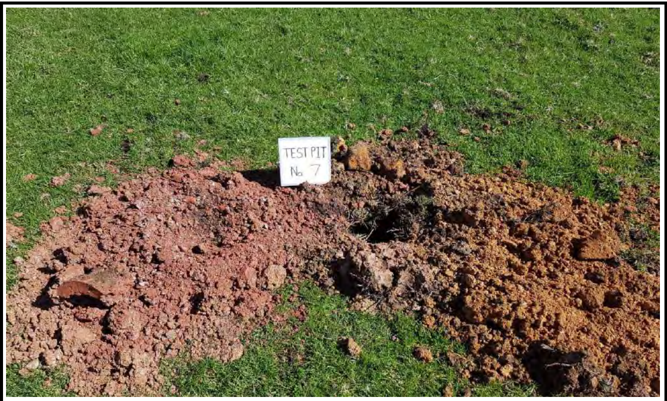
Test Pit No. 7 Spoil
