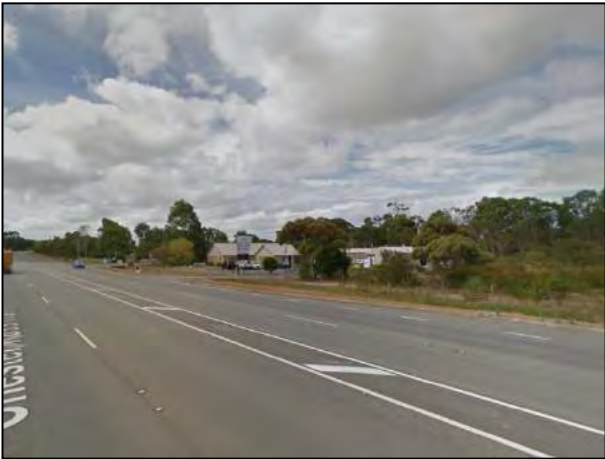
Photograph 5 – View of Albany Business Centre along Chester Pass Road to the south-west of Subject Site.
