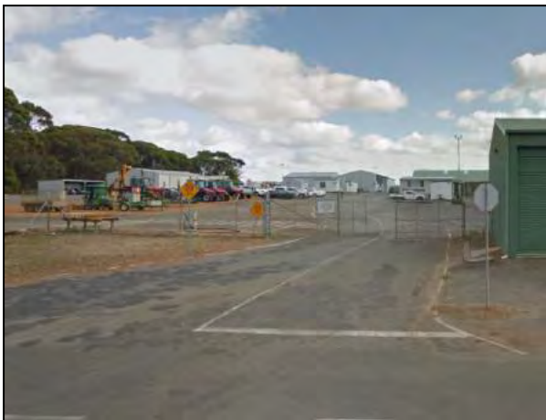
Photograph 7 – View of City of Albany holding facilities along Mercer Road to the south of Subject Site.
