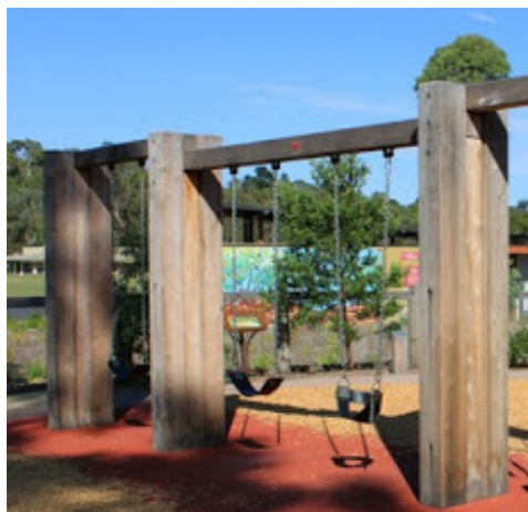
Swing set using large timber supports
