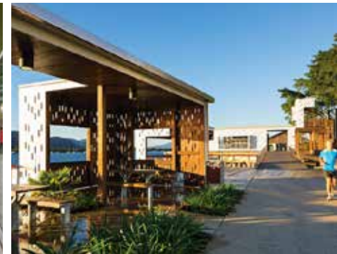
image source: ArchitectureAU, Cairns Foreshore
