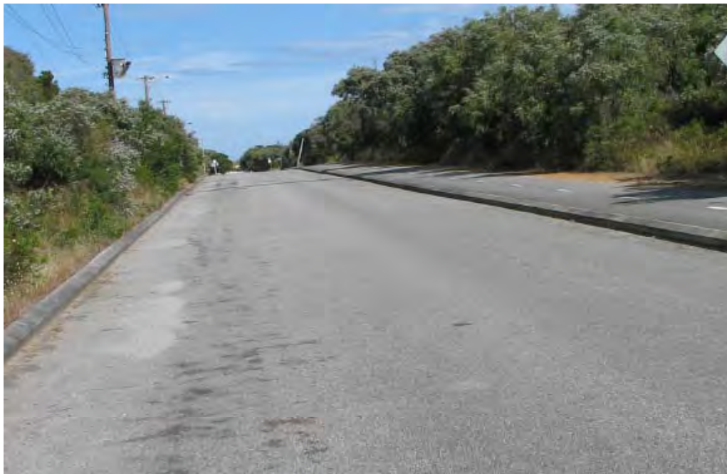
Plate 12 – Griffiths Street road pavement - looking south
