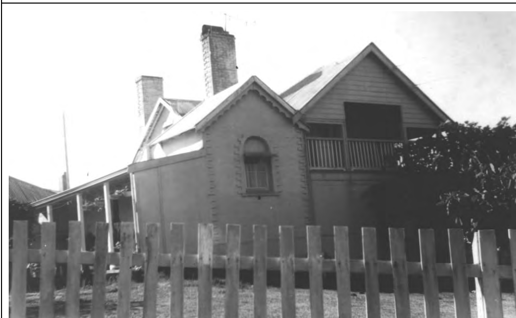
C1950s showing former skillion verandah with enclosure on west side [P2101 Albany History Collection]
