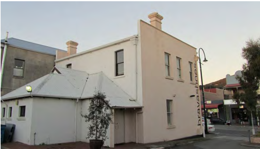
South-west elevation [H Munt]
