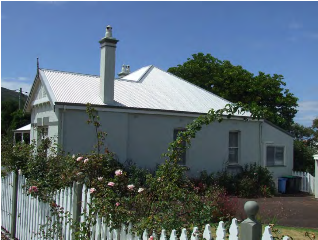
North-west elevation [H Munt 2018]
