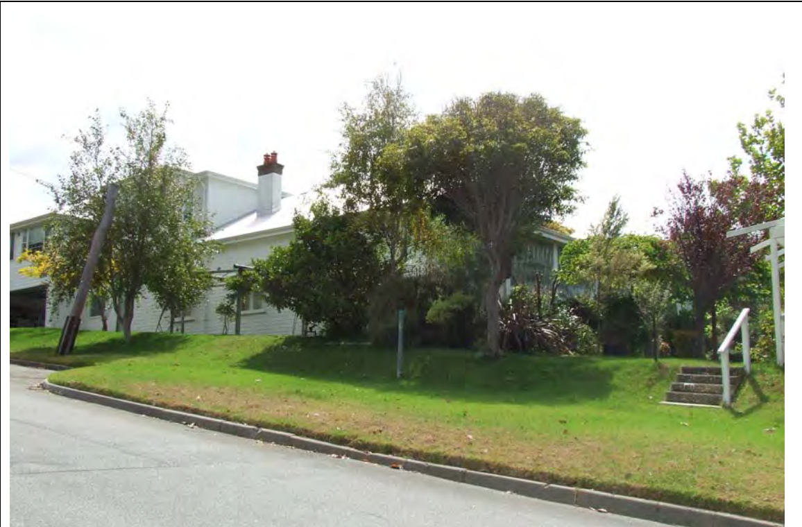
South-west elevation showing two storey addition at rear [H Munt 2018]
