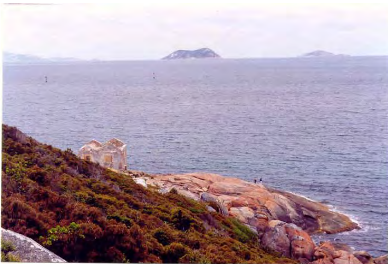
Lighthouse Keepers Cottage [Heritage Today 2000]
