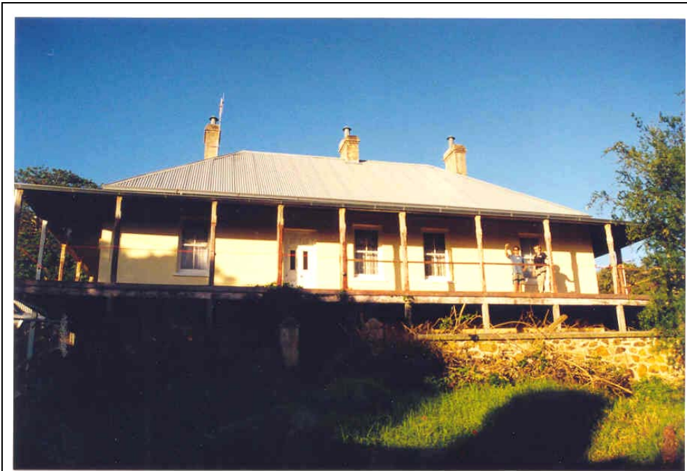
South elevation [Heritage Today 2000]
