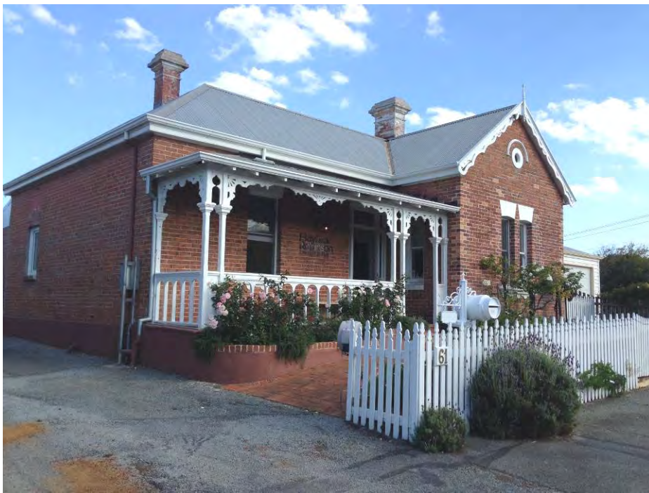
North-east elevation [H Munt 2017]
