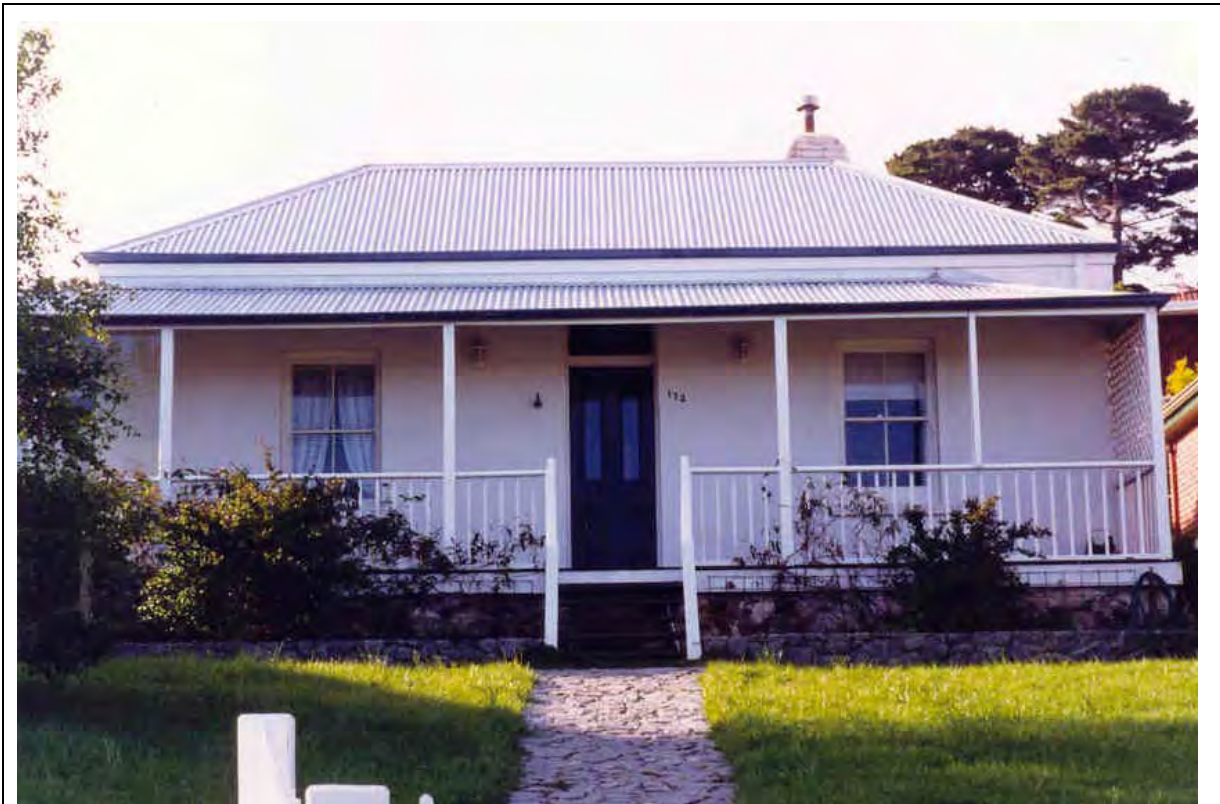
South (front) elevation [H Munt 2018]
