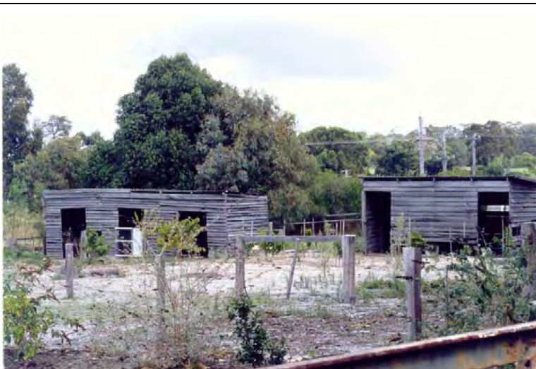
The stables next to Willyung Cottage (not original) [Heritage Today 2000]
