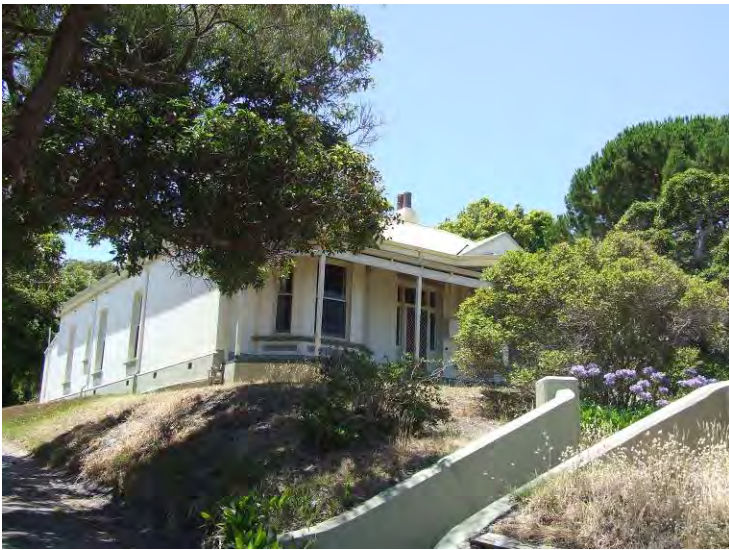
South-west elevation [H Munt 2017]
