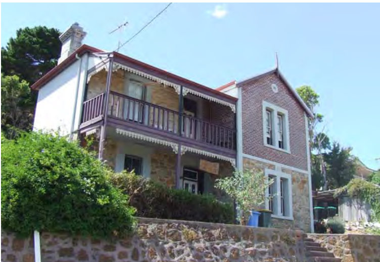
South-west elevation [H Munt 2018]
