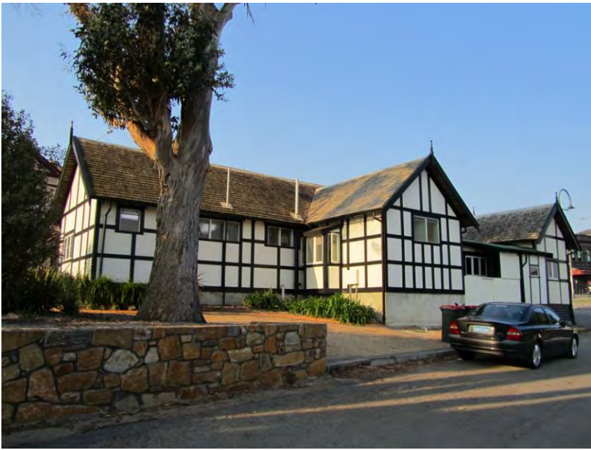
Rear (south) elevation [H Munt 2010]
