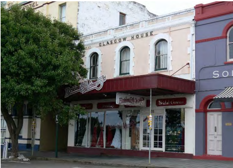
c2000 showing the former cantilevered awning [Heritage Today 2000]
