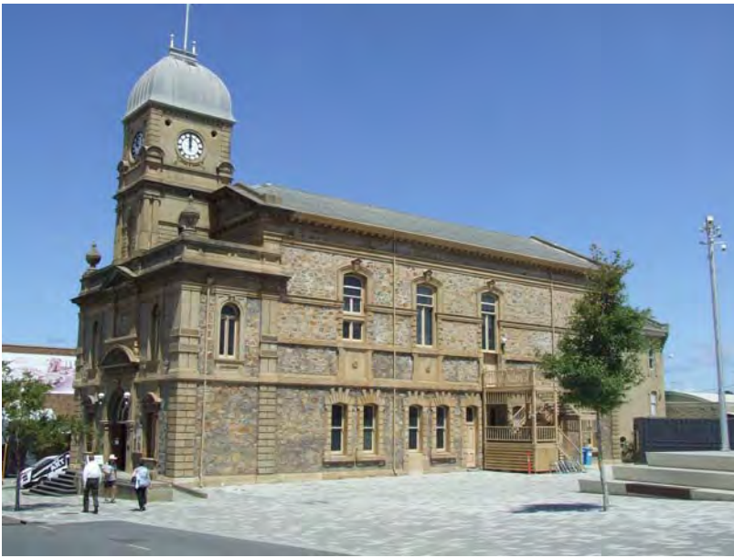
North-east elevation [H Munt 2018]
