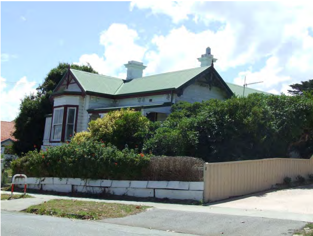
South-east elevation [H Munt 2018]
