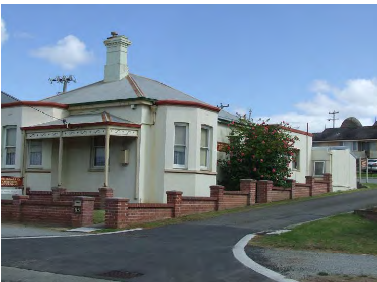
North-east elevation [H Munt 2016]
