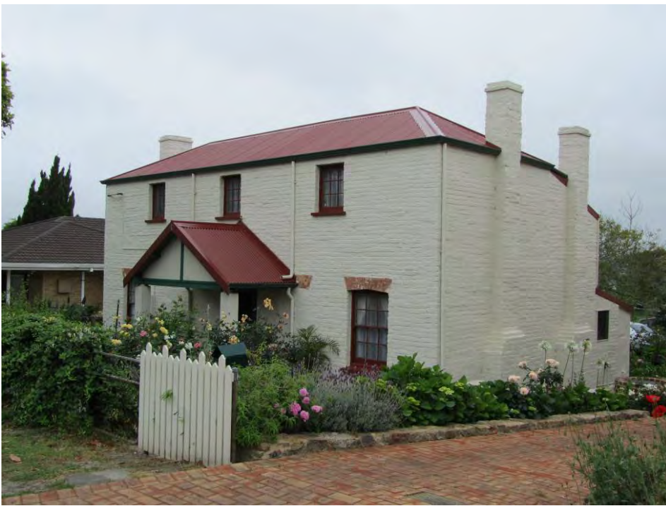
South-east elevation [H Munt 2015]
