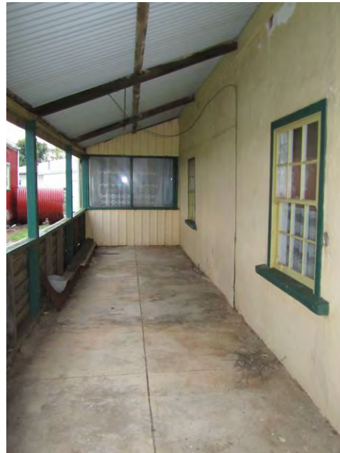
South verandah [H Munt 2011]
