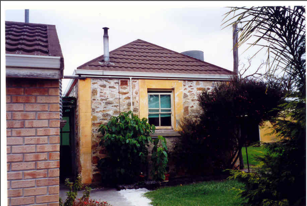
View of Pendeen Homestead from the rear [Heritage Today 2000]
