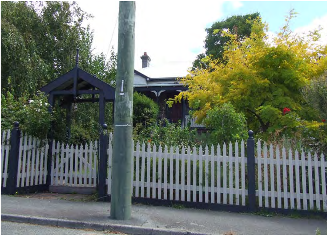
South (front) elevation [H Munt 2018]
