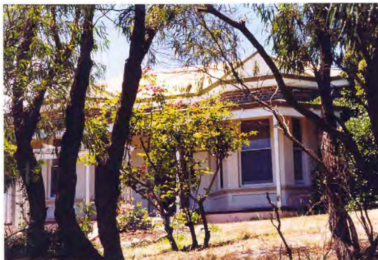
South elevation [Heritage Today 2000]
