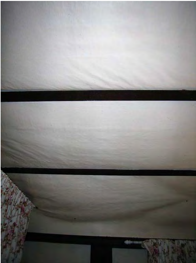
Interior hessian sheeting in ceiling [H Munt 2008]
