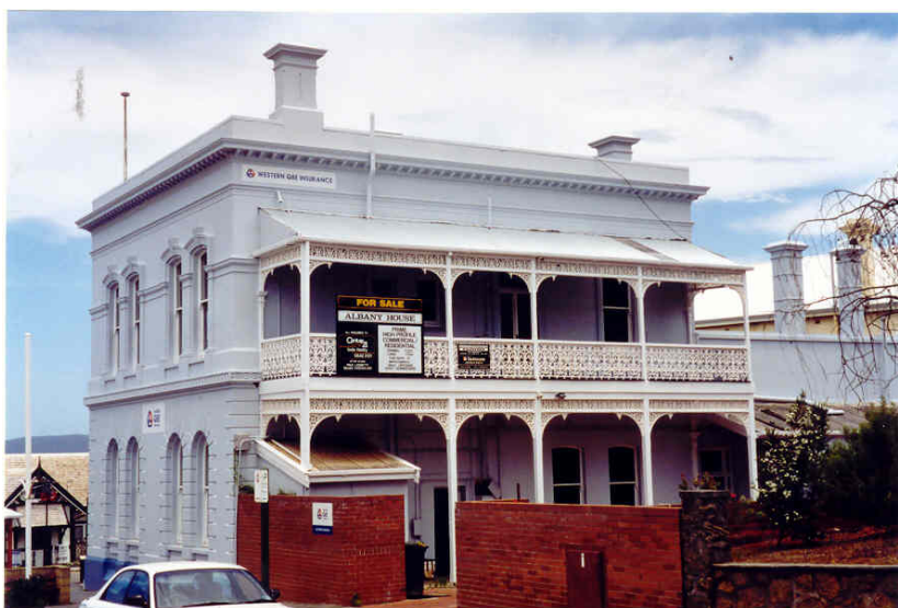
Albany House, rear view [Heritage Today, 2000]
