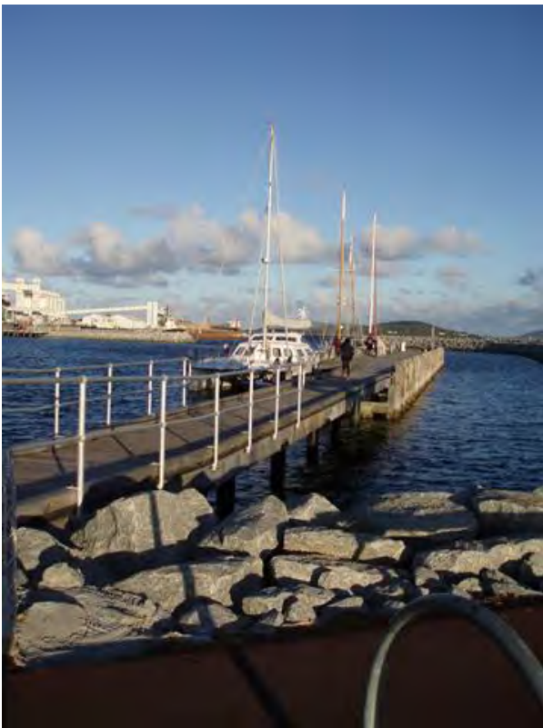
2011, after foreshore development, south east arm [State Heritage Office]
