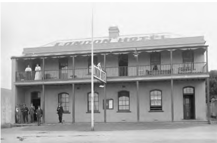
1907 – Sims original hotel (second London Hotel c1871) before renovations [SLWA 5323B/22]
