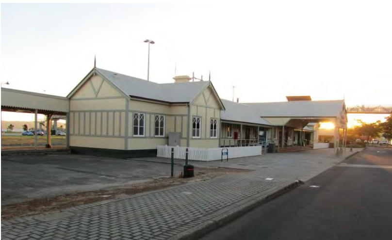
Railway Station north elevation [H Munt 2011]
