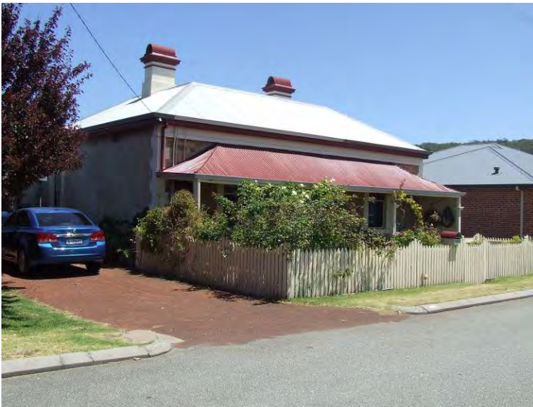
North-east elevation [H Munt 2017]
