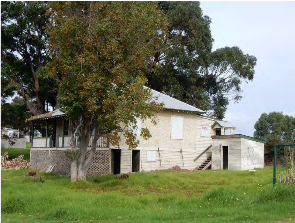
North elevation [H Munt 2017]
