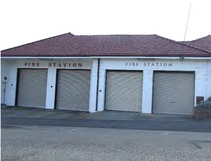
Fire Station, detail of garages (east) [H Munt 2016]
