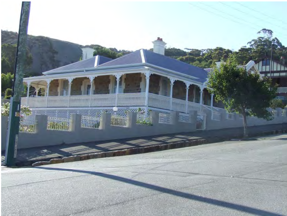
South-east elevation [H Munt 2018]
