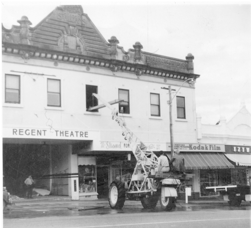
c1970s St Alban's Buildings, Regent Theatre section being demolished [AHC ICR1138962]
