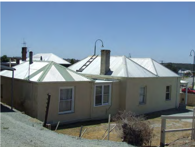
South-west elevation [H Munt 2016]
