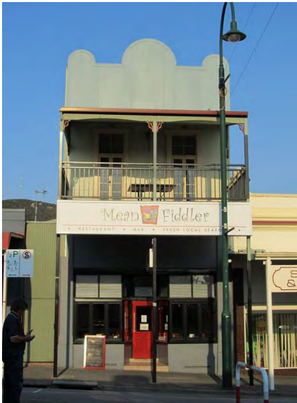
Mean Fiddler Restaurant is a remnant of the original two storey section of St Albans Buildings [H Munt 2010]
