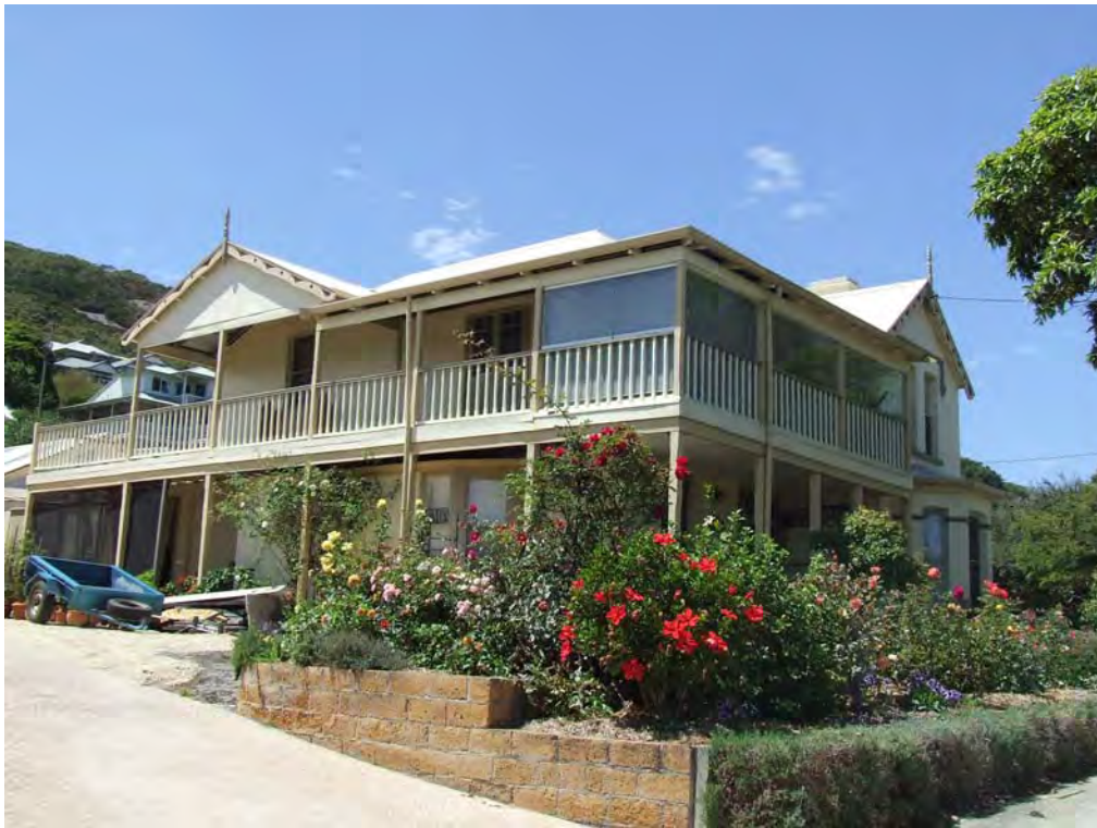
South-west elevation [H Munt 2018]
