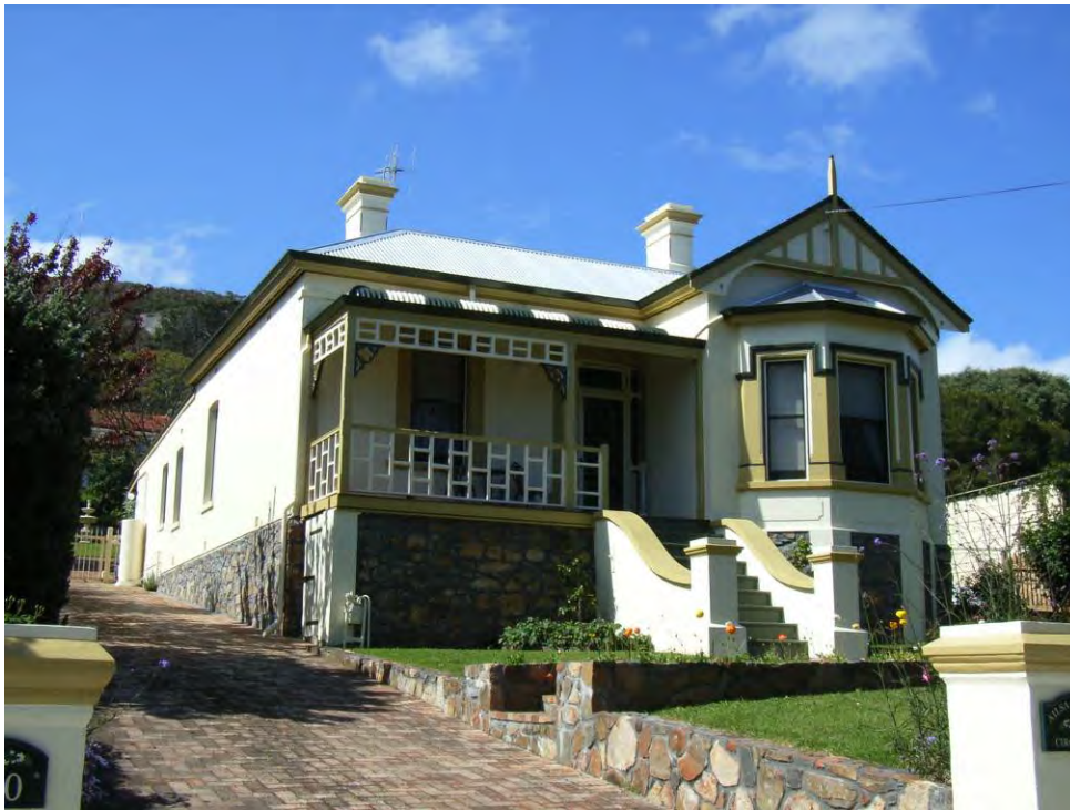
South-west elevation [H Munt 2008]
