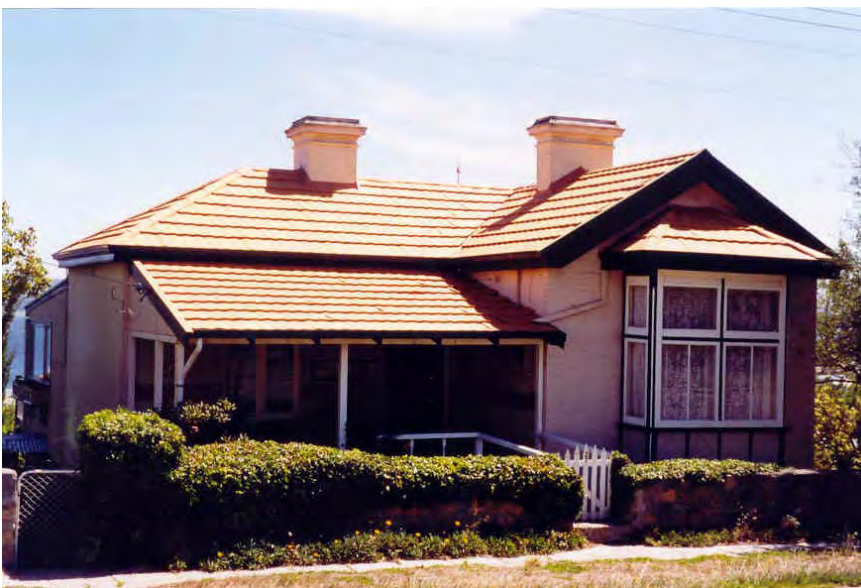
North-east elevation [Heritage Today 2000]
