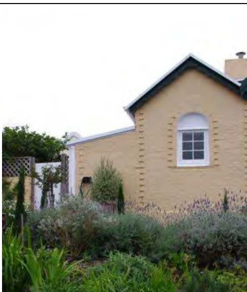
South elevation, west end [H Munt 2010]
