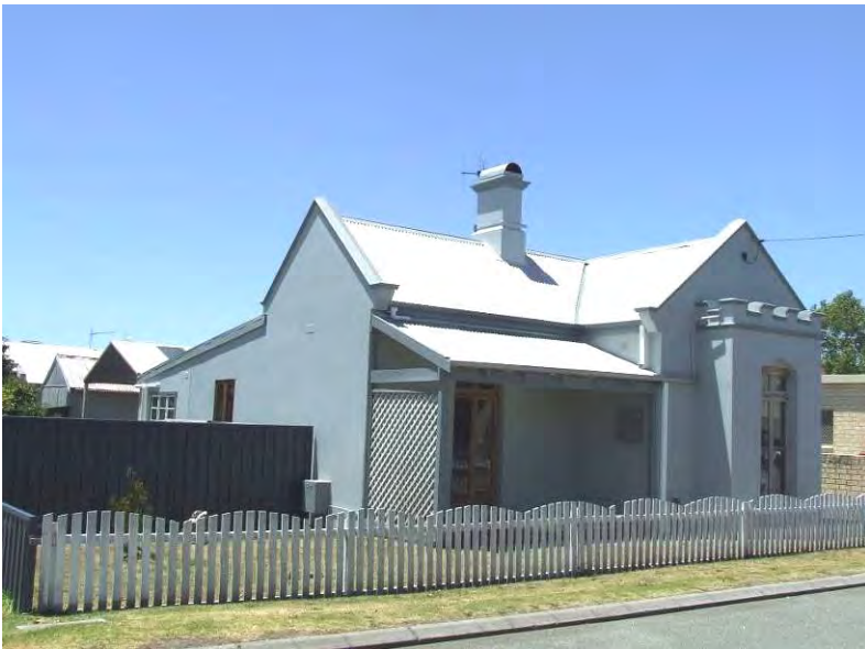
South-west elevation [H Munt 2017]
