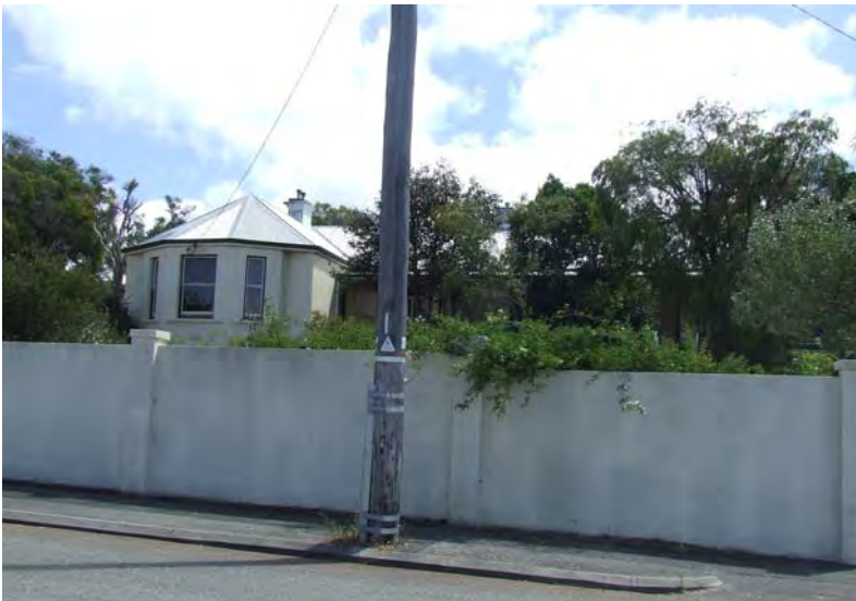
South (front) elevation [H Munt 2018]
