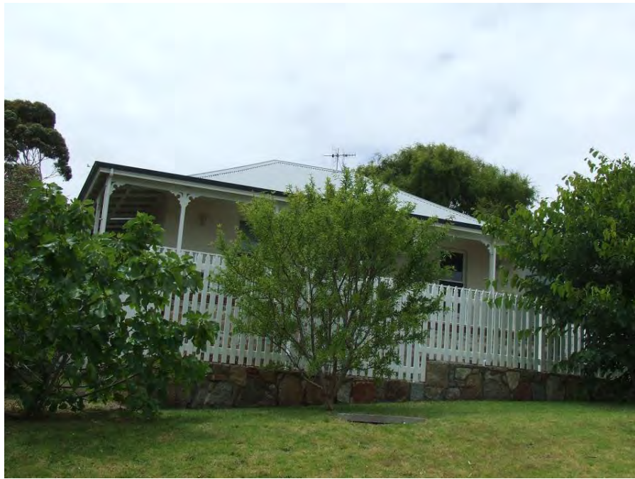
South-west elevation [H Munt 2015]
