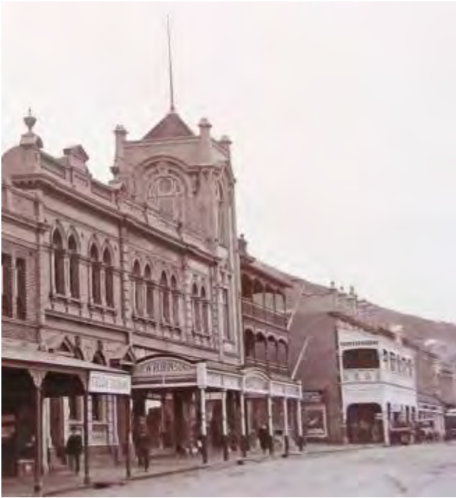
c1914 showing the tower and flagpole at the east end [detail, AHC]
