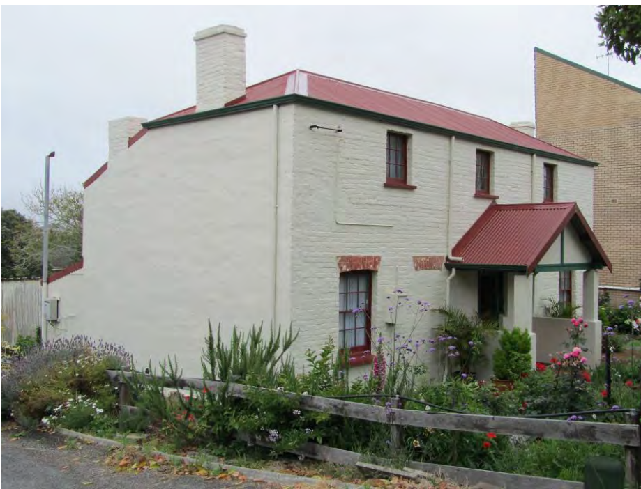
South-west elevation [H Munt 2015]
