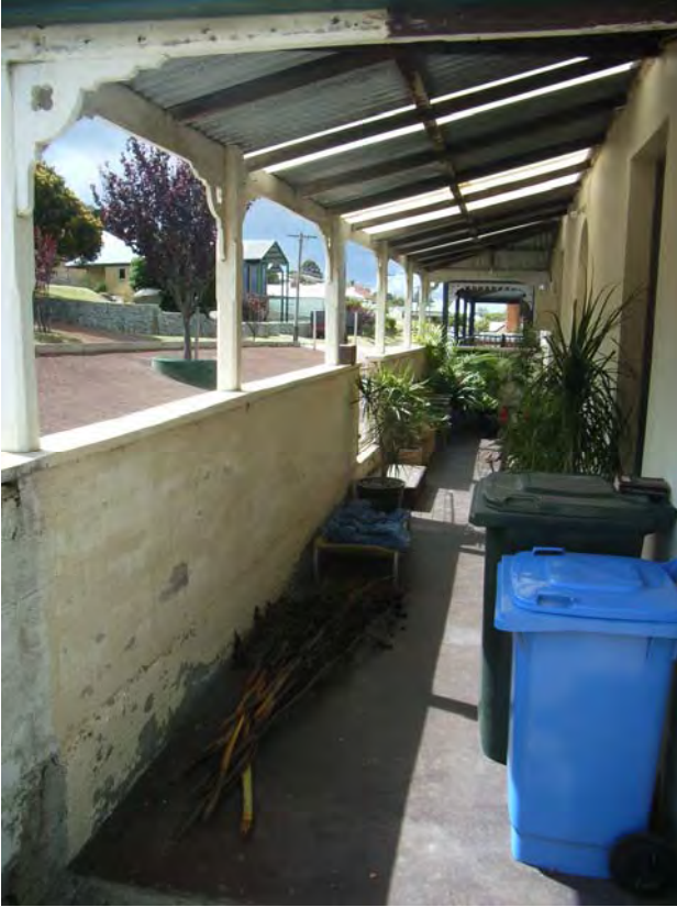
Before alterations and additions [H Munt 2007]
