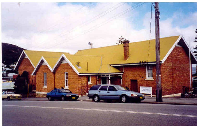
Building 2 [Heritage Today 2000]
