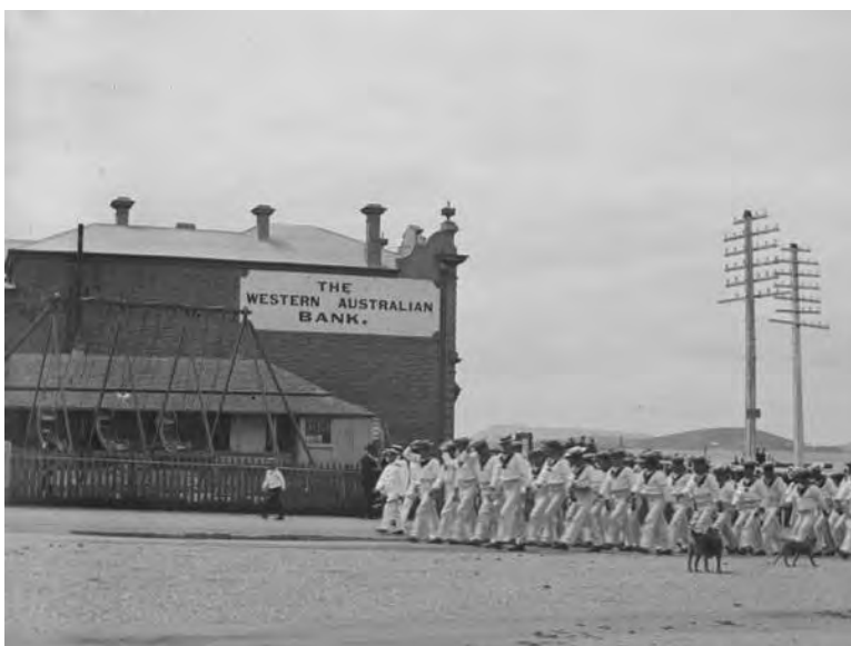
West elevation from York Street c1908 before the Empire Buildings was constructed [SLWA-b2856855-4]
