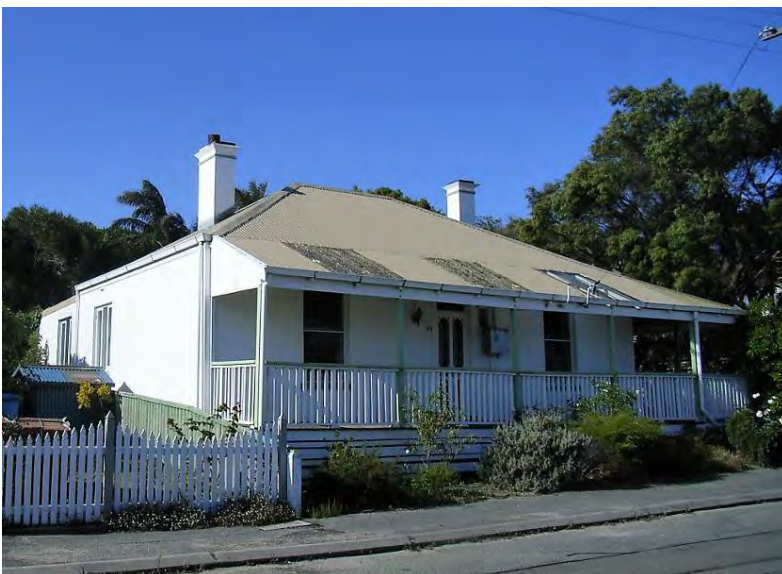
South-west elevation [H Munt 2008]
