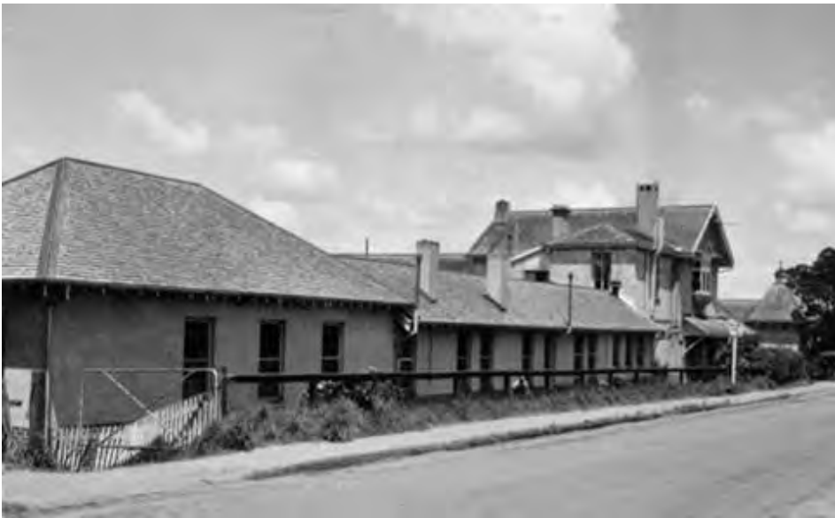
1954 – note the shingle roof on the eastern wing [SLWA 011006D/816B]
