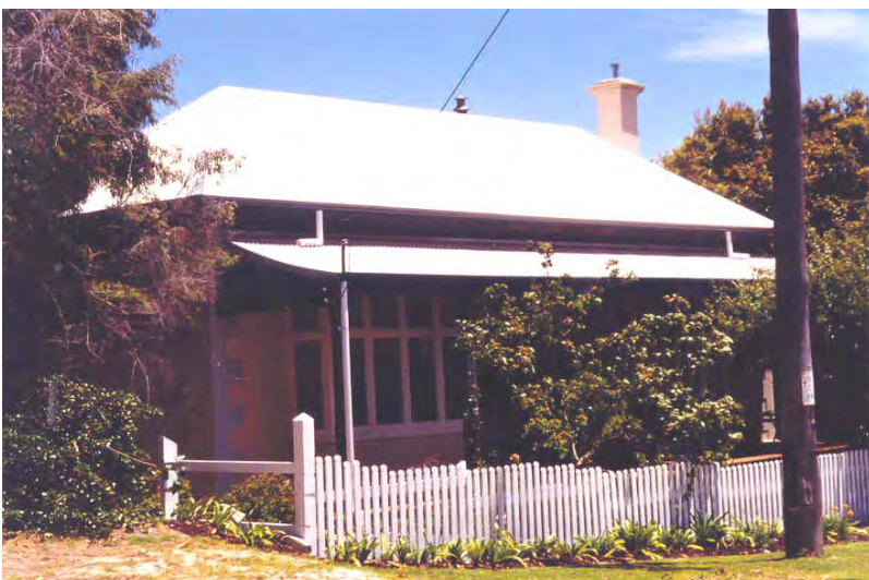
North-east elevation [Heritage Today 2000]
