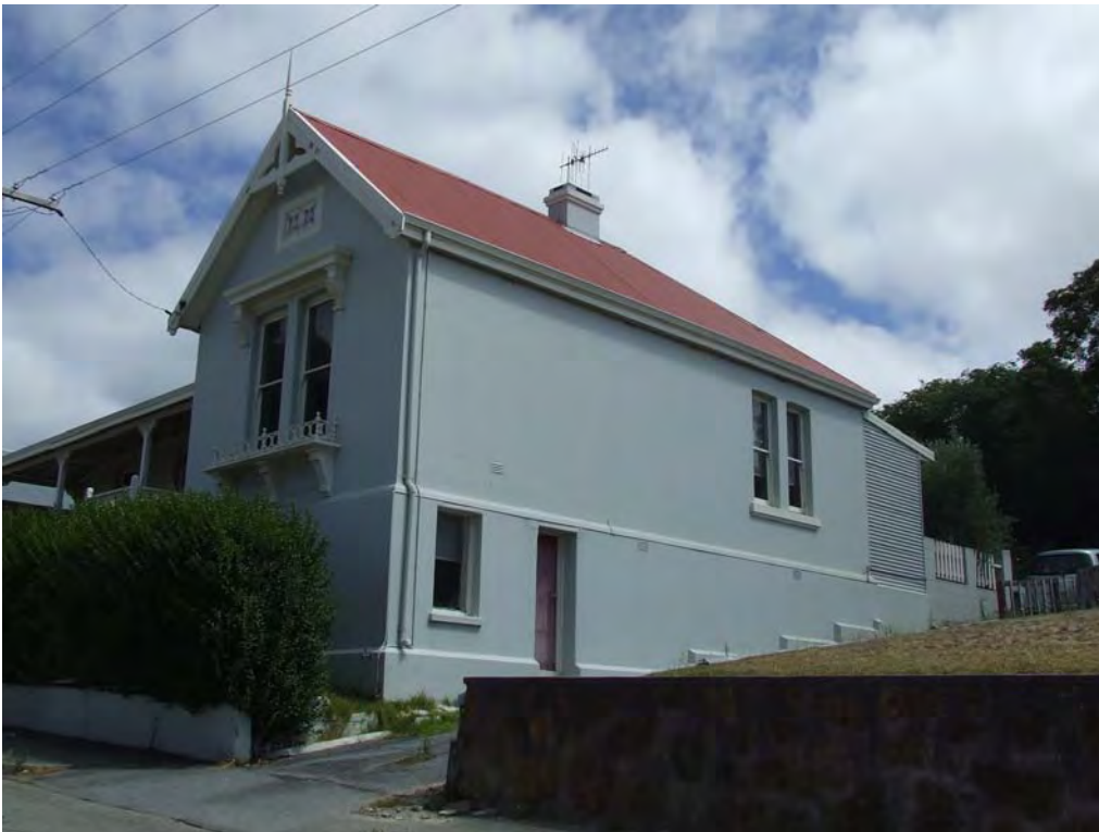
South-west elevation [H Munt 2018]
