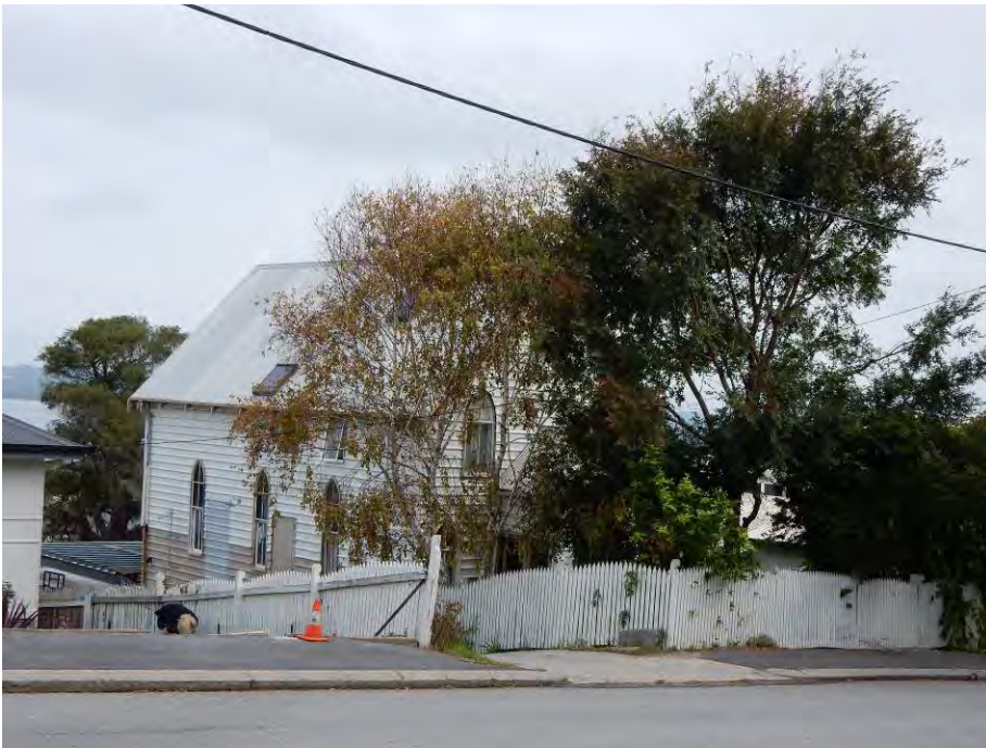
North-east elevation [H Munt 2017]
