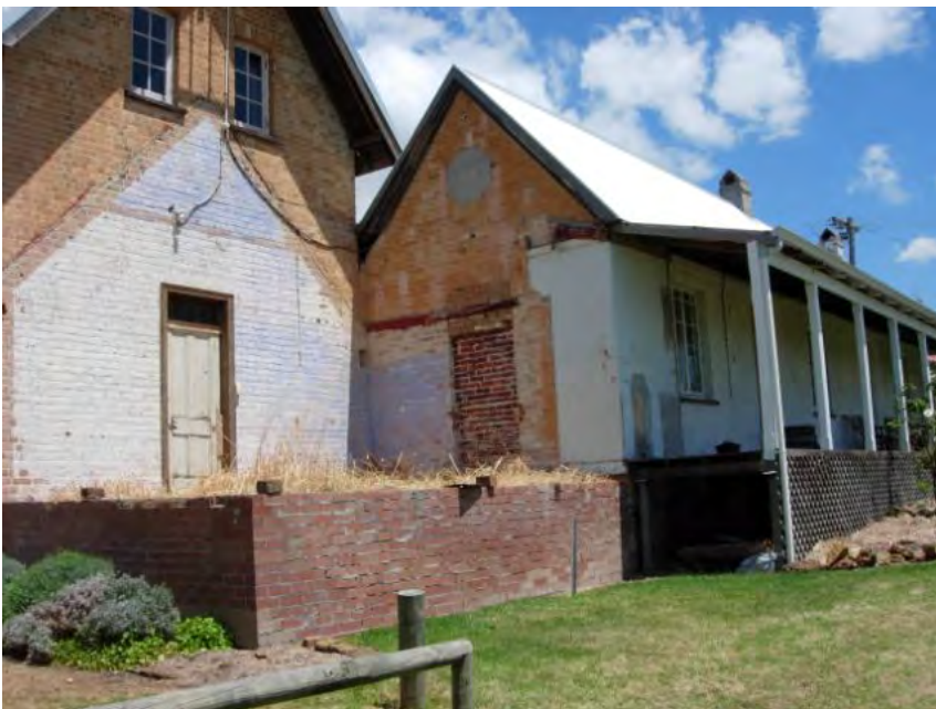
North east elevation during renovations 2009 [H Munt 2009]
