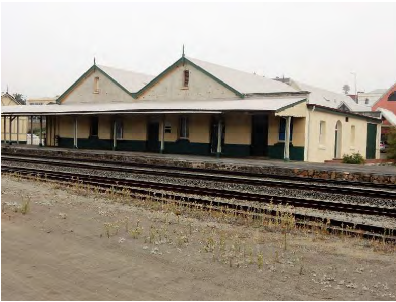
Railway Station Bond Store south-east elevation [H Munt 2017]
