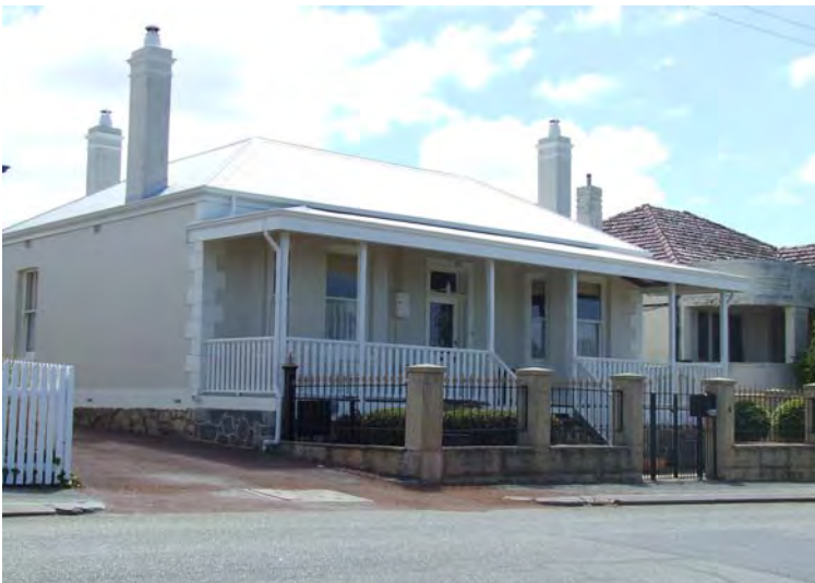
South-west elevation [H Munt 2018]
