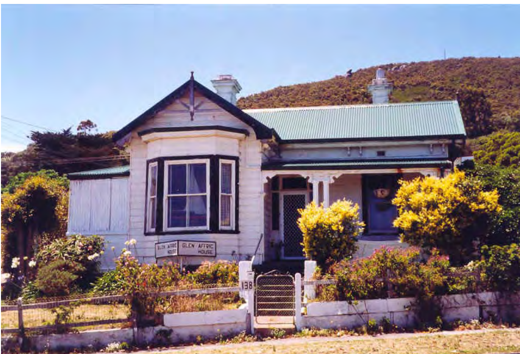
South elevation [Heritage Today 2000]
