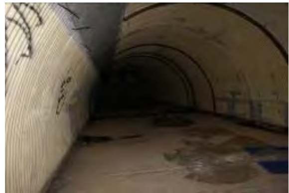
Tunnel/bunker [City of Albany, 2010]
