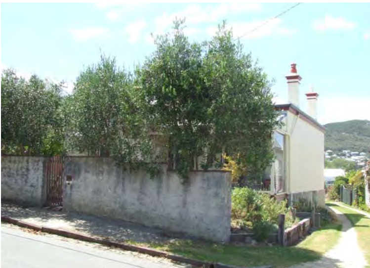
South-west elevation [H Munt 2018]
