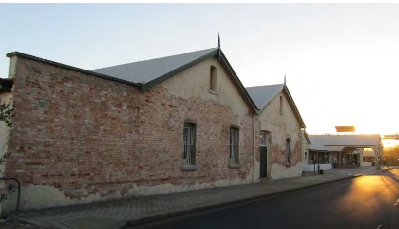
Bond store prior to conservation works [H Munt 2011]
