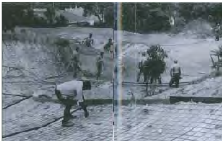
Laying the foundations 1976 [source City of Albany]
