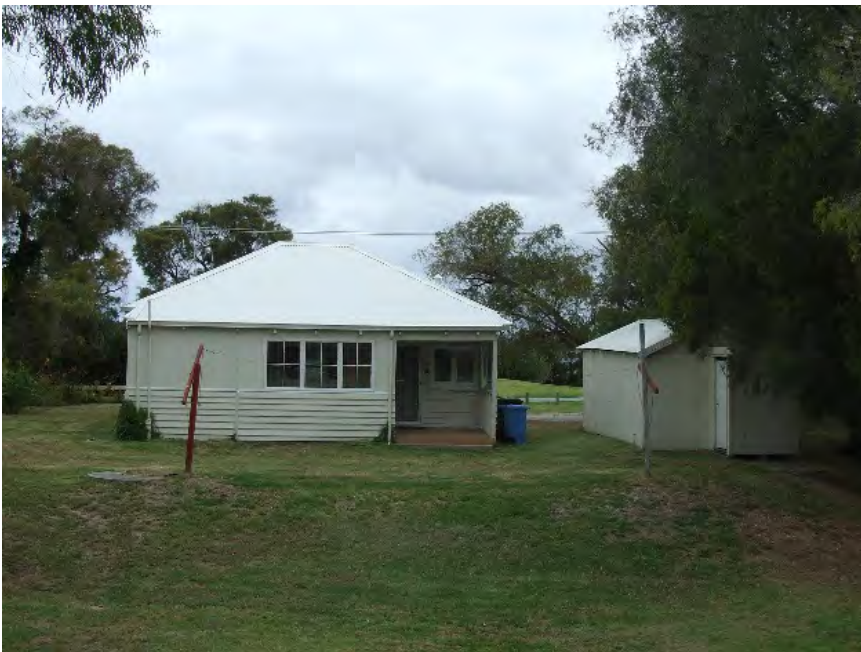
Rear elevation north [H Munt 2015]
