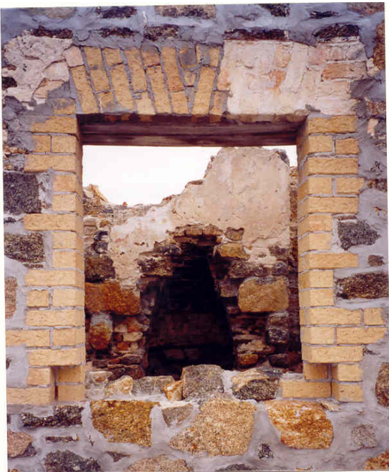
Lighthouse Keepers Cottage detail of window [Heritage Today 2000]
