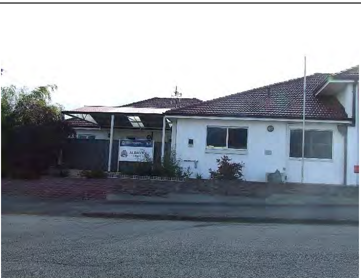
Fire Station, front (south-east) [H Munt 2016]
