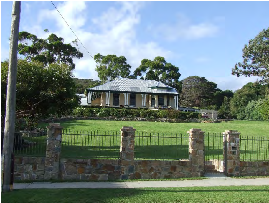
96 Brunswick Rd, front elevation (south) [H Munt 2016]
