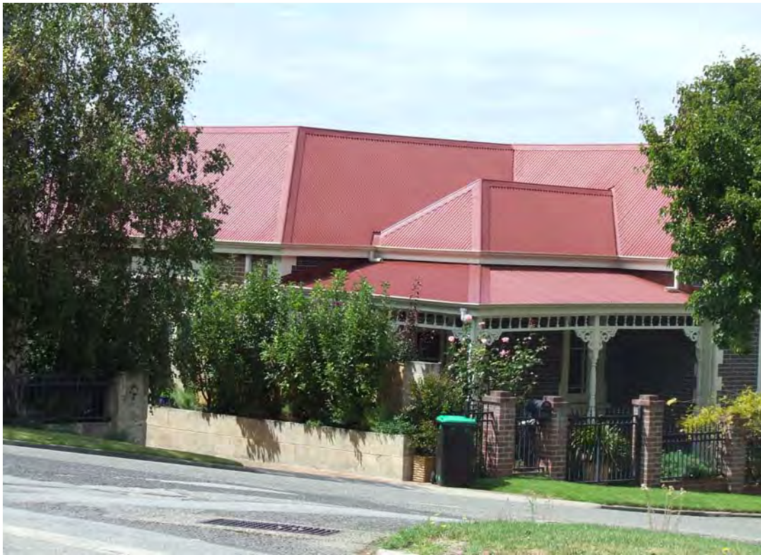
North-west elevation [H Munt 2018]
