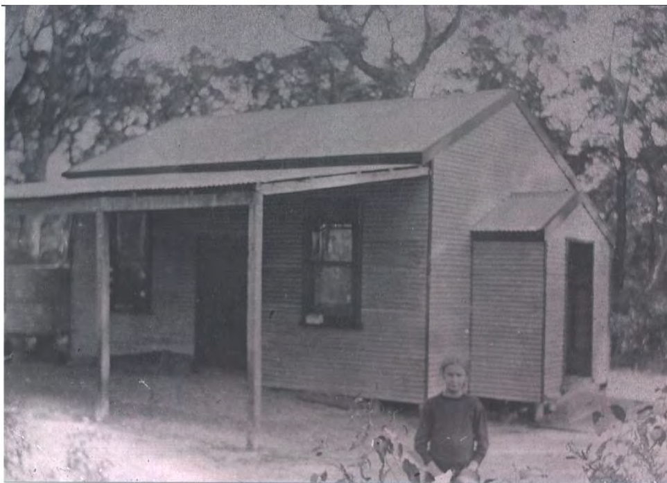
c1915 Kalgan Hall after completion of the verandah. Note the water tank at the southern end of the building and the small timber ramp leading to the porch entrance [photograph included in Conservation Plan, courtesy Chris Andrews, and Kalgan Settlers' Association]
