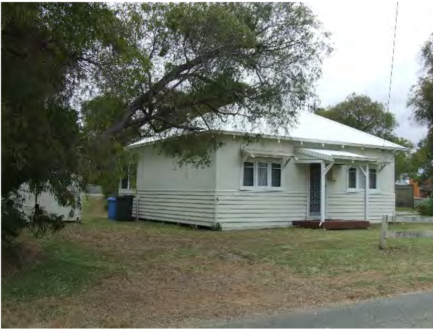
Front elevation south-west [H Munt 2015]
