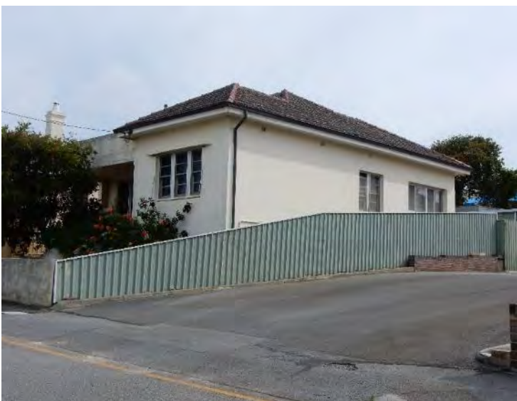
Officer's House south-east elevation [H Munt 2017]
