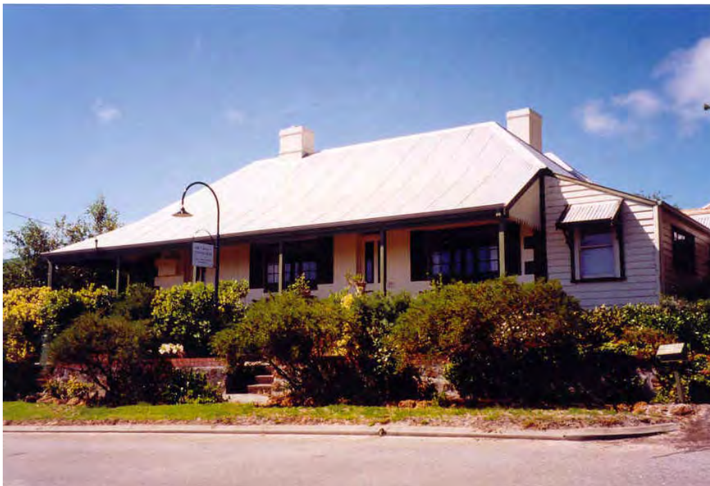
South elevation [Heritage Today 2000]
