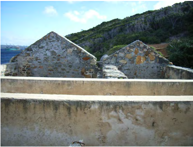
Looking over the top showing former gables and cement capping on top of wall plate [H Munt 2009]
