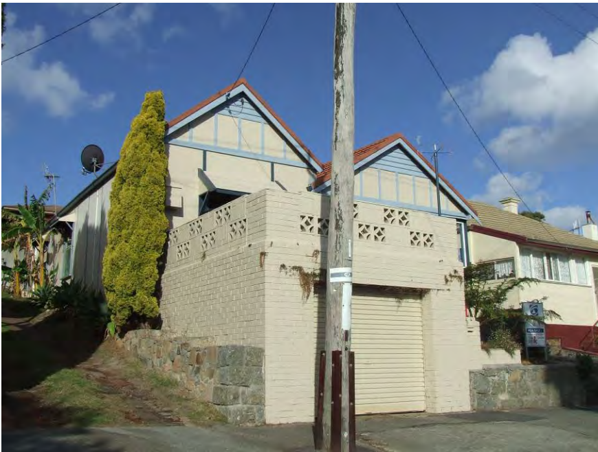
North-west elevation [H Munt 2016]
