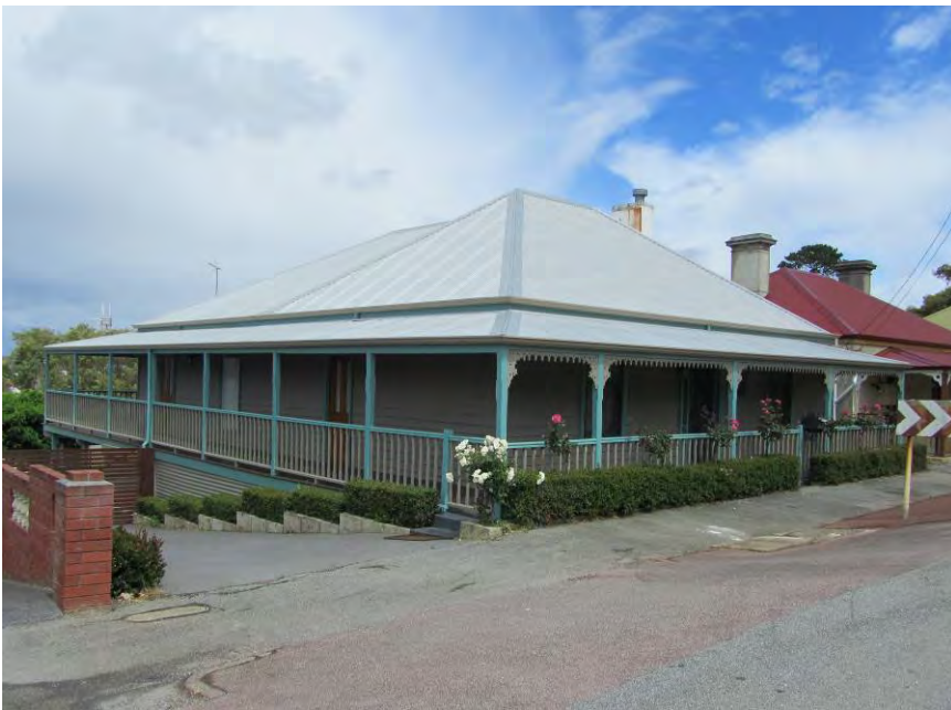
South-east elevation [H Munt 2010]
