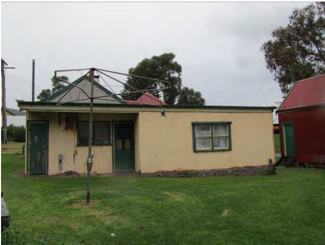
Rear elevation [H Munt 2011]
