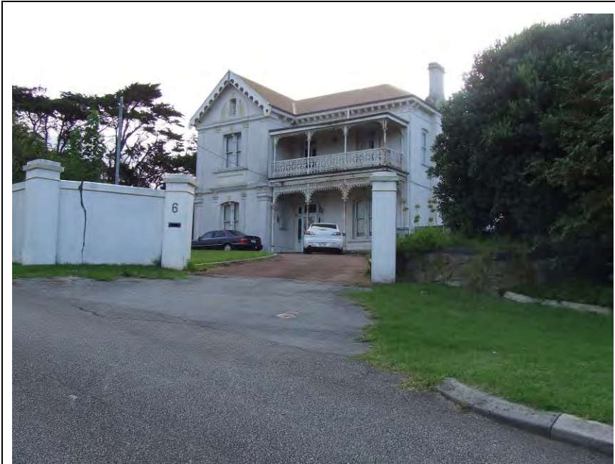
Front aspect from road [H Munt 2017]
