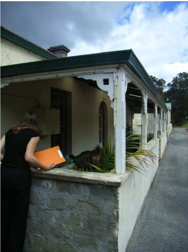
Before alterations and additions [H Munt 2007]
