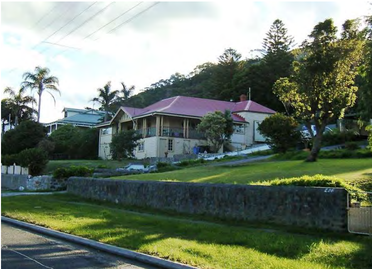
South-east elevation [H Munt 2008]
