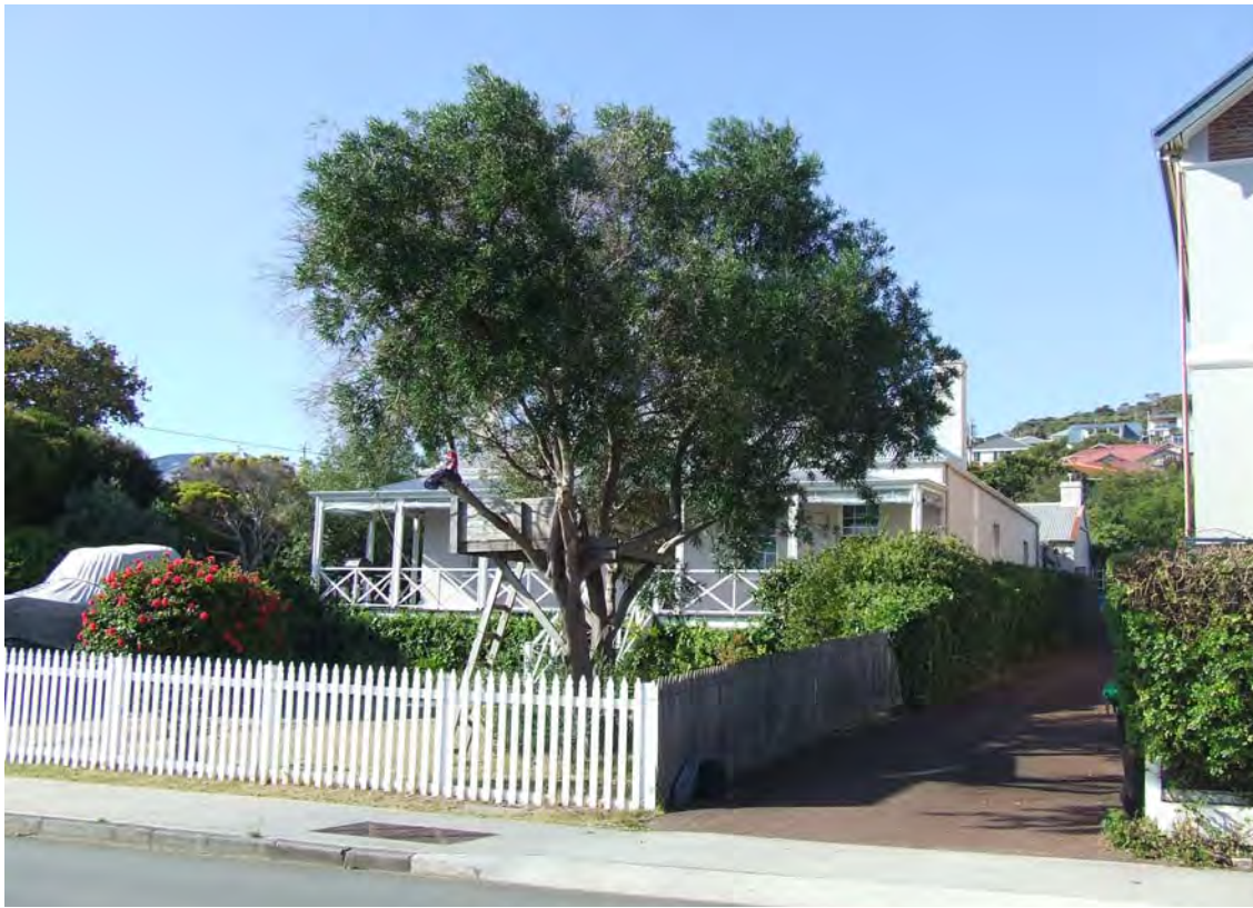
South-east elevation [H Munt 2018]
