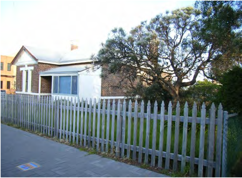
Sergeant's Quarters (fmr), 1 Duke Street, [H Munt 2010]
