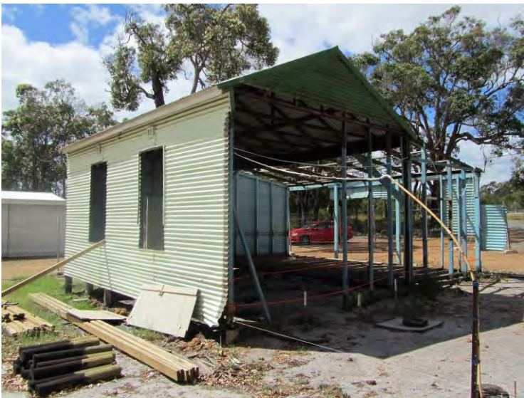
2012 demolition/reconstruction works [H Munt 2012]
