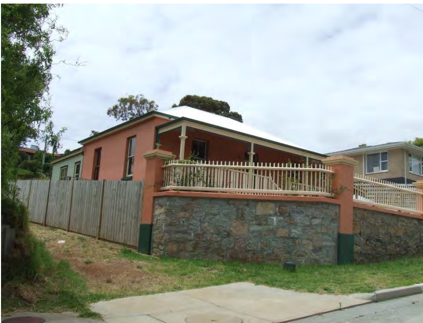
South-west elevation [H Munt 2015]
