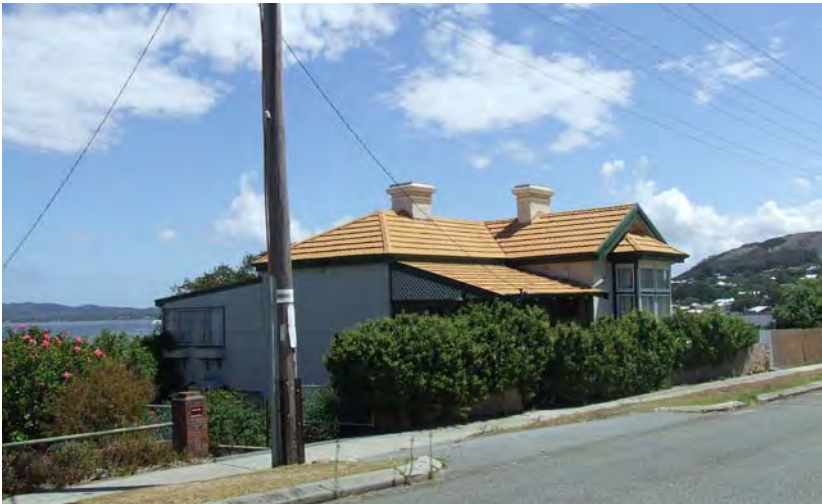
North-east elevation [H Munt 2018]
