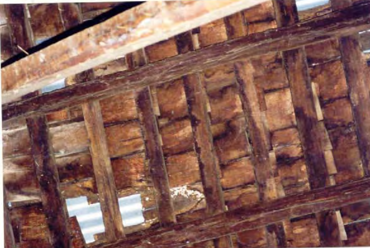
Internal view - wooden shingles under corrugated iron roof [Heritage TODAY 2000]
