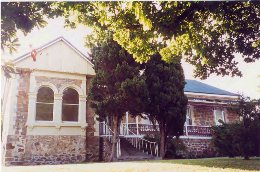
Headmaster's Quarters, east (front) elevation [Heritage Today 2000]
