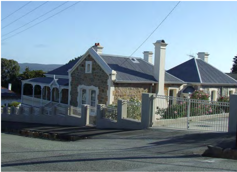
North-east elevation [H Munt 2018]
