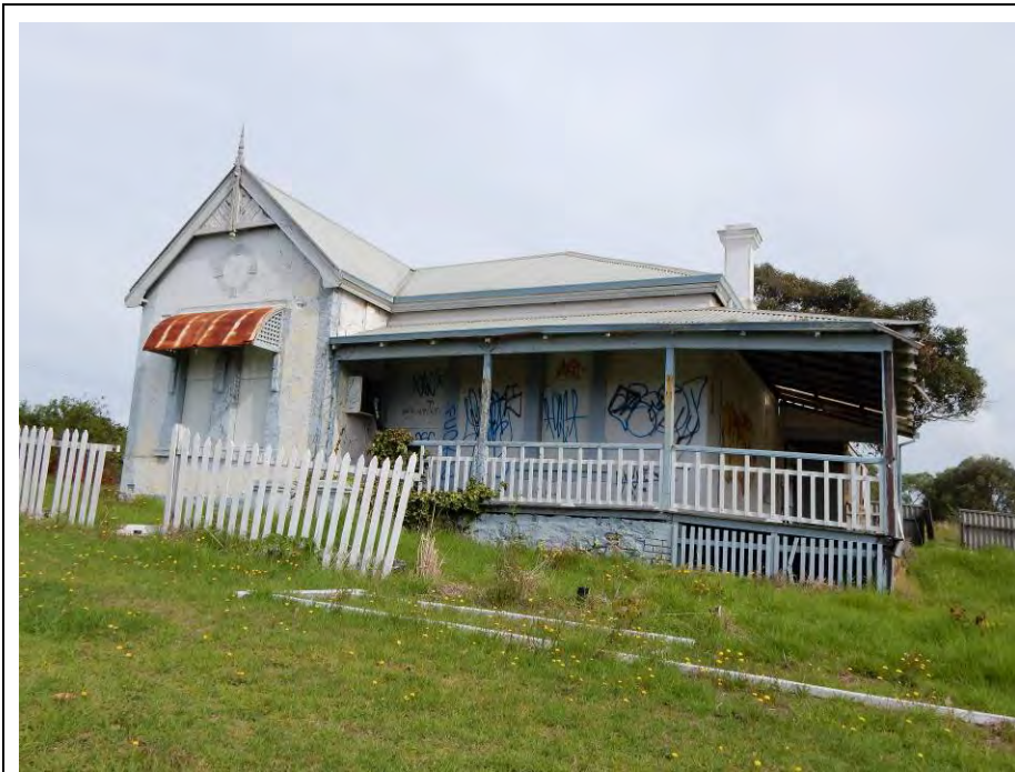
East elevation [H Munt 2017]
