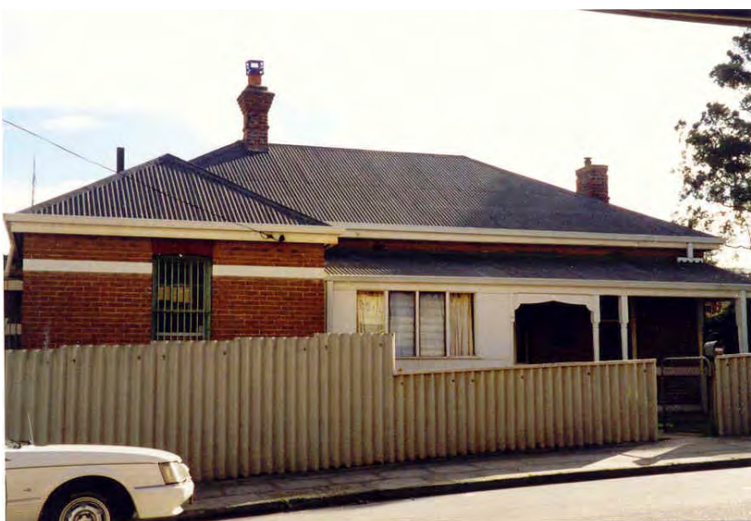
Lockup and Residence (fmr), 1 Collie Street [Heritage Today 2000]
