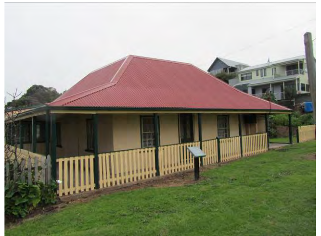
South-east elevation [H Munt 2011]
