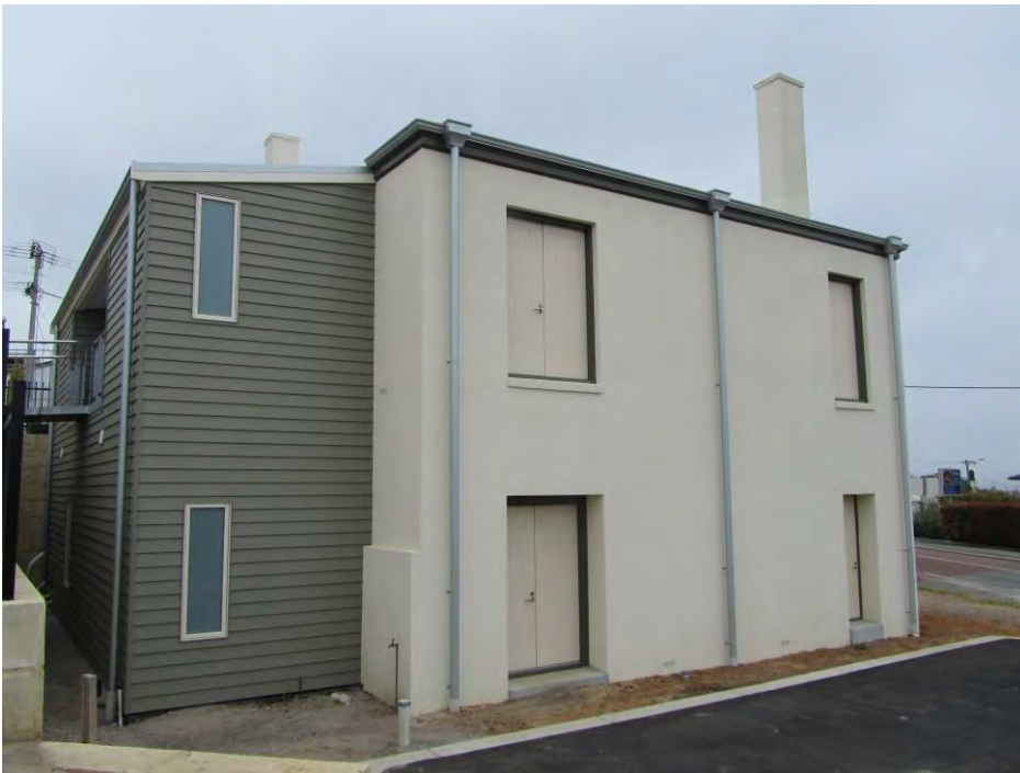
Western façade [H Munt 2017]
