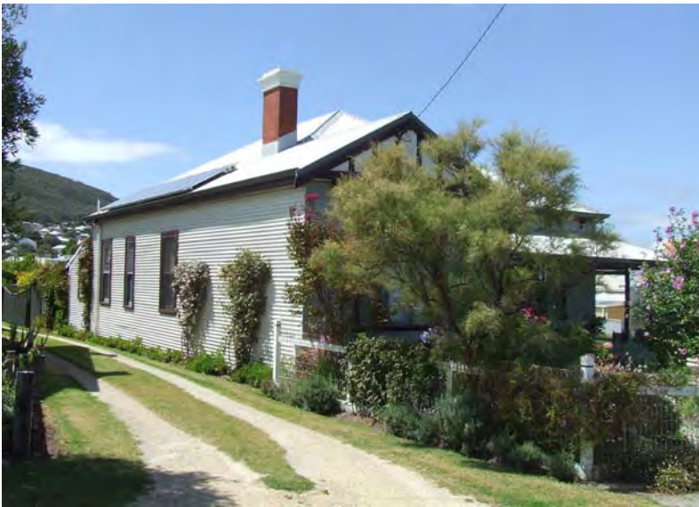
North-west elevation [H Munt 2018]
