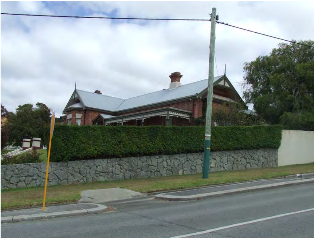
South-east elevation [H Munt 2018]
