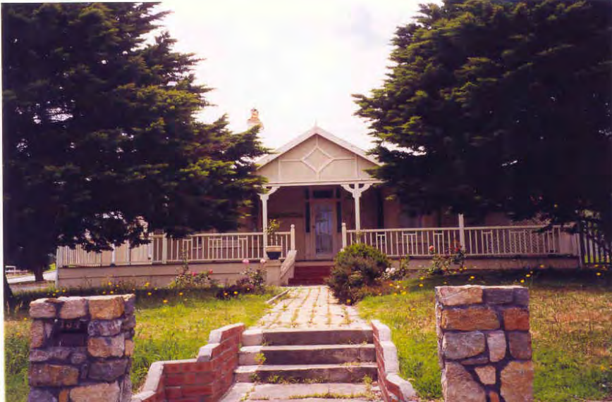
St Joseph's Lodge/New Camfield (Parish Centre) [Heritage Today 2000]
