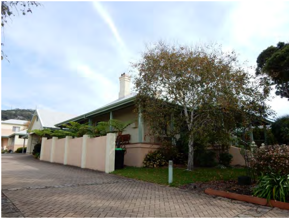
North-east elevation [H Munt 2017]
