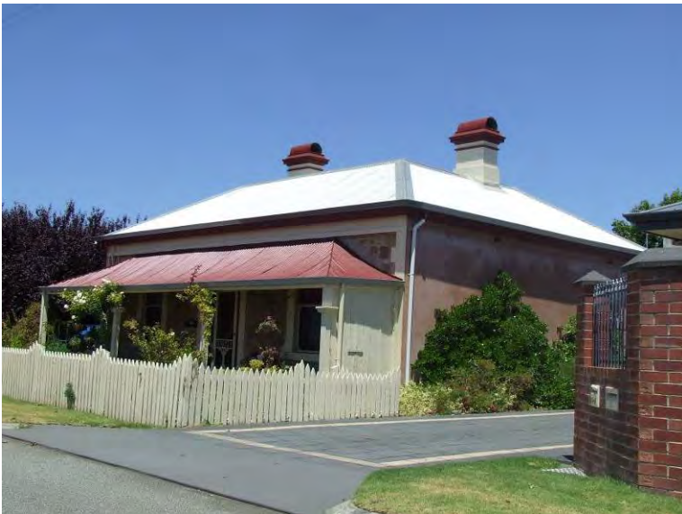
North-west elevation [H Munt 2017]
