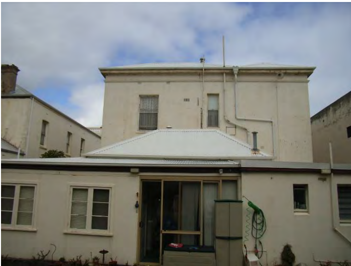
Rear elevation [H Munt 2008]
