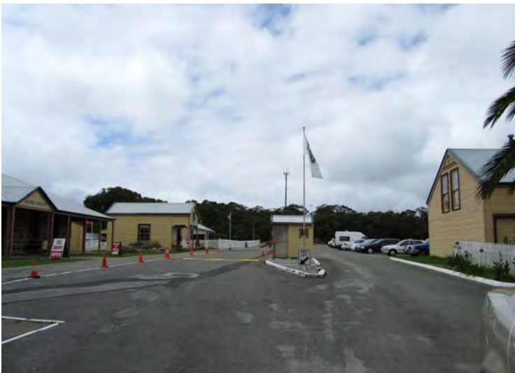
Front entry as it was in 2011 looking east [H Munt 2011]
