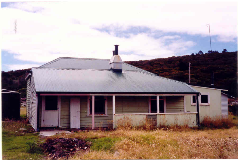
Coxwain's Quarters [Heritage Today 2000]
