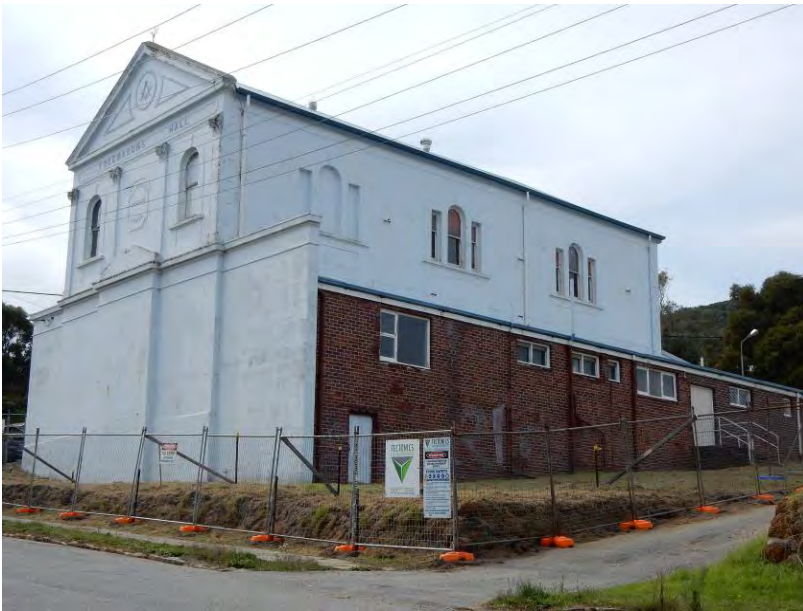
South-west elevation [H Munt 2017]
