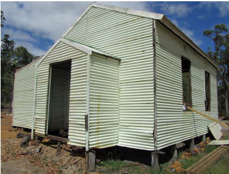
2012, just prior to demolition/reconstruction works [H Munt 2012]
