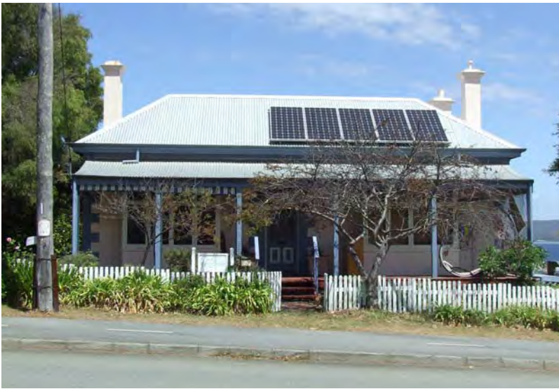
North elevation [H Munt, 2018]
