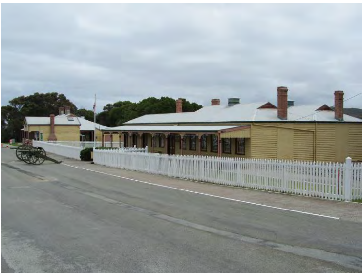
Guard House and Garrison Barracks looking west [H Munt 2011]
