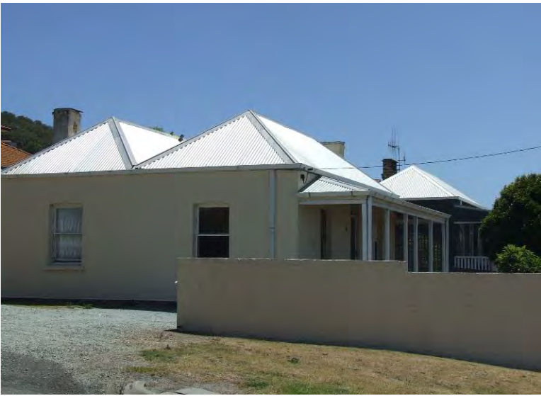
South-east elevation [H Munt 2016]
