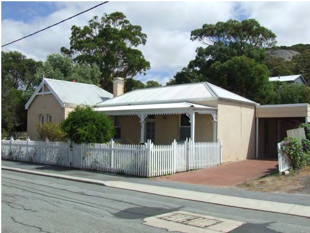
South-east elevation [H Munt 2018]
