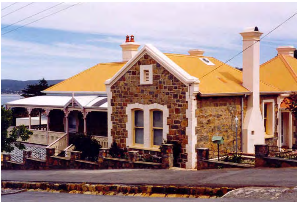
North-east elevation [Heritage Today 2000]
