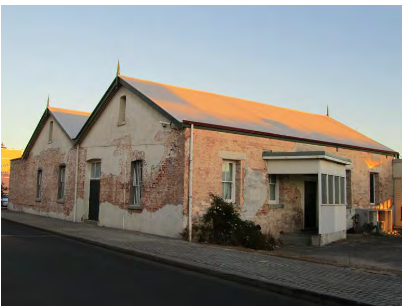
Bond store prior to conservation works [H Munt 2011]
