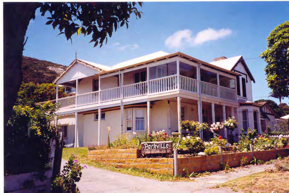
South-west elevation [Heritage Today, 2000]
