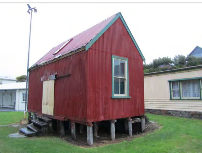
Net Shed – south-east elevation [H Munt 2011]
