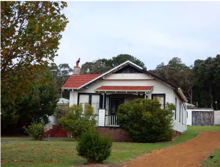
North-west elevation [H Munt 2017]
