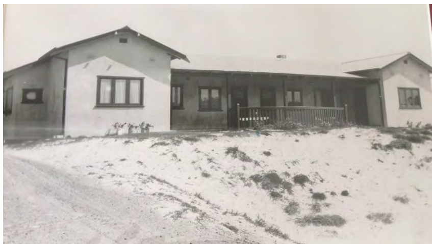
The flats just after completion, 1938 [source, CWA]
