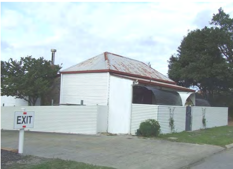
South-east elevation [H Munt 2017]
