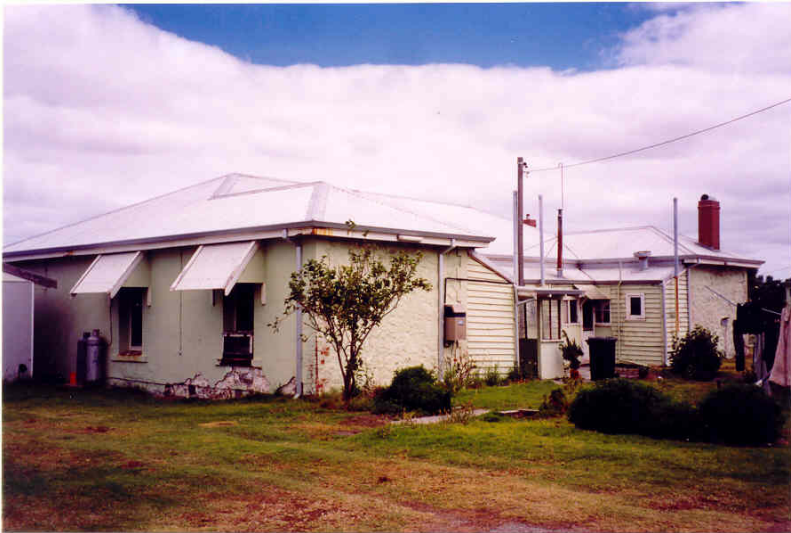
Pilot Crew Quarters, front view, facing the ocean [Heritage Today 2000]
