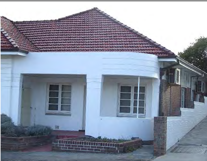
Fire Station, front (north-east) [H Munt 2016]
