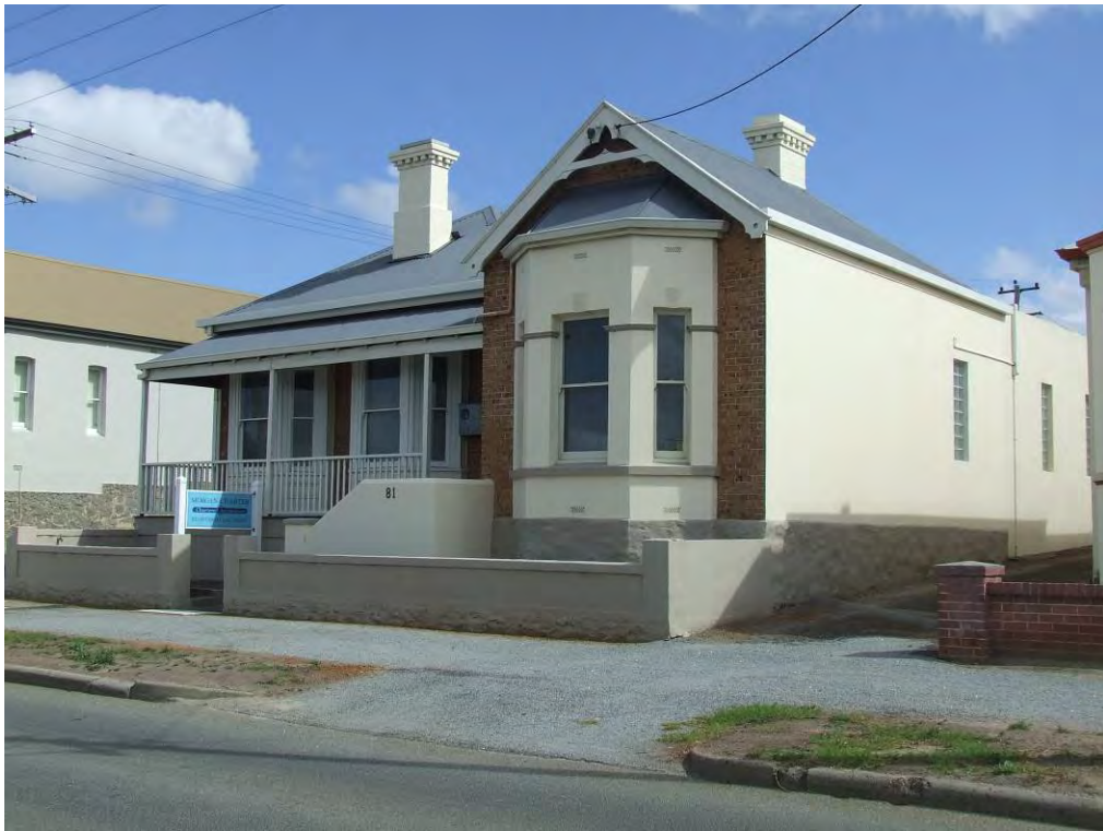
North-east elevation [H Munt 2016]
