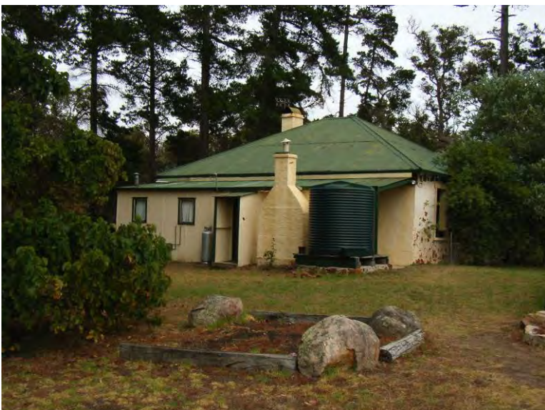
Rear elevation [H Munt 2009]
