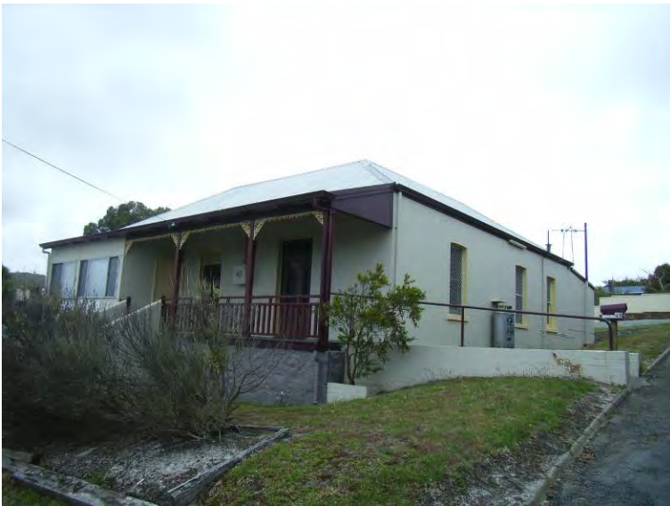
South-east elevation [H Munt 2008]
