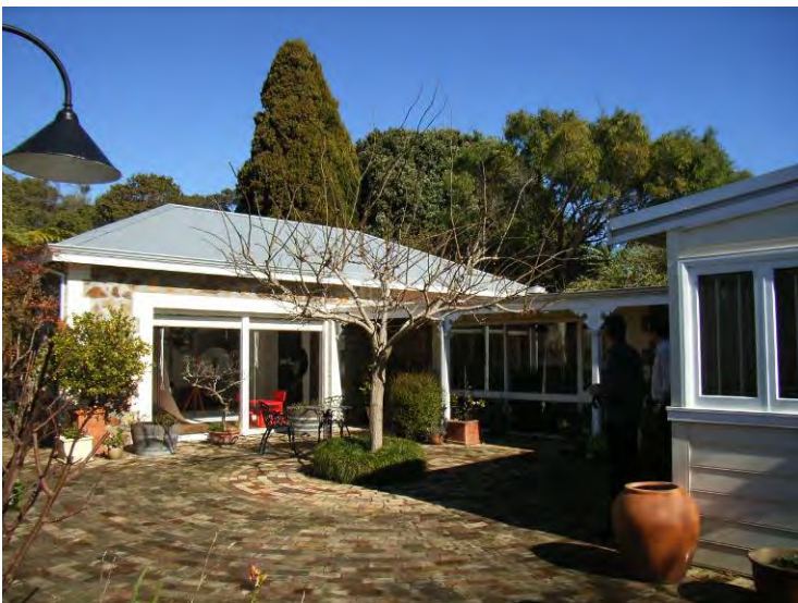
Rear showing link and addition [H Munt 2009]
