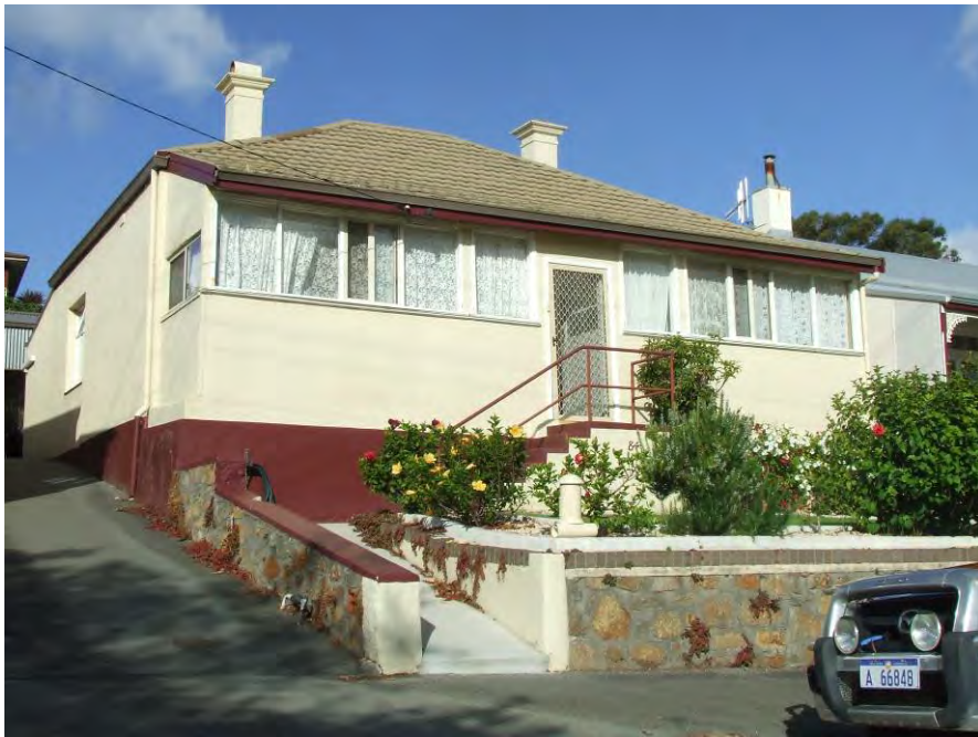
North-west elevation [H Munt 2016]
