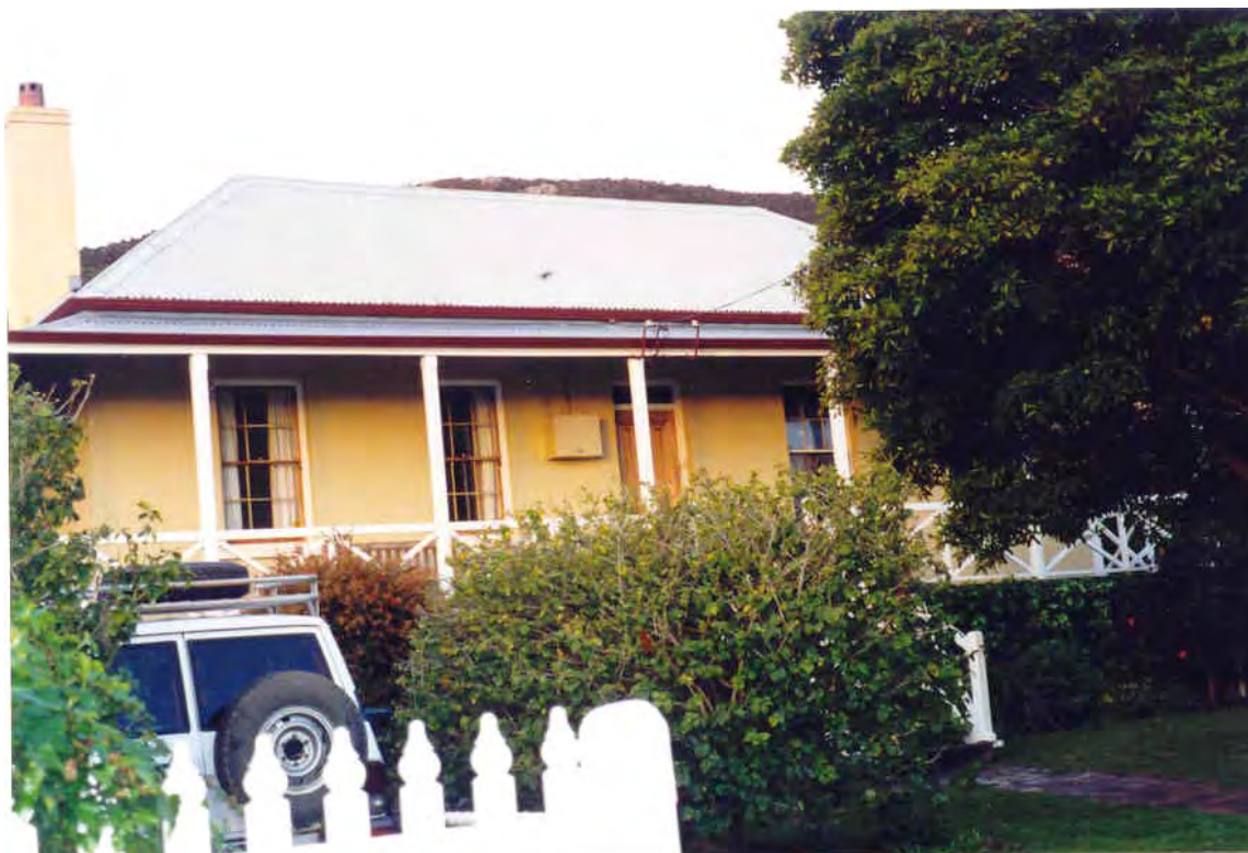
South (front) elevation [Heritage Today 2000]
