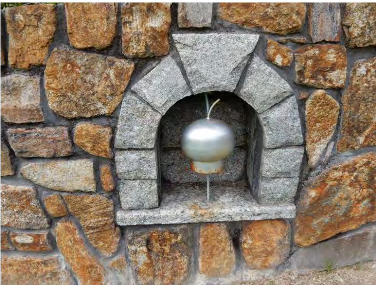
Detail of sculptural inserts into waterfall retaining wall [H Munt 2017]
