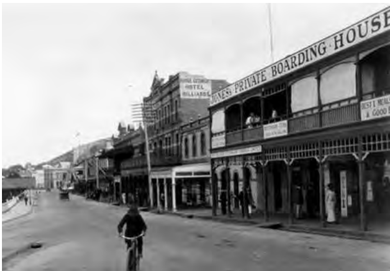
1915 showing double storey timber verandah [SLWA 0531D]
