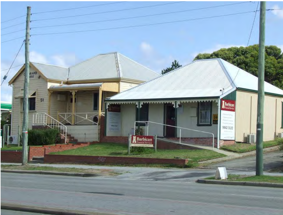
North-east elevation [H Munt 2017]
