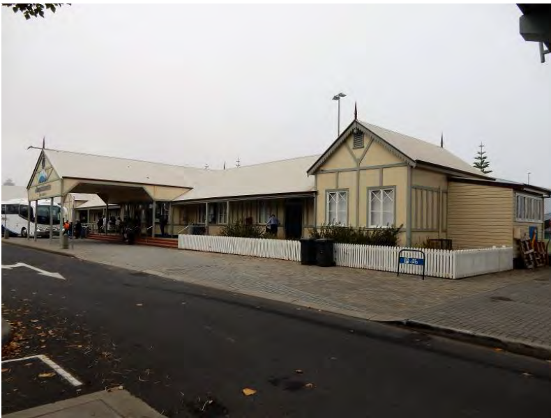
Railway Station north elevation [H Munt 2017]
