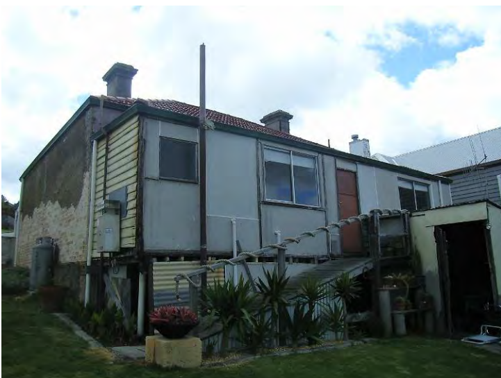
Before alterations and additions [H Munt 2007]
