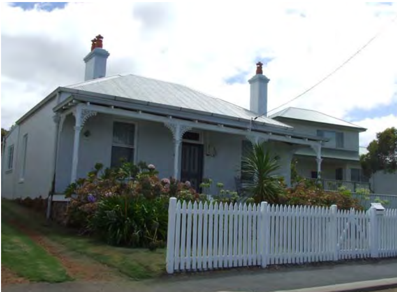
South-west elevation [H Munt 2018]
