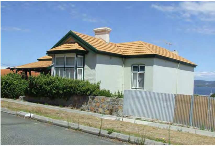
North-west elevation [H Munt 2018]
