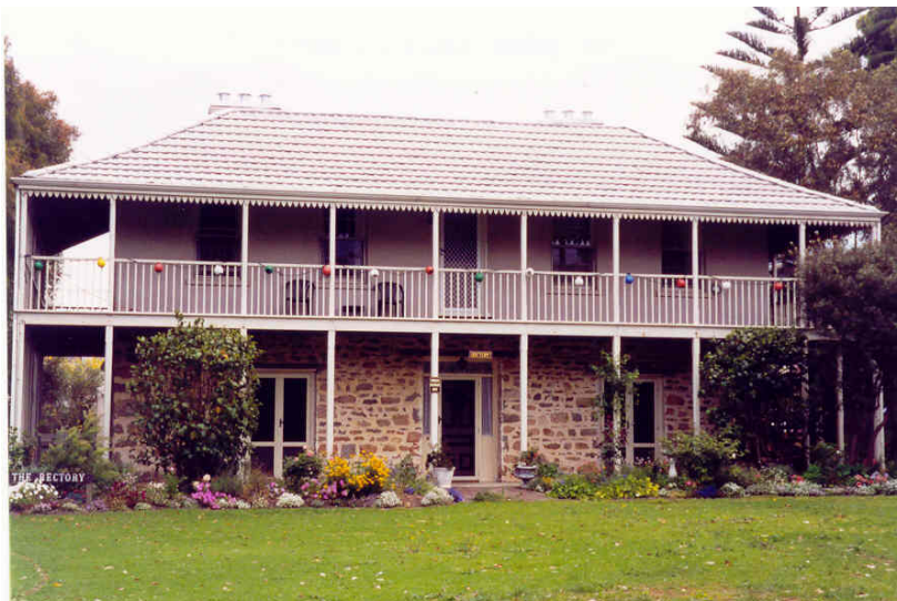
The Rectory [Heritage Today 2000]
