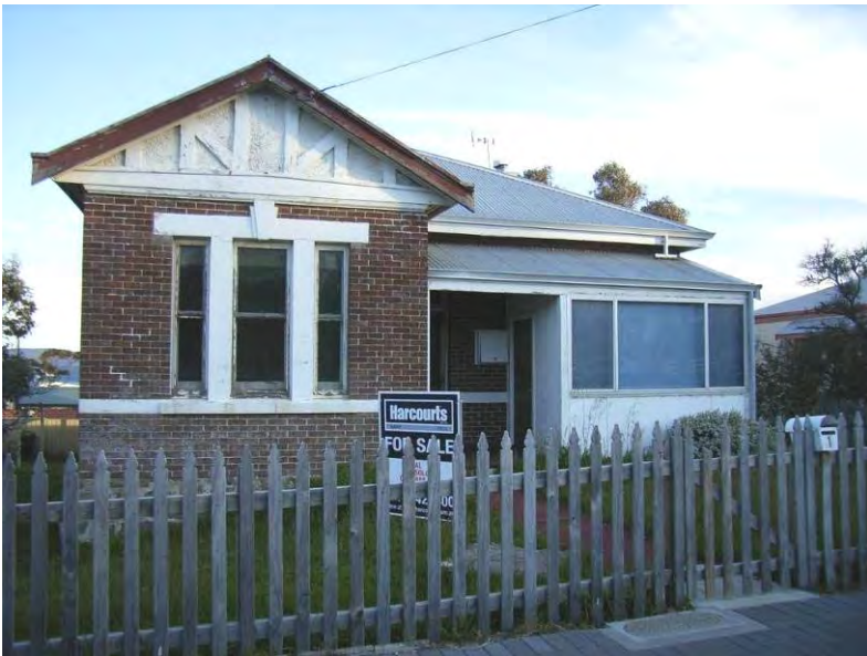
Sergeant's Quarters (fmr) – 1 Duke Street [H Munt 2010]
