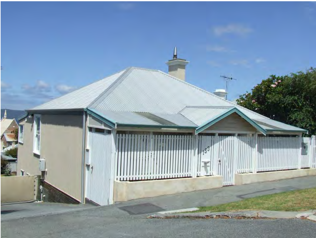
North-west elevation [H Munt 2018]
