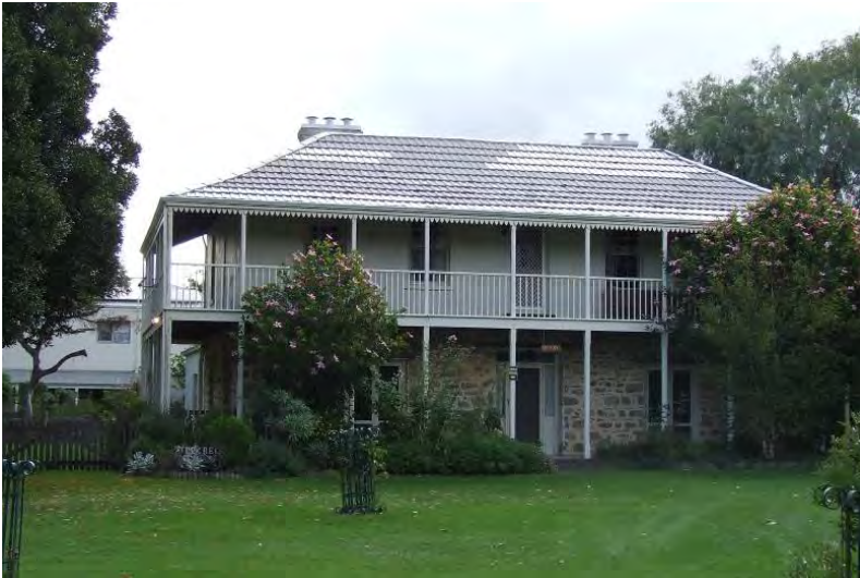
The Rectory front elevation (east) [H Munt 2017]
