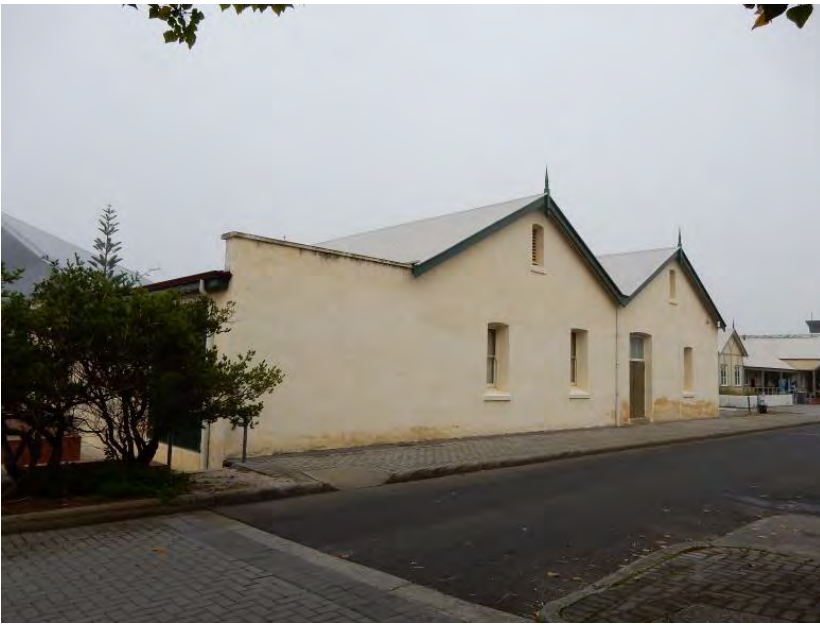
Railway Station Bond Store north elevation [H Munt 2017]
