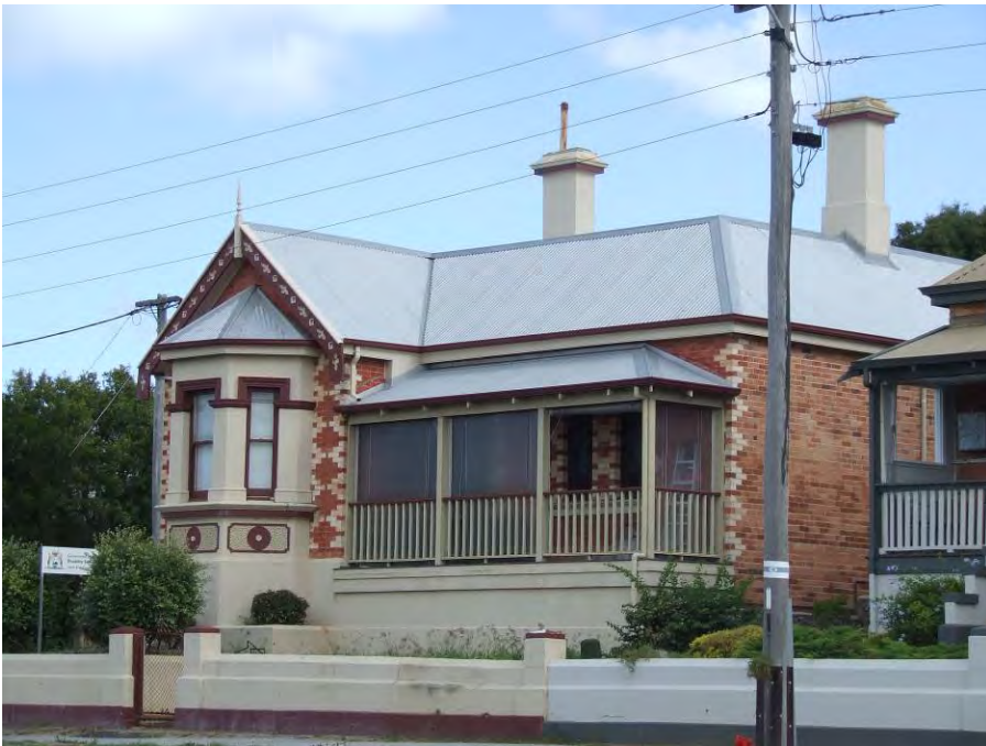
North-east elevation [H Munt 2016]
