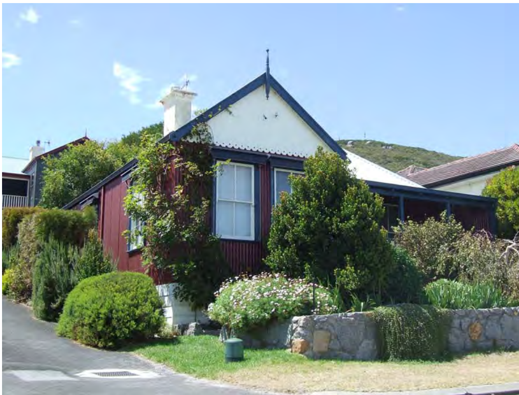
South-west elevation – note the change to external cladding, apron cladding and front window [H Munt 2018]
