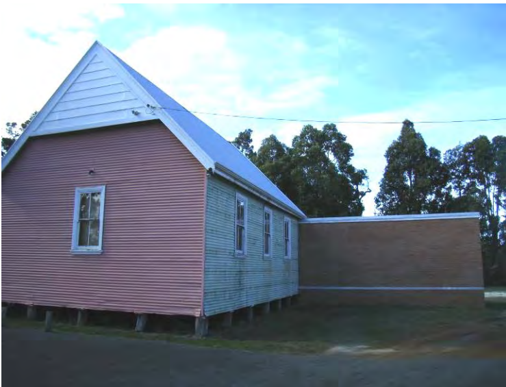
Side and rear elevation [H Munt 2007]
