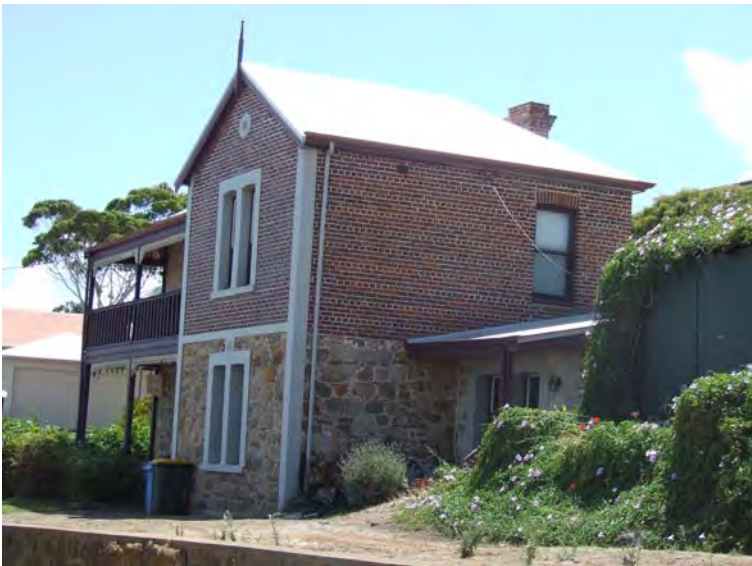
South-east elevation [H Munt 2018]
