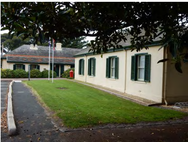
Residency - north and north-west elevation [H Munt 2017]
