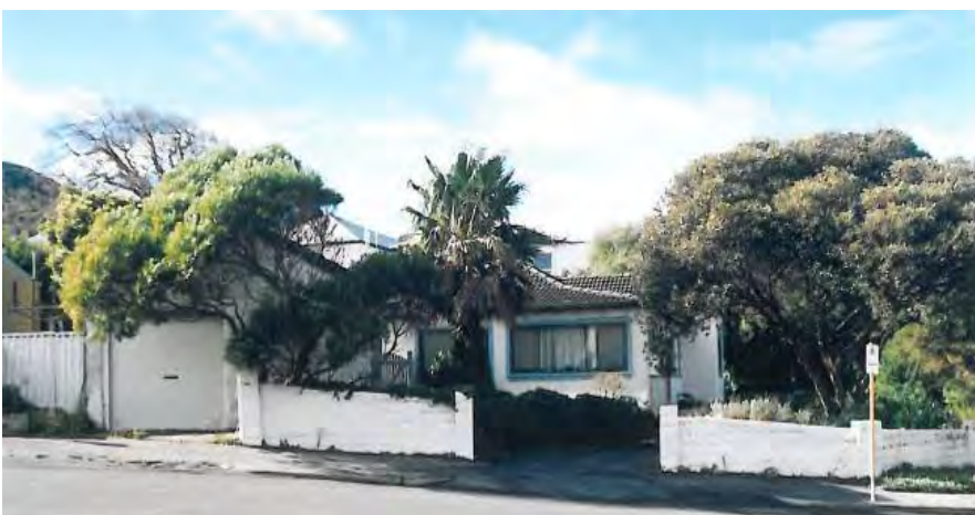
2000, west elevation from Spencer St [Considine and Griffiths, Stirling Tce Conservation Plan, 2000]
