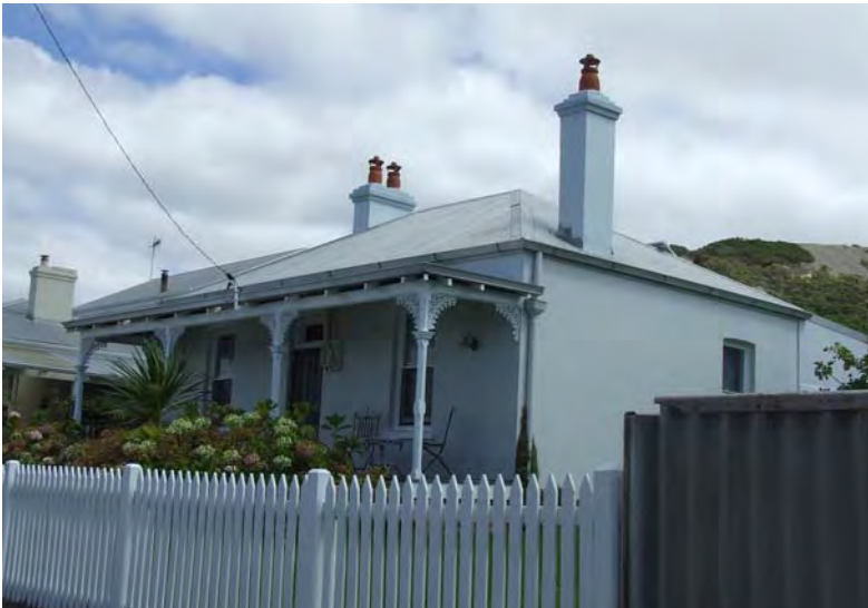
South-east elevation [H Munt 2018]
