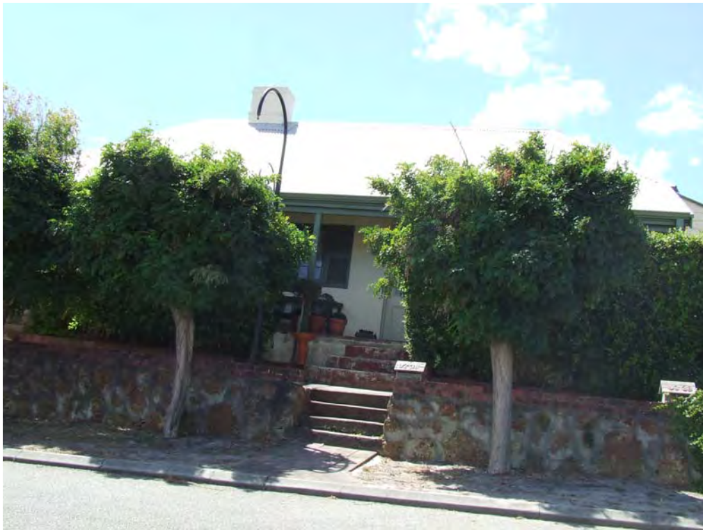
South (front) elevation [H Munt 2018]
