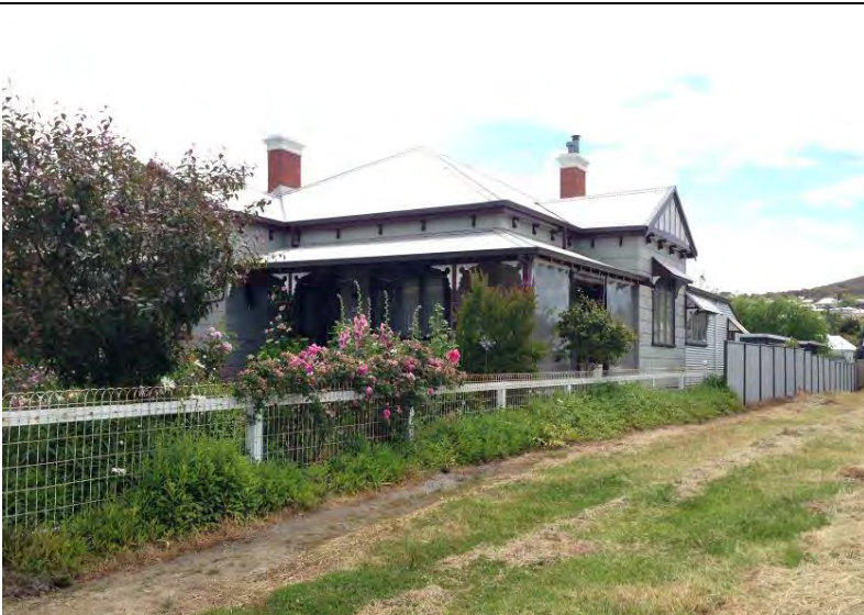
South-west elevation [H Munt 2016]
