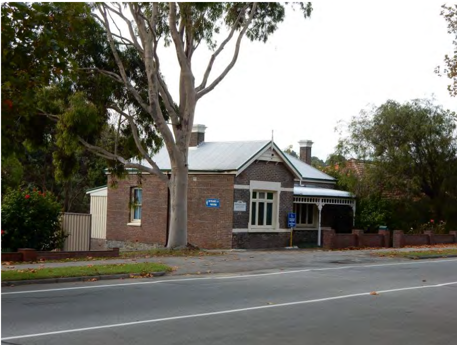
South-west elevation [H Munt 2017]
