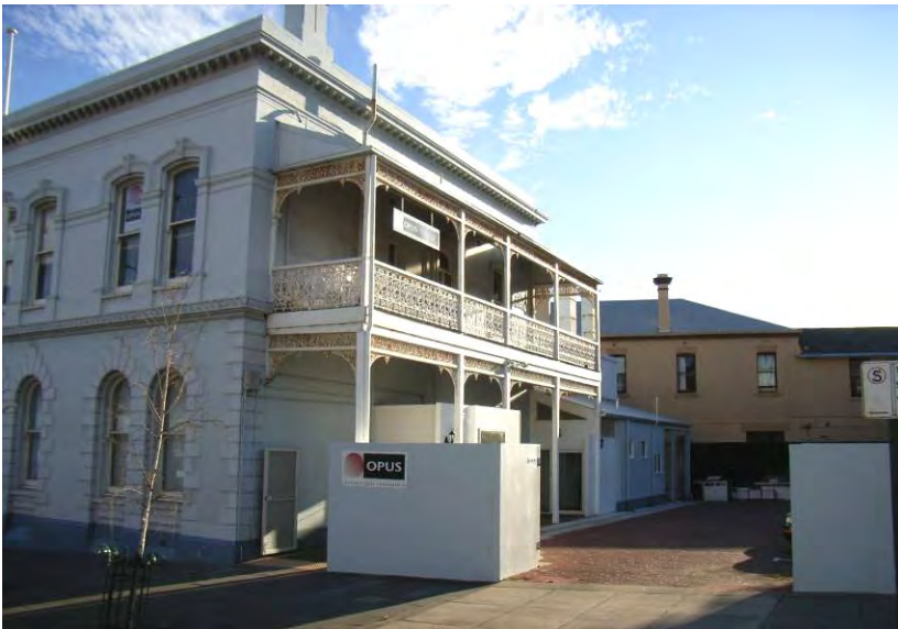
Albany House, rear view after alterations [H Munt, 2008]
