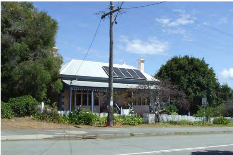
North-east elevation [H Munt, 2018]
