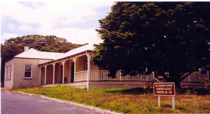
St Joseph's Lodge/New Camfield (Parish Centre) [Heritage Today 2000]
