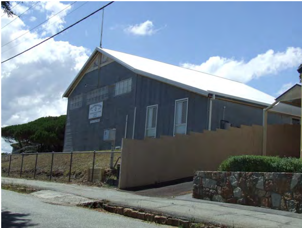
South-west elevation from Spencer Street [H Munt 2018]
