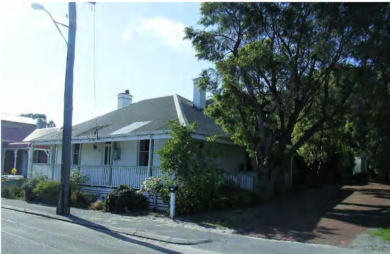
South-east elevation [H Munt 2008]
