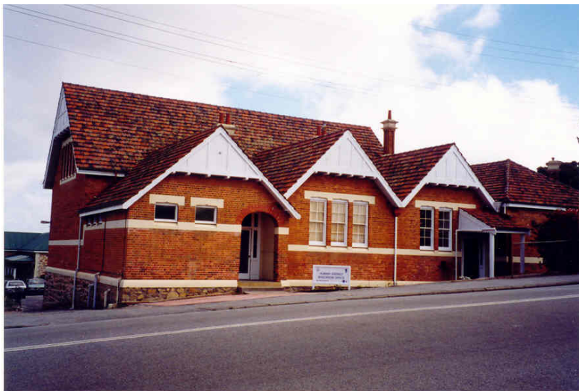
Building 1 [Heritage Today 2000]
