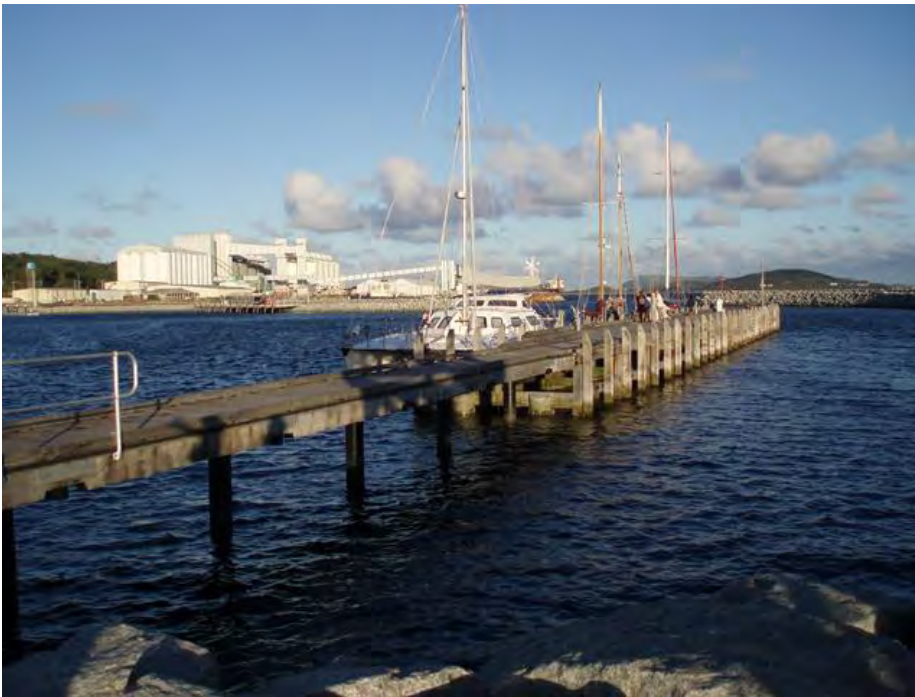
2011, after foreshore development, south east arm [State Heritage Office]
