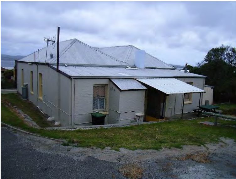
Rear (north) elevation [H Munt 2008]
