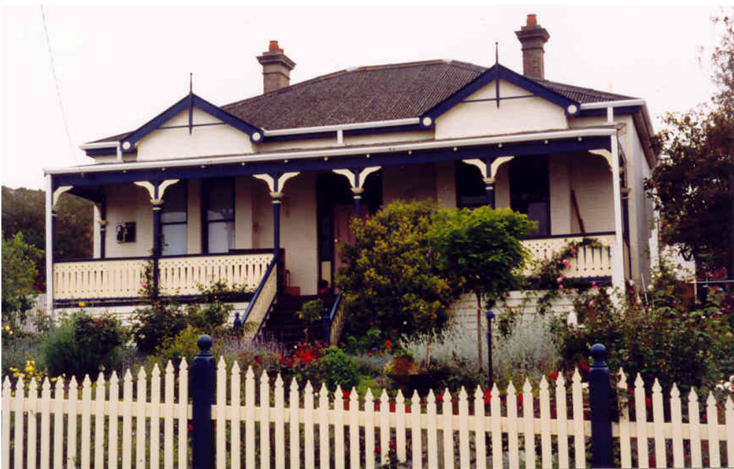
South (front) elevation [Heritage Today 2000]
