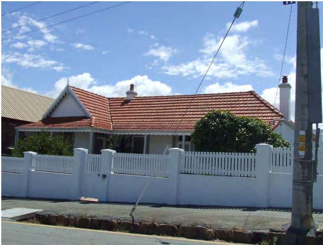
South-east elevation [H Munt 2018]
