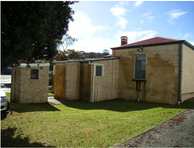
Rear elevation [H Munt 2008]
