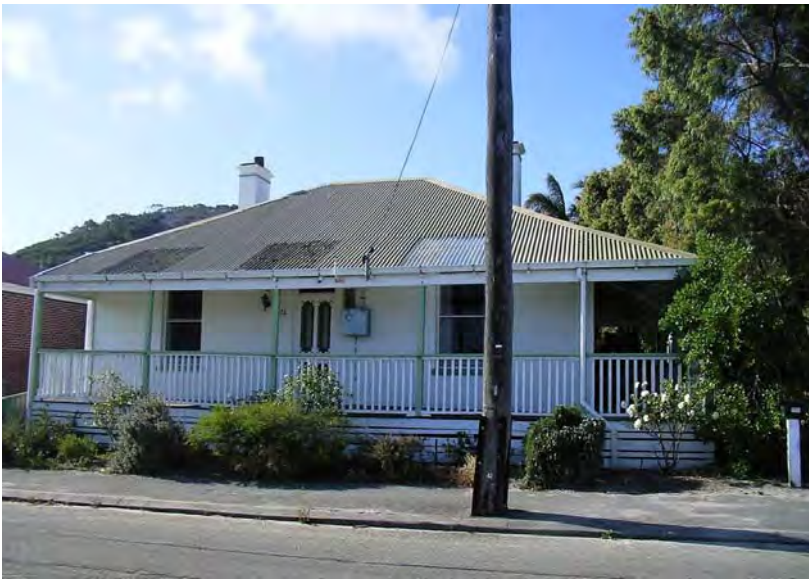
South (front) elevation [H Munt 2008]
