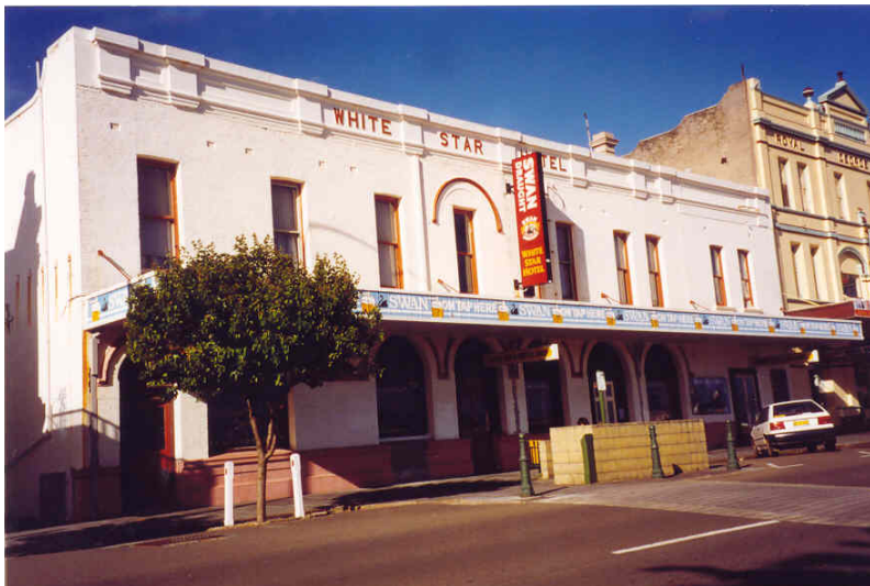
Showing the former cantilevered awning removed c2014 [Heritage Today 2000]
