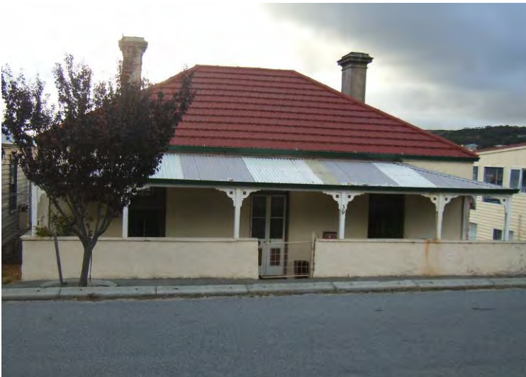
Before alterations and additions note decromastic tiles and front wall [H Munt 2007]
