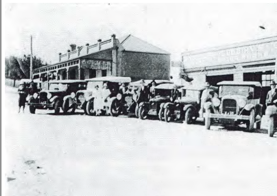
c1920 showing the original skillion verandah on the warehouse and unpainted facebrick to the side elevation [Albany Historical Society]
