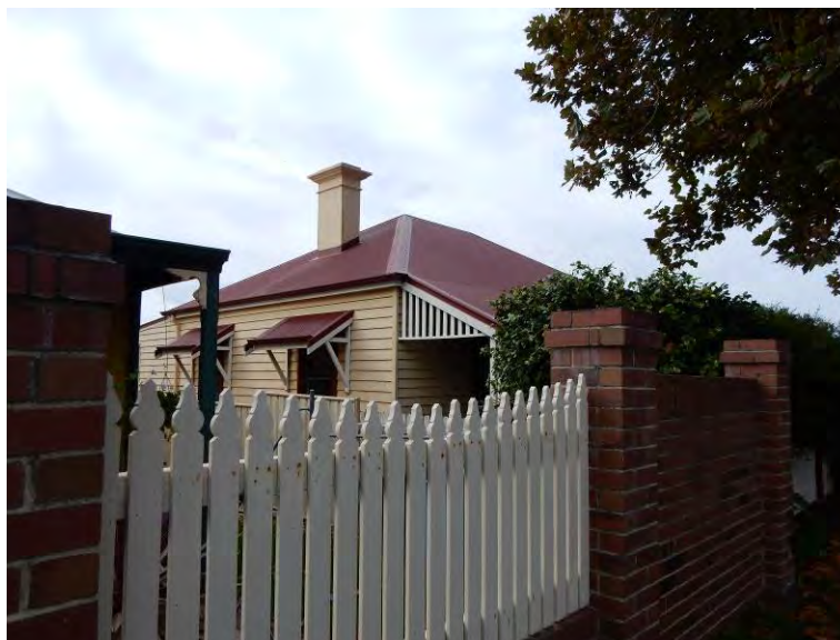
South-west elevation [H Munt 2017]
