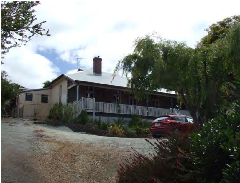
South-west elevation [H Munt 2018]
