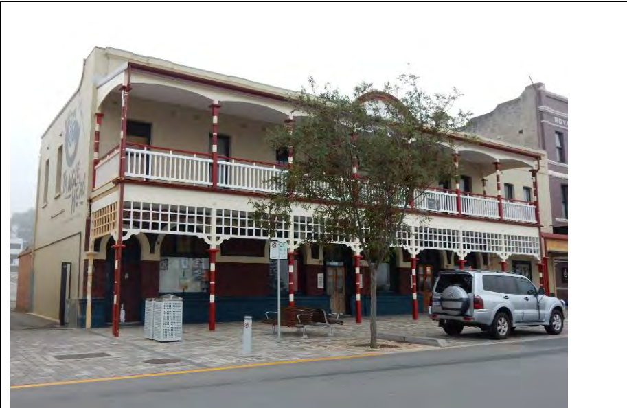
With the reconstructed 1910 two storey verandah added 2016 [H Munt 2017]
