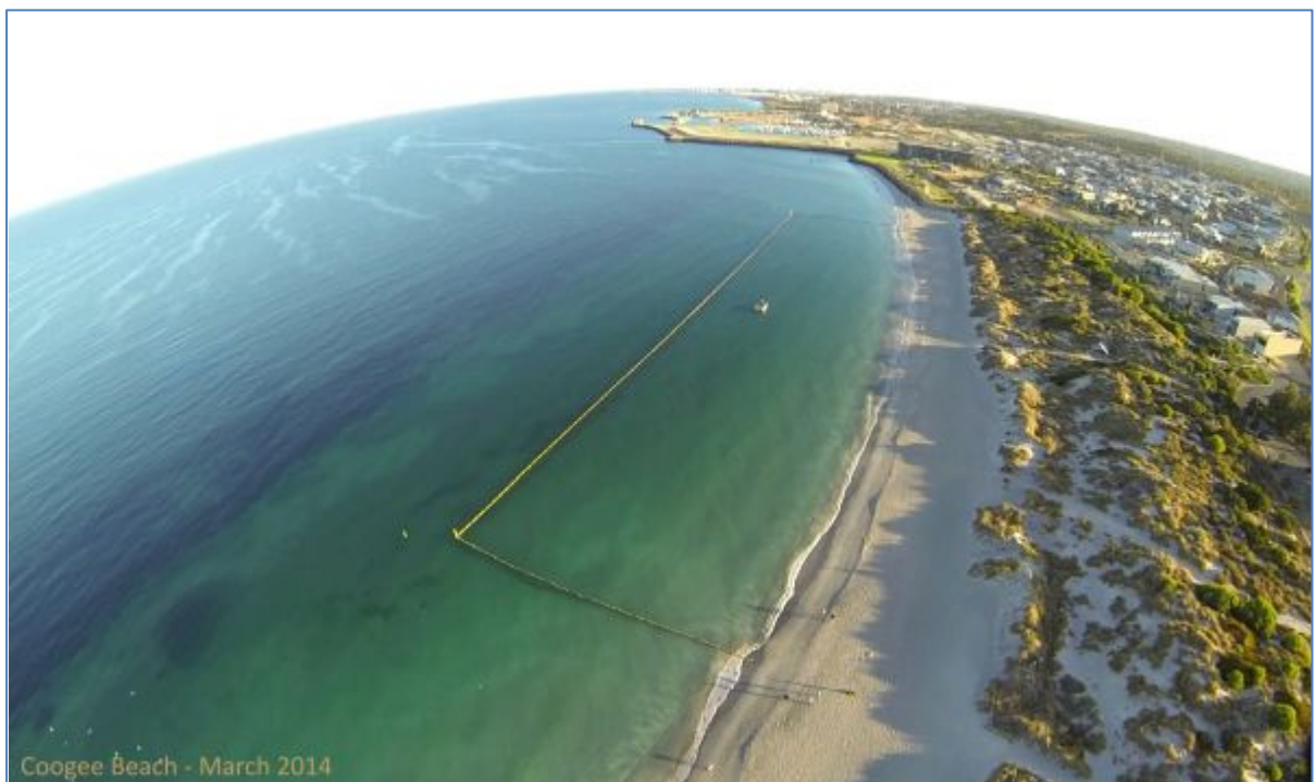
Image 1 – Eco Shark Barrier installed at Coogee Beach March 2014
