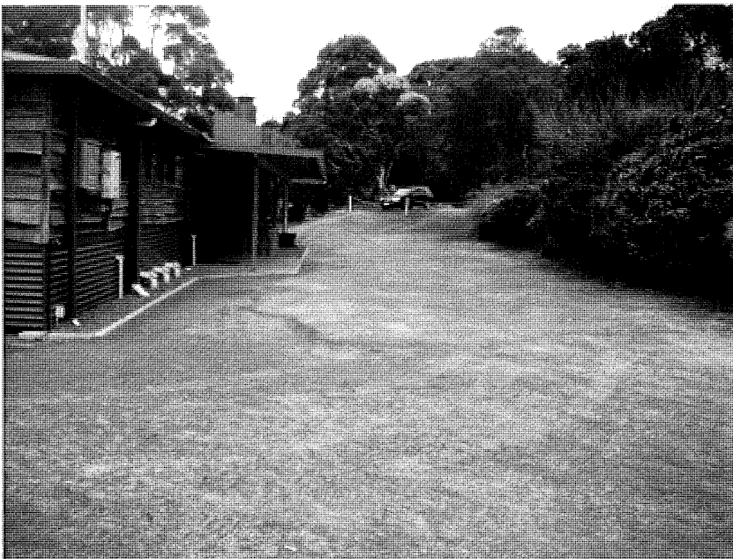
The drive entry to the function centre. There is room for dropping off of patrons in the LHS at the foreground, with sufficient paved width for continuing one way access available on the RHS.
