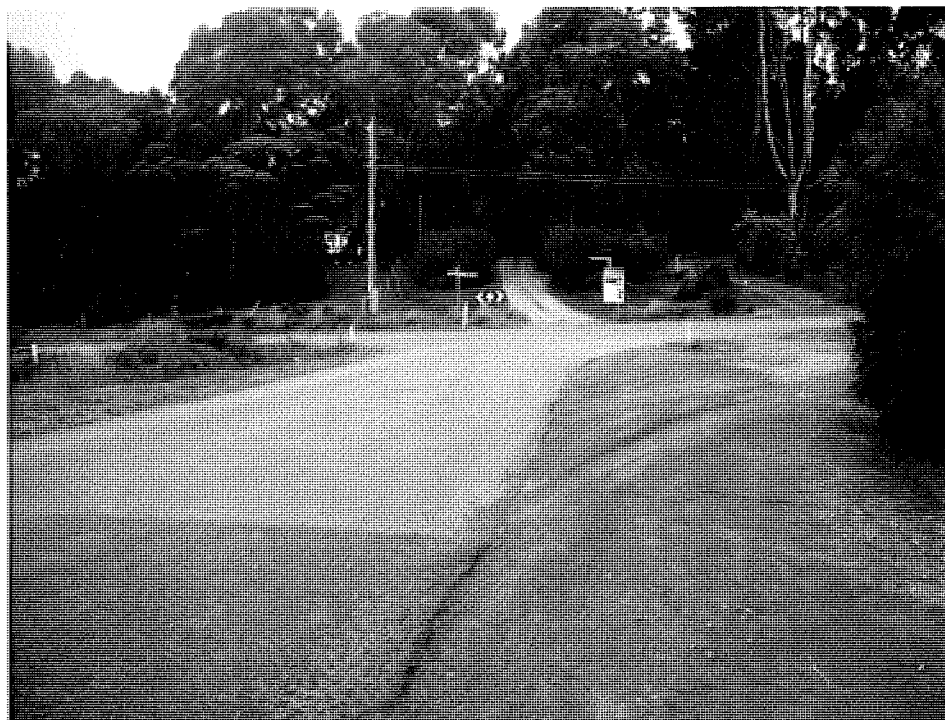
The view from the extremity of the proposed EXIT turn-outs towards the intersection with Coombes Road. Removal of the vegetation to the right would improve the visibility from the exit. IT IS STRONGLY RECOMMENDED THAT THE CITY INSTALL A STREETLIGHT ON THE POLE AT THE INTERSECTION IN ORDER TO ILLUMINATE IT, REINFORCE THE 60KM/HR SPEED LIMIT AT NIGHT, AND TO PROVIDE ADDITIONAL NIGHT WARNING OF THE INTERSECTION FROM OVER THE COOMBES Rd APPROACH CREST.
