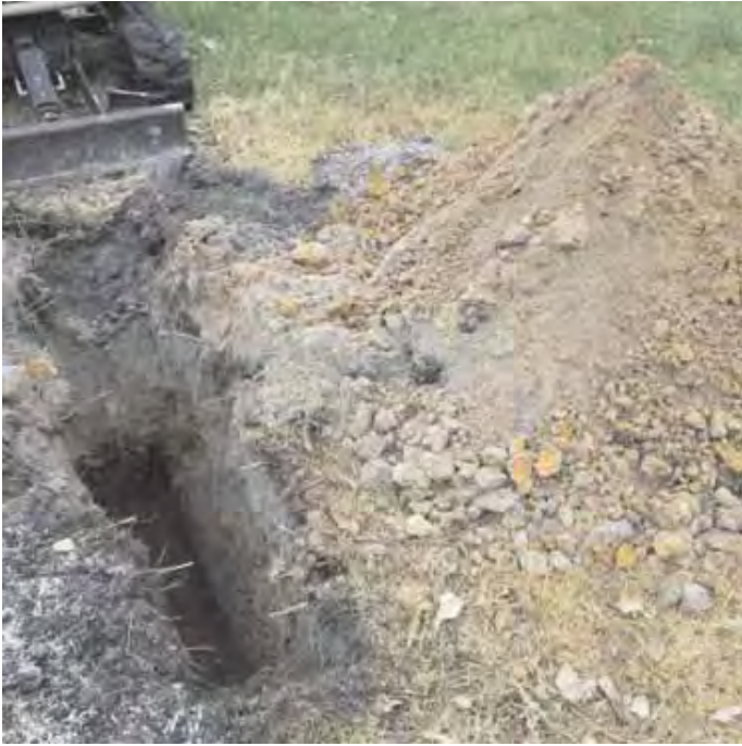
Test Hole on Lot 13
