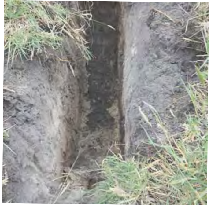
Test Hole on Lot 10
