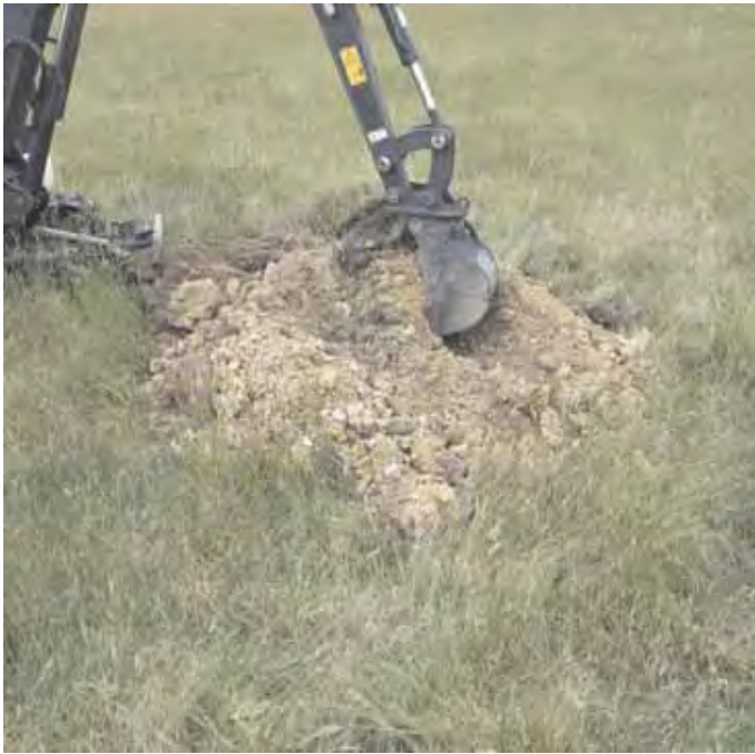
Test Hole on Lot 17
