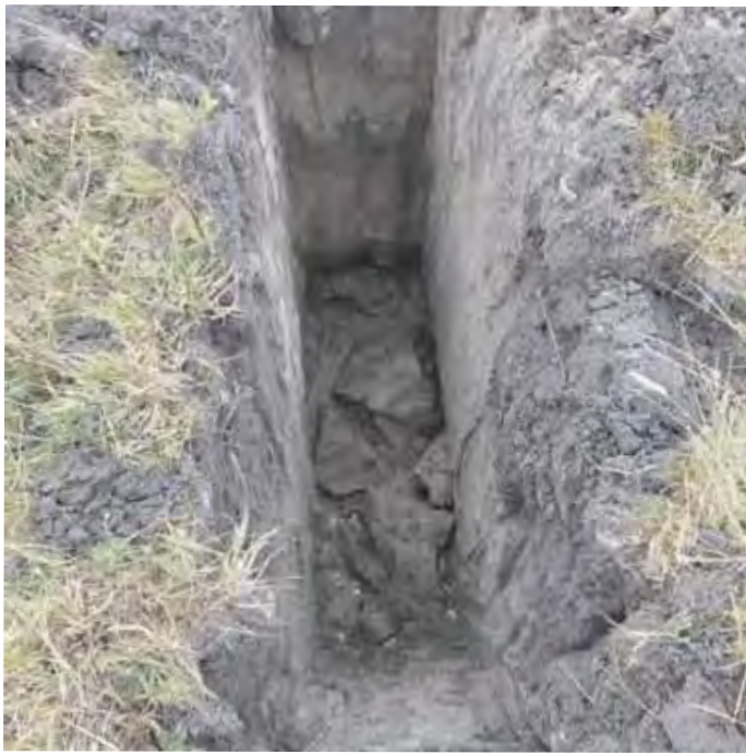
Test Hole on Lot 4
