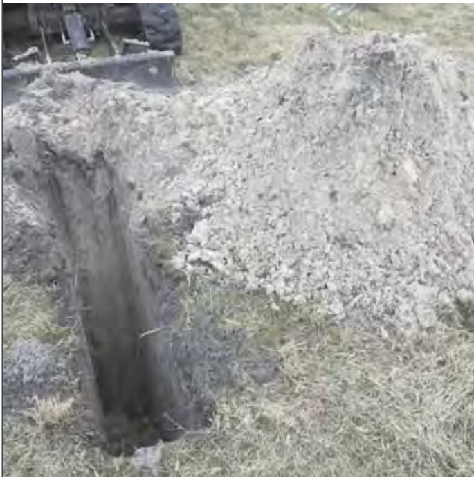
Test Hole on Lot 18
