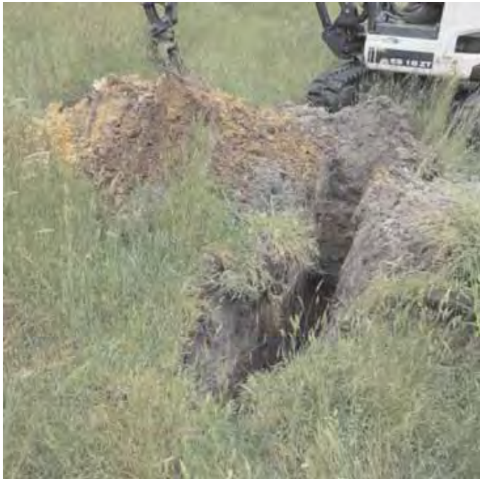
Test Hole on Lot 14
