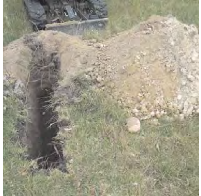
Test Hole on Lot 12
