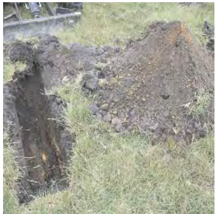
Test Hole on Lot 16
