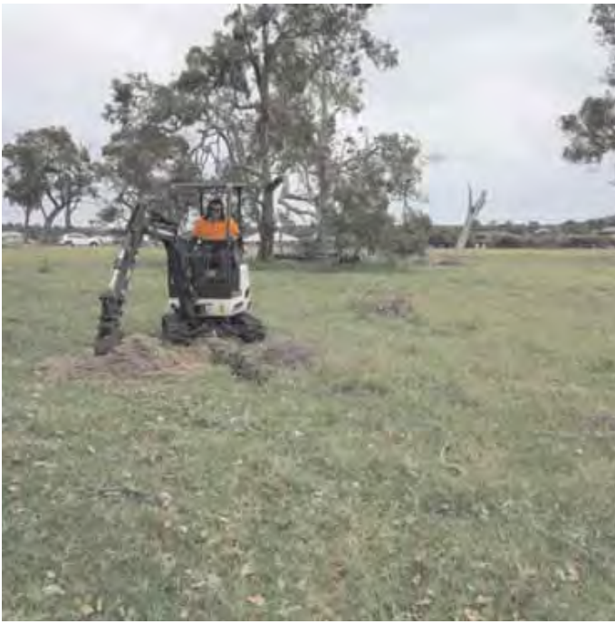
Test Hole on Lot 1
