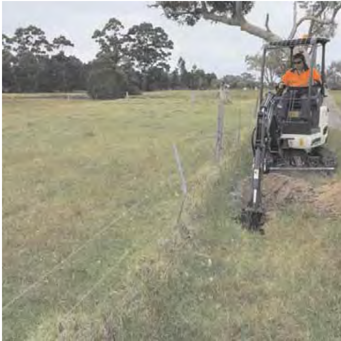
Test Hole on Lot 6
