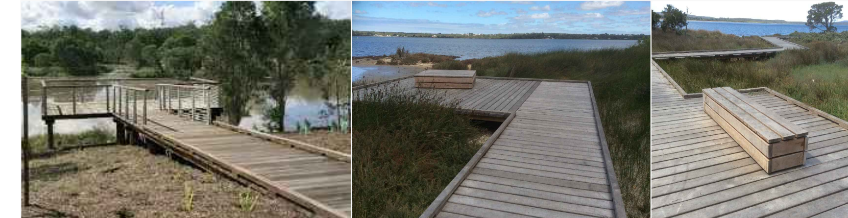
TIMBER DECKED VIEWING PLATFORM WITH TIMBER SEAT AND A TIMBER BOARD WALK FORMING THE TRANSITION TO NEW LIMESTONE PATHWAY
