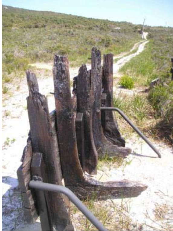
Restored section of Elvie showing jarrah planks and ribs
