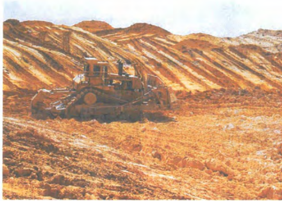
Bulldozer ripping and crushing limestone
