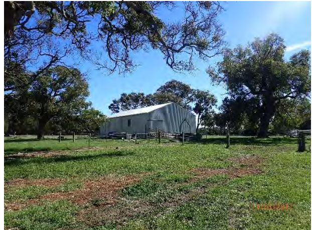
Photograph 4: View of shed infrastructure located on the adjacent property to the south east. Photo taken in 2017.
