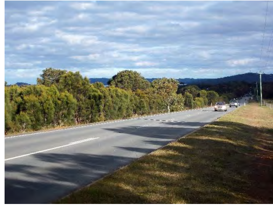
View of Lower King Road showing that a future intersection will have appropriate sight distances.
