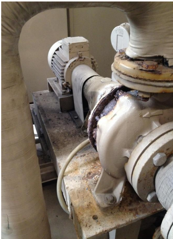
Figure 6 - Evaporator Pump
