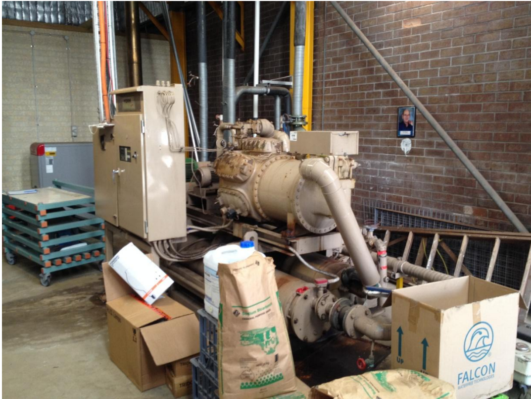
Figure 3 – Trane Heat Recovery Unit (Compressor Set)
