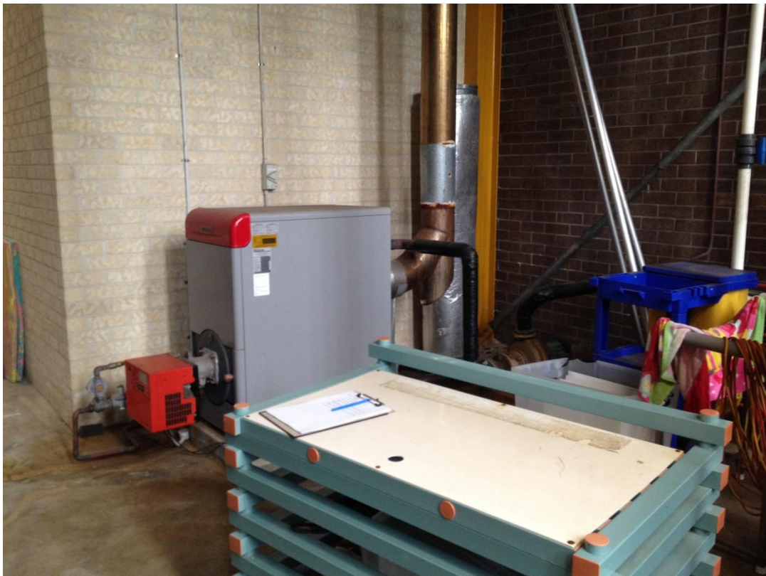
Figure 4 - LPG Boiler
