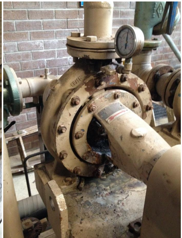
Figure 7 - Condenser Pump
