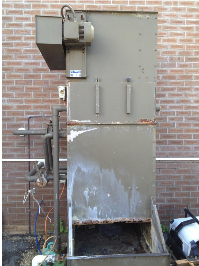
Figure 8 - Evaporative Condenser
