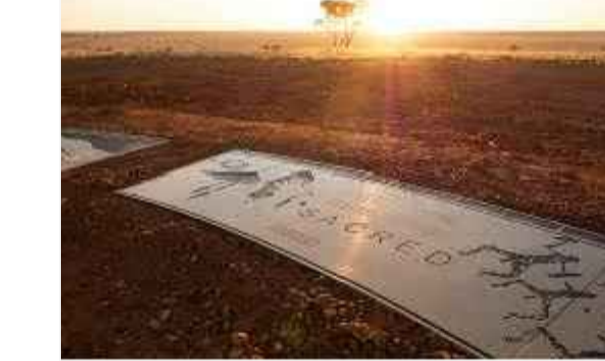
'DIRECTIVE SIGNAGE' IN NEW PATH WAY CAST IN LIME STONE COLOURED CONCRETE TO FORM DISTINGUISHED SECTION IN NEW LIME STONE WALK TRAIL (INDICATIVE LAYOUT)
