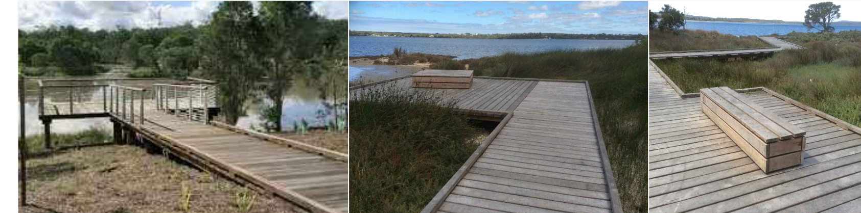
TIMBER DECKED VIEWING PLATFORM WITH TIMBER SEAT AND A TIMBER BOARD WALK FORMING THE TRANSITION TO NEW LIMESTONE PATHWAY
