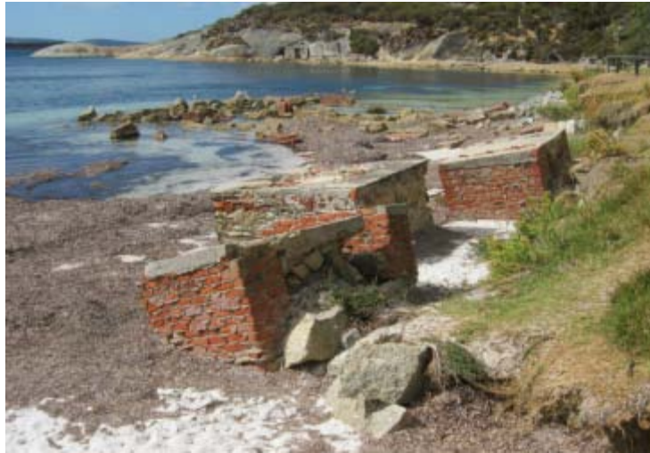
The debris in 2014
