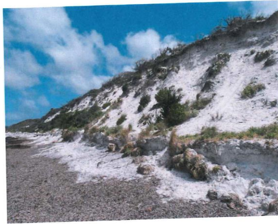
Photo 2. Recent ongoing erosion of both the older steep, high erosional scarp and the younger low erosional bench at the northern end of Goode Beach, as seen on 3 October 2017
