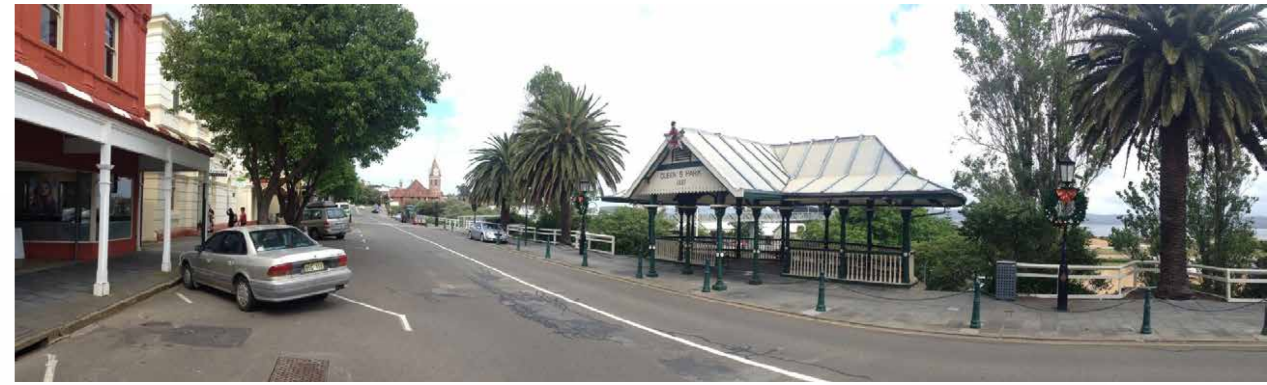
EXISTING CONDITION - LOOKING SOUTH EAST
