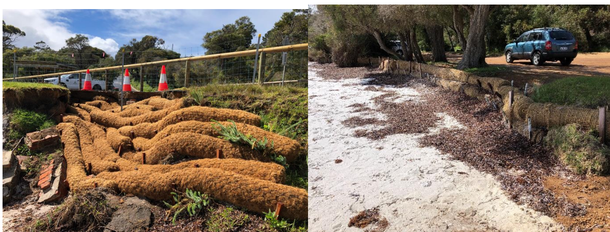
Figure 3.13 Coir Logs Installed by the City of Albany in 2021 to Combat Erosion
