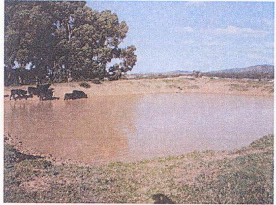
Plate 3: The artificial dam constructed on Lot 35.
