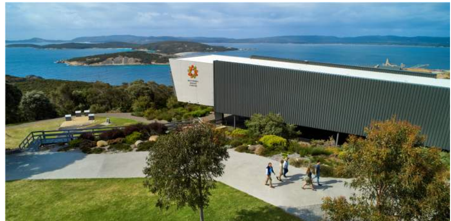
Wastewater treatment system at the National Anzac Centre Image: frances andrijich photography
