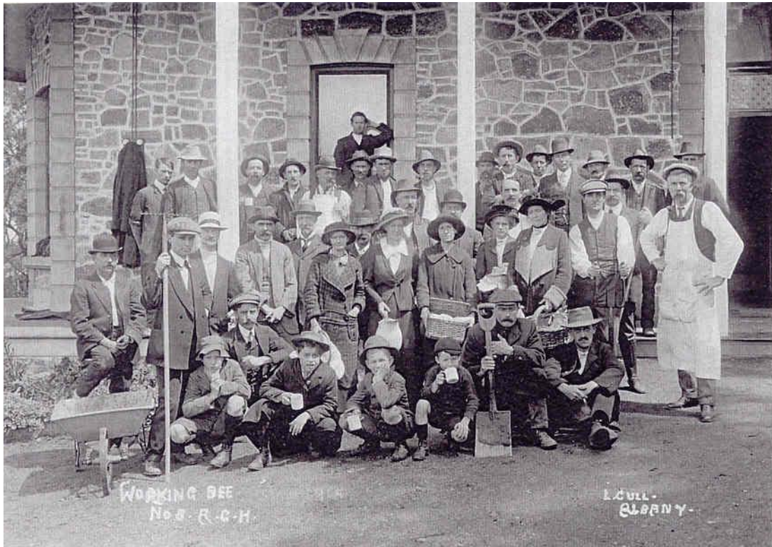
Photograph 36: Working bee at The Rocks Hostel 1915 (Courtesy of the City of Albany Local Studies Collection)
