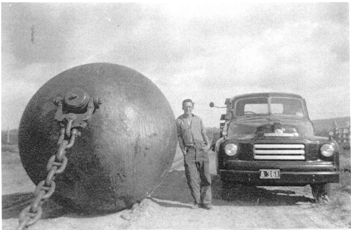
Photograph 38: Ball and Chain land clearing at Manypeaks 1950s (Courtesy of the City of Albany Local Studies Collection)
