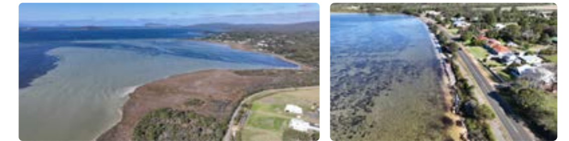
Areas associated with MU2 – unprotected assets close to coastal zone
