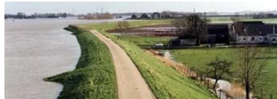
Earth levee example from the Netherlands (California Water Blog, 2015)
