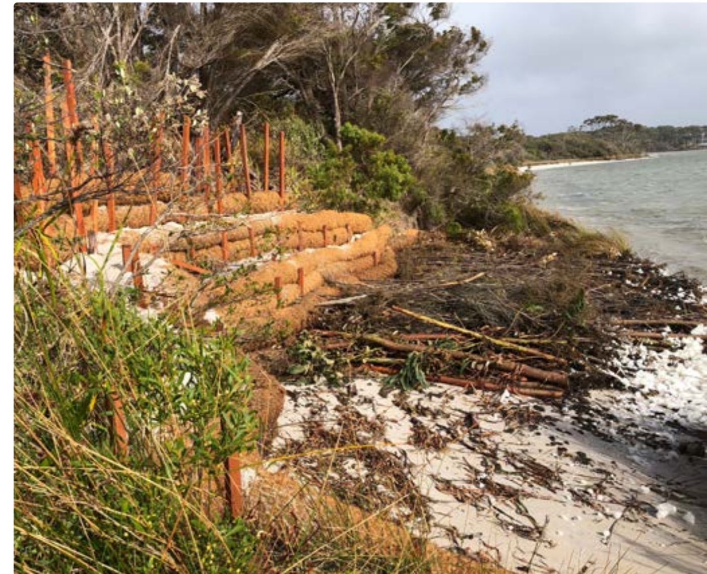
Erosion/protection - Princess Royal Harbour
