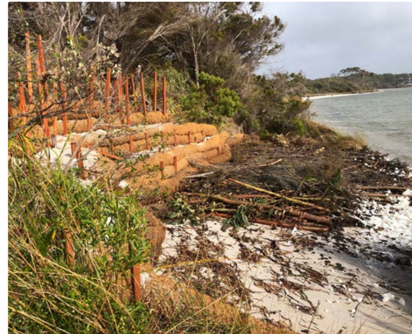
Erosion/protection - Princess Royal Harbour
