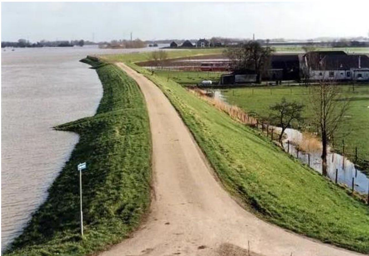
Figure 8-3 Earth levee example from the Netherlands (California Water Blog, 2015)
