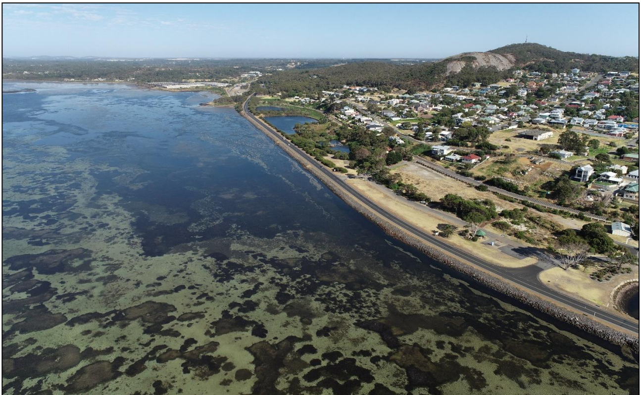
Figure 5-2 Hardened shoreline (seawall) between Point Frederick and Melville Point captured in January 2022 (image source: City of Albany, 2022)
