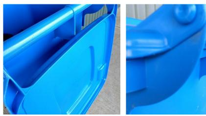
The centre rib on the original blue general waste bins, that prevent the bin lid slapping the body of the bin.
