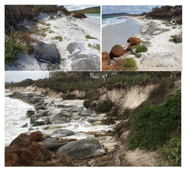
Figure 28: Erosion and state of the beach and GSC trial groynes and GSC revetment at Emu Beach, taken 26<sup>th</sup> February 2020 (top) and August 2020 (bottom).
