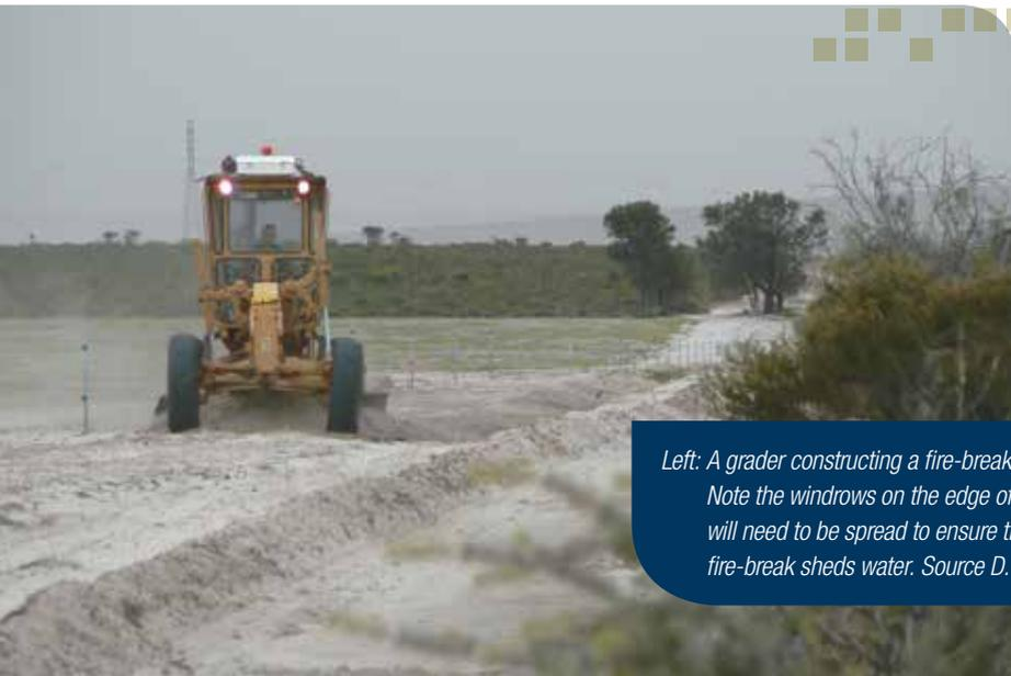
Left: A grader constructing a fire-break. Note the windrows on the edge of the break will need to be spread to ensure the fire-break sheds water. Source D. Atkins.
