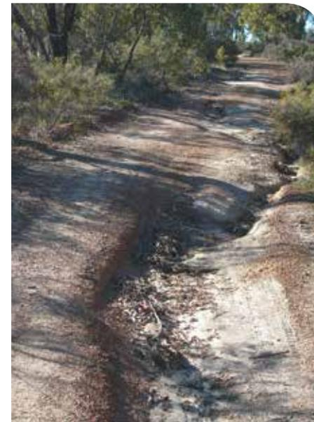
*Above: Water erosion on a fire-break without adequate erosion-prevention measures.*
